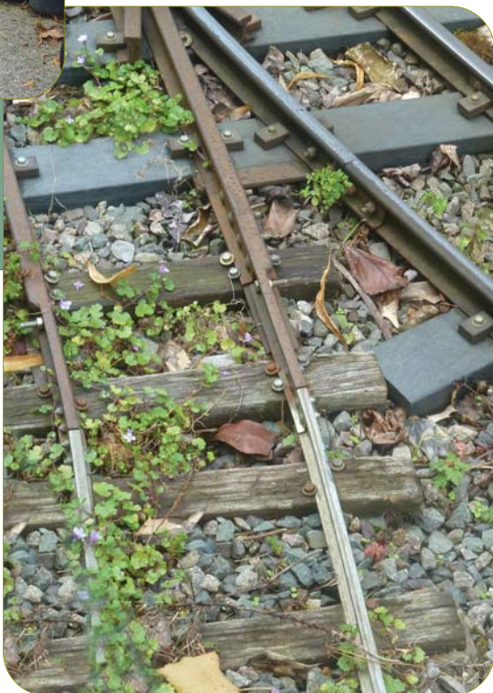
ABOVE: The old stock shed and lengthy disused tramway section from the mainline RIGHT: The whole railway was originally laid with 2lb/yd rail, and the siding to the old stock shed is one of the few stretches still in place. The junction with the newer 6lb rail is in the middle of the picture
