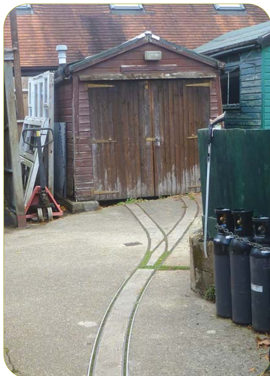
ABOVE: The old stock shed and lengthy disused tramway section from the mainline RIGHT: The whole railway was originally laid with 2lb/yd rail, and the siding to the old stock shed is one of the few stretches still in place. The junction with the newer 6lb rail is in the middle of the picture
