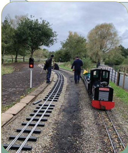
Relaying and ballasting at Moors Valley
