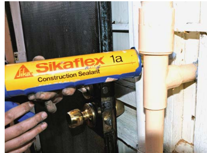
Exposed PVC pipe is painted to protect it from UV degradation. The hole is sealed with an adhesive sealant to prevent moisture from entering. Photo: David Glover.
