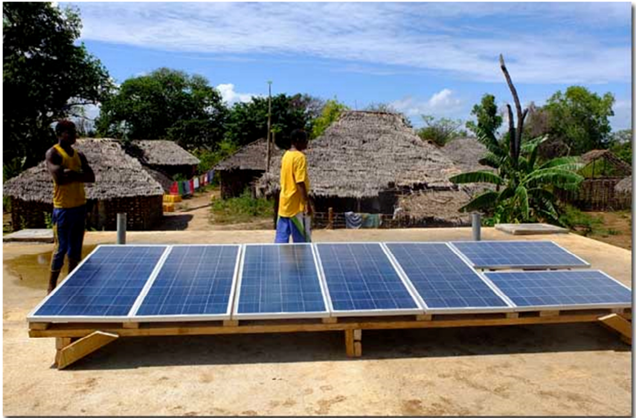
Harvesting the sun –Kokota’s portable microgrid is powered by a shared 700 W photovoltaic (PV) array. (Photo: Jeff Schnurr)
