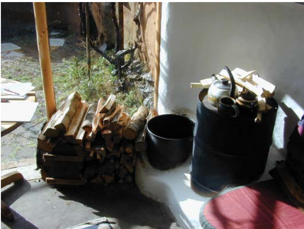
Above: The Rocket Mass Heater with bench at lower right in the home of Ianto Evans and Linda Smiley has been in use for over ten years. Dry firewood, split thin and cued up in the sun, small feed barrel and heat exchange barrel nestled in cob. Below: The continuation of the bench above. Note the thermometer about half-way up on the exposed vertical stack.
