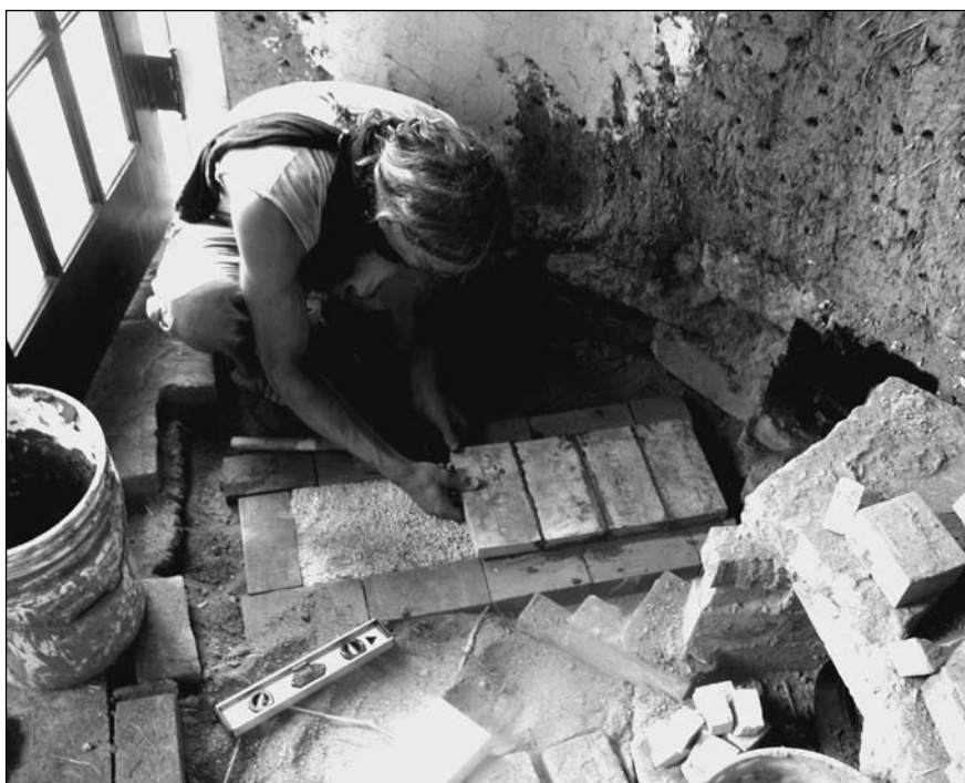
Chris laying the foundation for the stove. The burn tunnel of brick rests on a bed of perlite. Note Chris is building his first layer of brick and insulation sub-floor level. You can see the completed stove on page 84. Photos, this page, Christopher Reinhart.
