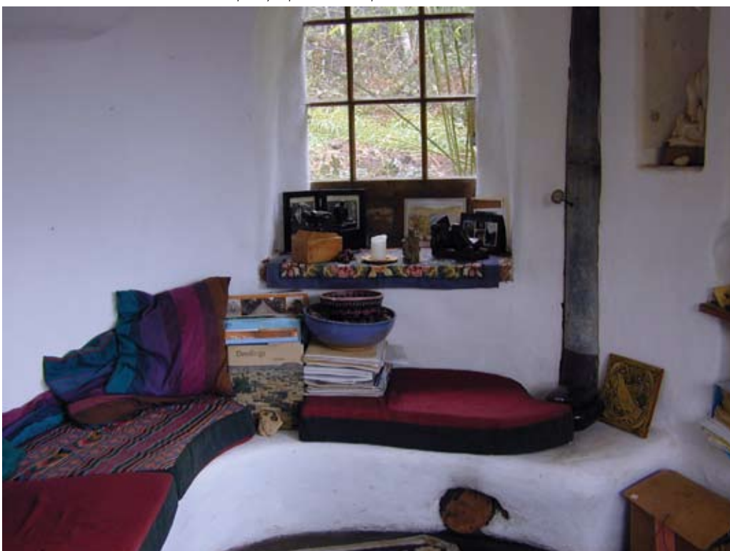
Above: The Rocket Mass Heater with bench at lower right in the home of Ianto Evans and Linda Smiley has been in use for over ten years. Dry firewood, split thin and cued up in the sun, small feed barrel and heat exchange barrel nestled in cob. Below: The continuation of the bench above. Note the thermometer about half-way up on the exposed vertical stack.
