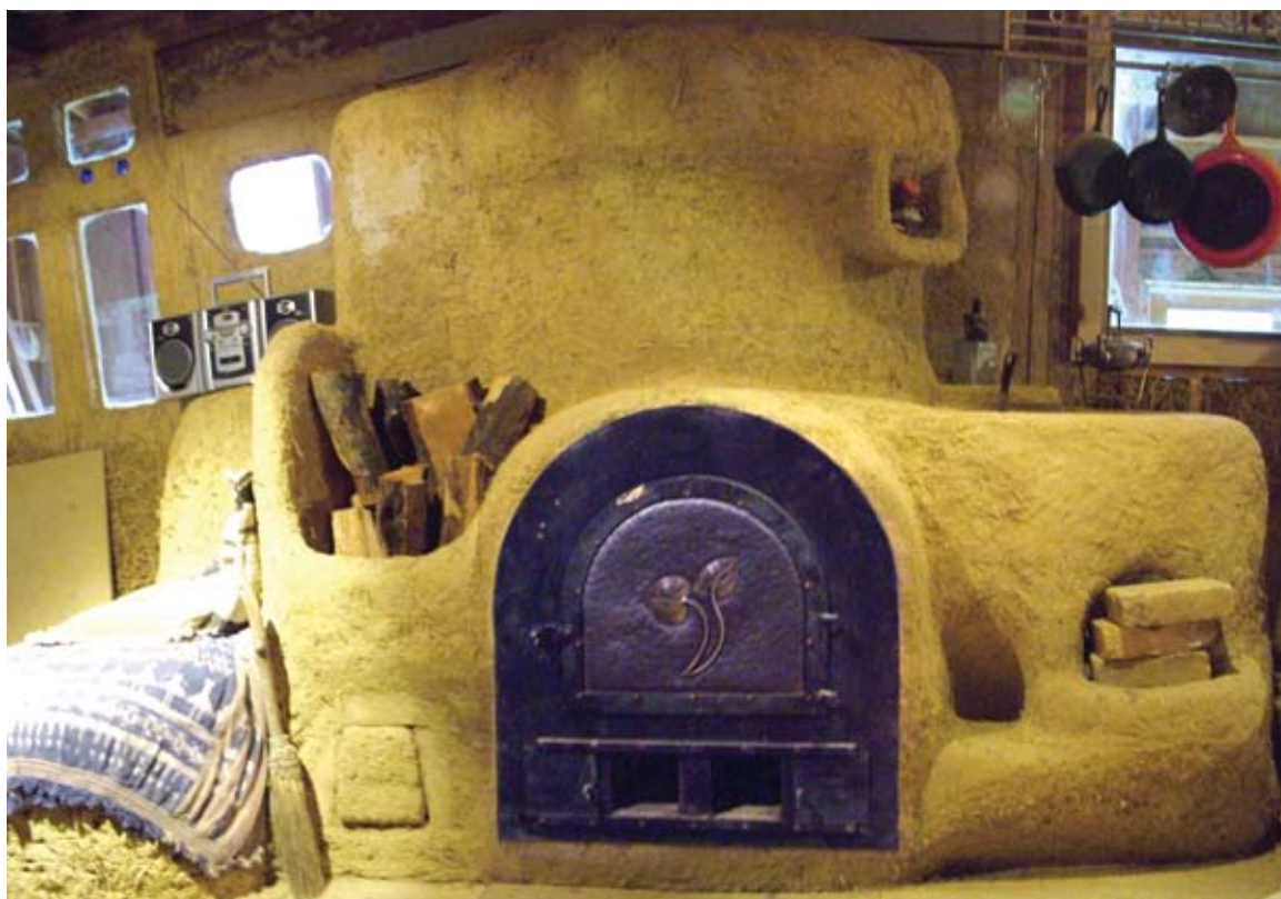
Above: Chris Reinhart's Rocket Stove. Note that the barrel is exposed quite a bit to maximize radiant heat. Below: Kirk Mobert's Rocket Stove with cooking surface on top. There are two cold air intakes below the metal door. The cob bench box keeps firewood dry.
