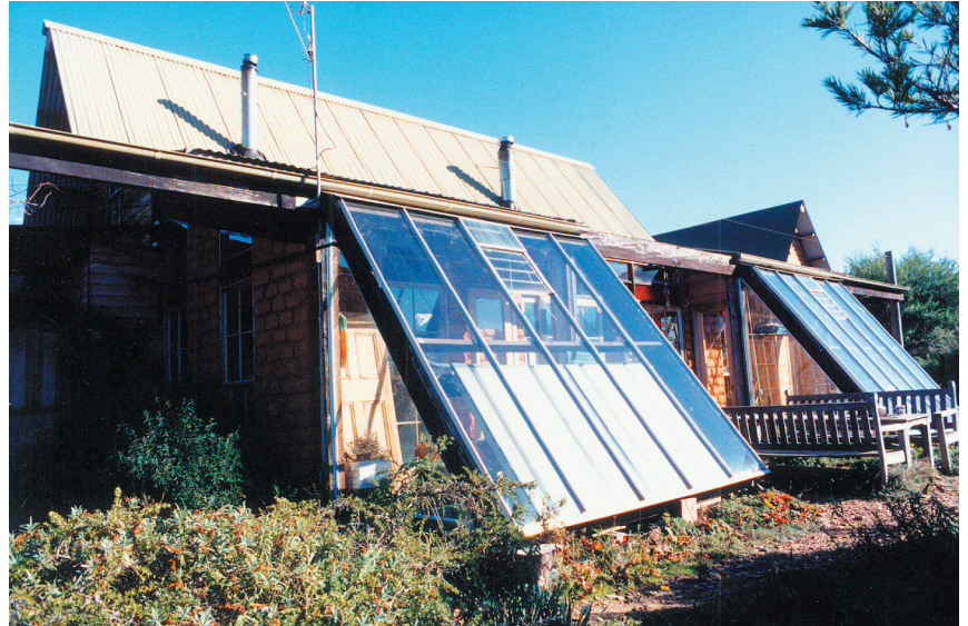
Cold climate solution — glasshouses face sunward on this mudbrick and timber house to warm the interior in winter. Heat is vented off in summer. A cosy sitting and dining nook was placed between glasshouses.
