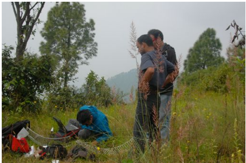
Figure CSD 5: Preparing for relay installation, Kumaon Network
