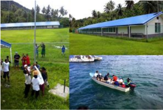
Figure CSP 4 : Mounting the pole mast in Udot
