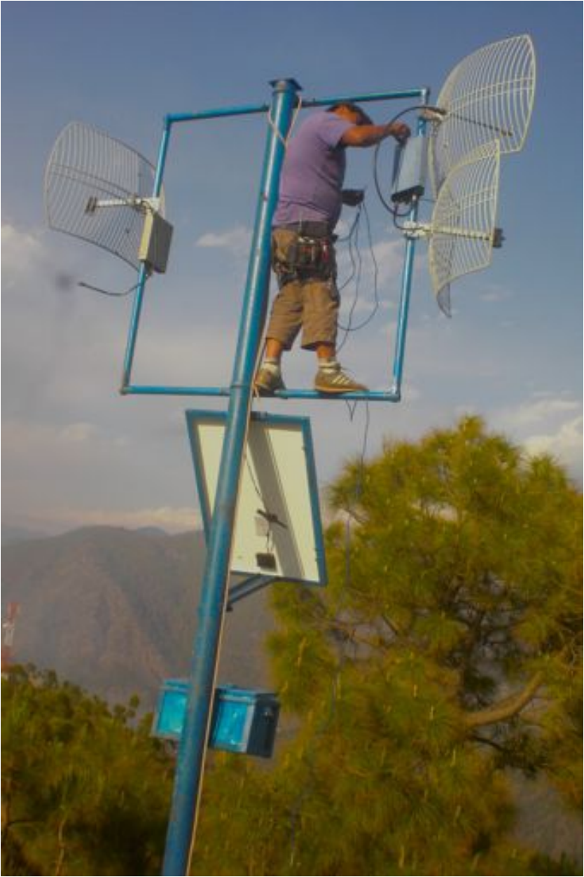
Figure CSD 8: Backhaul Relay, Garhwal Network
