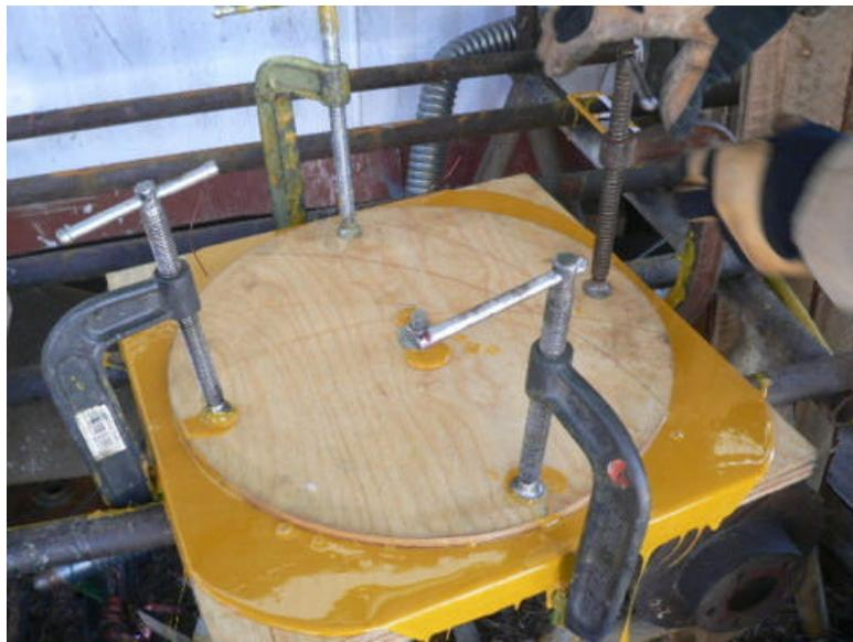
Put a C clamp on each side of the mold (use 4 C clamps) and tighten them evenly. You'll have some idea when the resin is hard by all the stuff that spilled out the side! Let the stator sit in the mold until the resin is hard.
