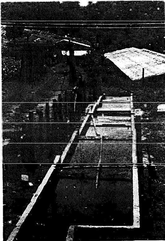
**Illustration 2-5: Sludge conditioning canals with overflow dams.**
