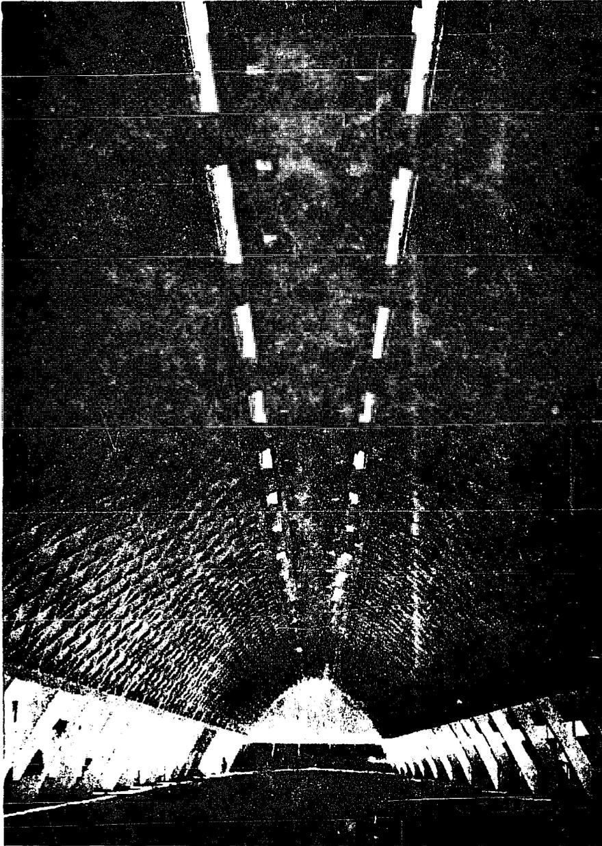
**FIGURE 8** Ferrocement-roofed warehouse in Tortona, Italy, for storing salt, designed and built by Nervi, 1950-51. Ferrocement has been used for high-priced domes and enormous roofs over stadiums, opera houses, restaurants, etc., but this specialized application is less relevant to the urgent needs of most developing countries. (Studio Nervi, Rome)
