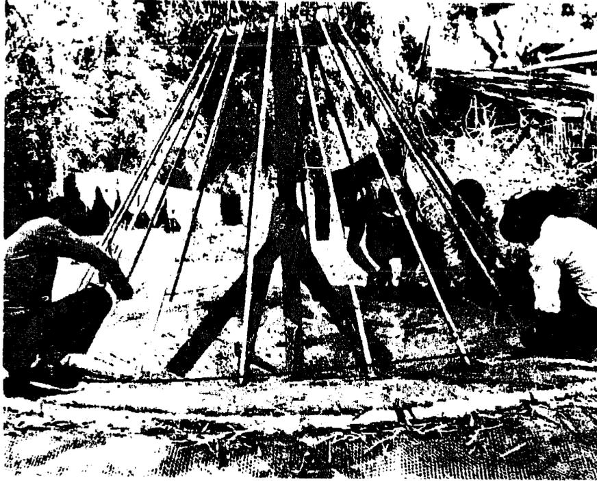
**FIGURE B-2** Ferrocement construction is straightforward, but labor-intensive: Construction of the walls begins after the base is complete. Mesh from base is integrated into the walls, which are strengthened with waterpipes or bamboo struts. Then horizontal hoops of reinforcing rod are wired to the struts. (Applied Scientific Research Corporation of Thailand)
