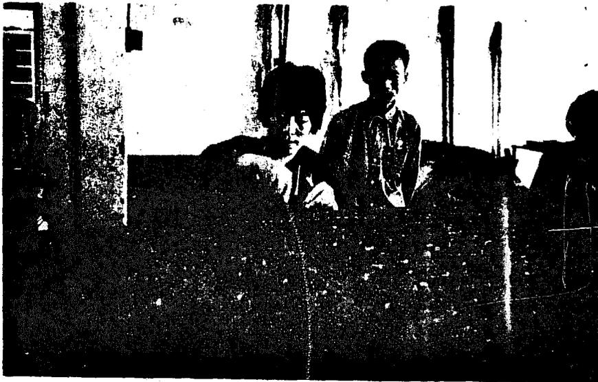
FIGURE A-6 Worker ties together layers of mesh and rods by threading short lengths of wire through and pulling them back with a small hooked tool. Although the construction uses unskilled labor, a supervisor maintains quality control.
