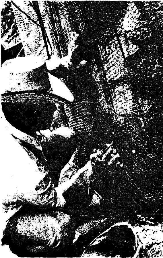
FIGURE 9 A paste of mortar is forced into the layers of mesh by hand . . . (Smith Kam-pempool, Applied Scientific Research Corporation of Thailand)
