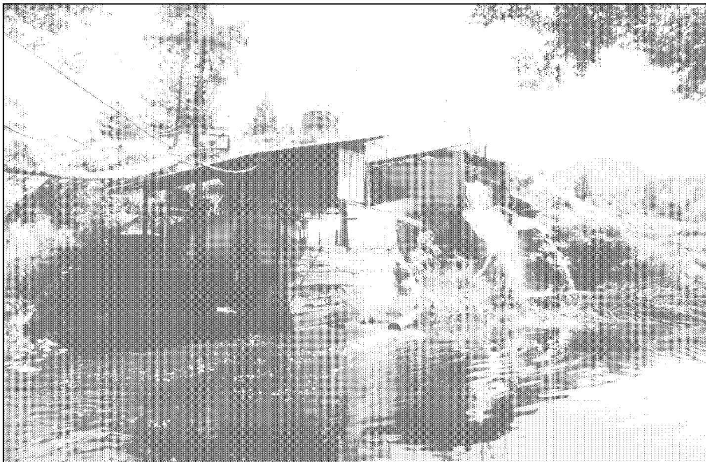
Above: Stuart Higgs' hydroelectric turbine generates power for two all-electric homes. On the left is the powerhouse holding the 30,000 watt alternator. To the right, overflow water spills from the fish guard. The day this photo was taken the turbine was producing 12 kw. (288 kwh/day) while cycling 770 pounds of water per second. Photo by Richard Perez
