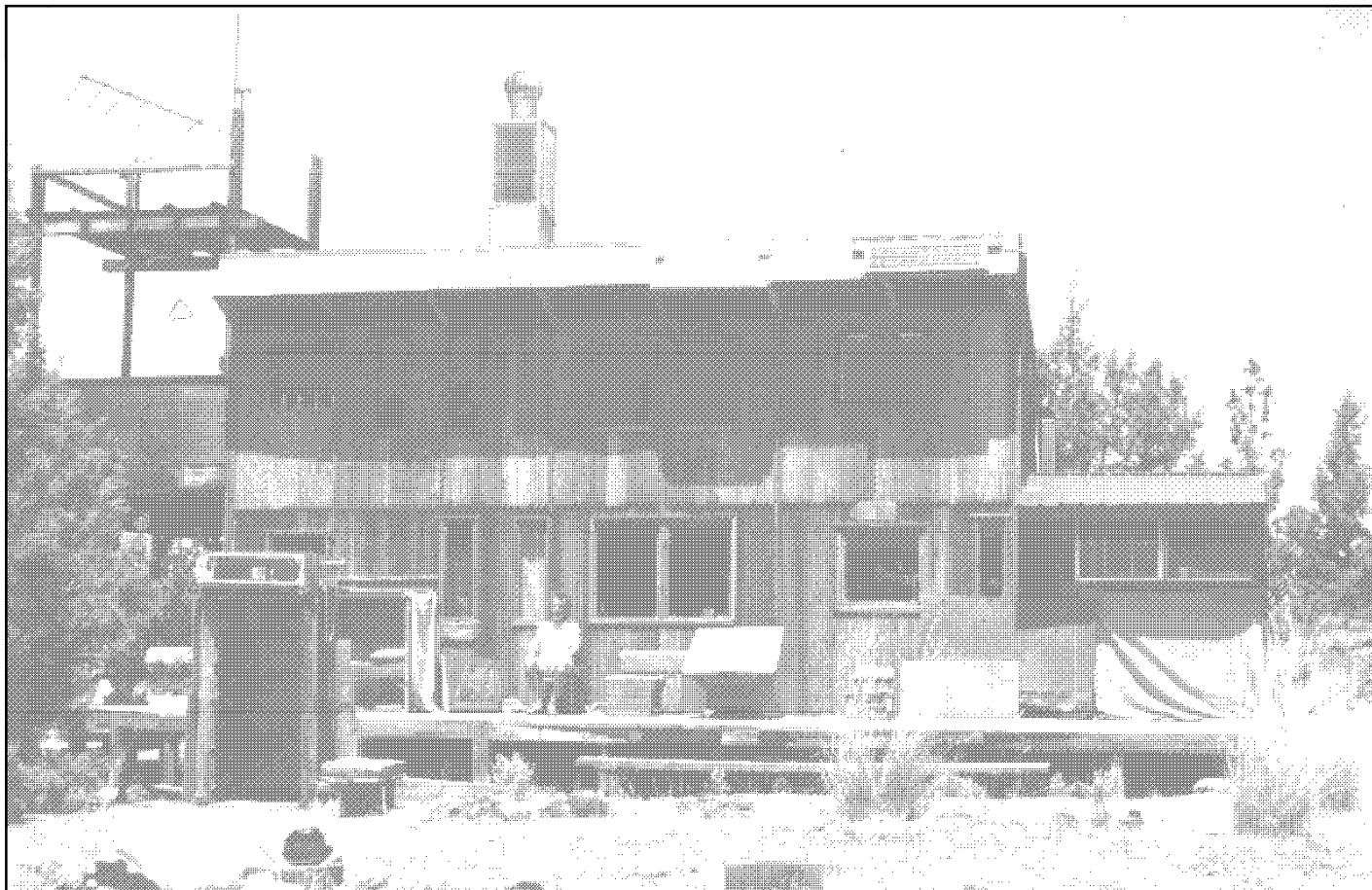
Above: Stu Ward's solar-powered and owner-built home in northern California. Two solar electric panels provide the power, a solar oven does the cooking, and passive solar architecture keeps the home warm. Photo by Kathleen Jarschke-Schultze
