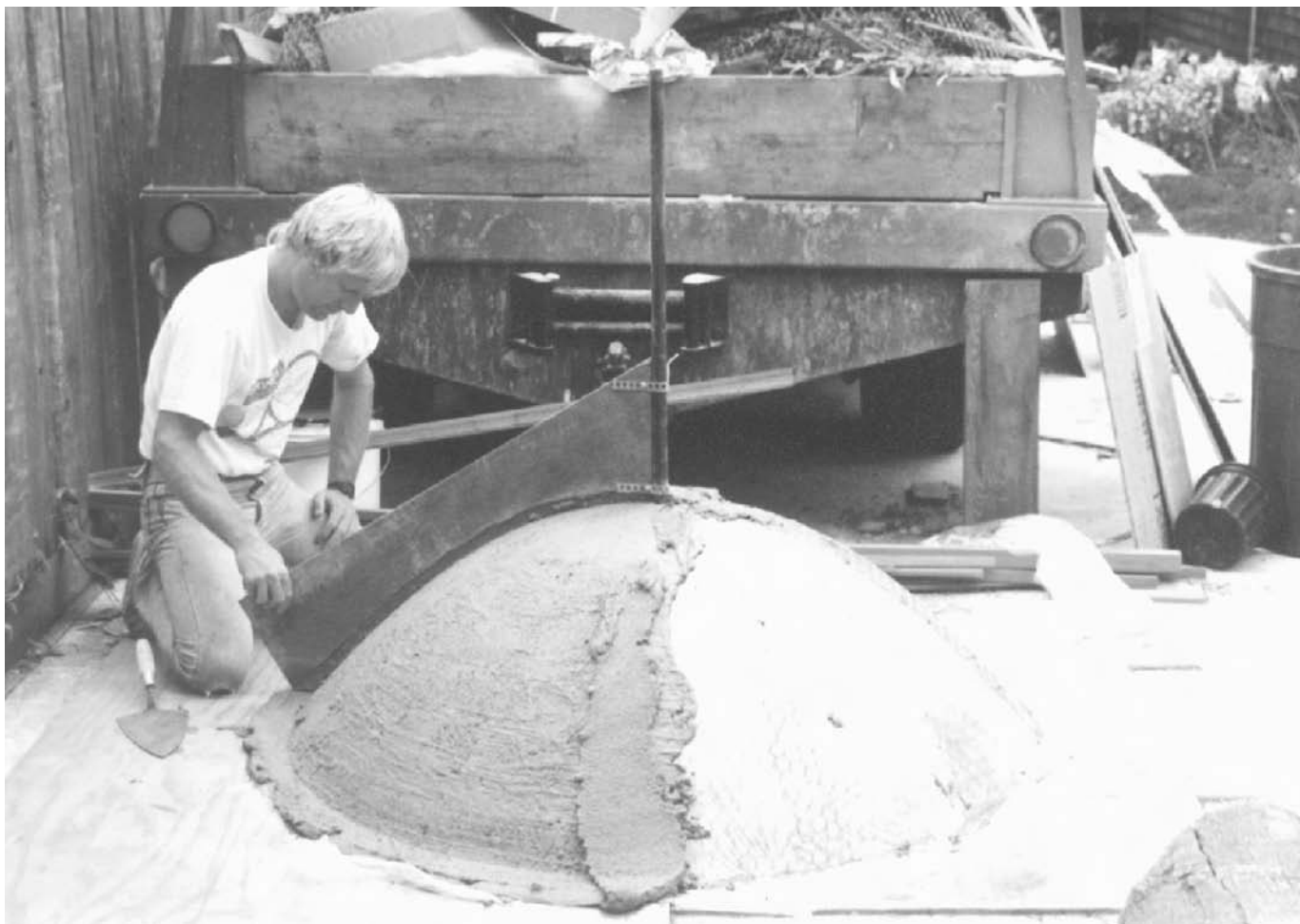
Above: After the form is done, Cody Brewer constructs a parabolic cooker.
