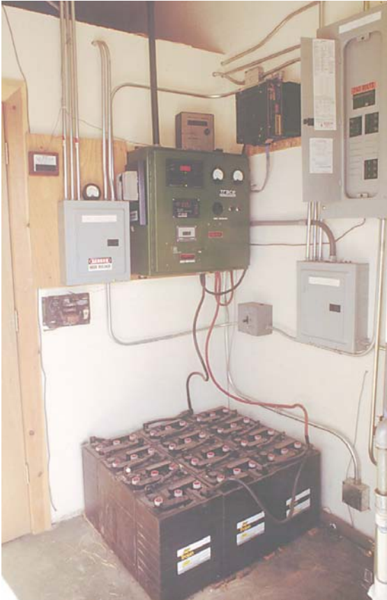
Above Left: The batteries and energy processing equipment.
