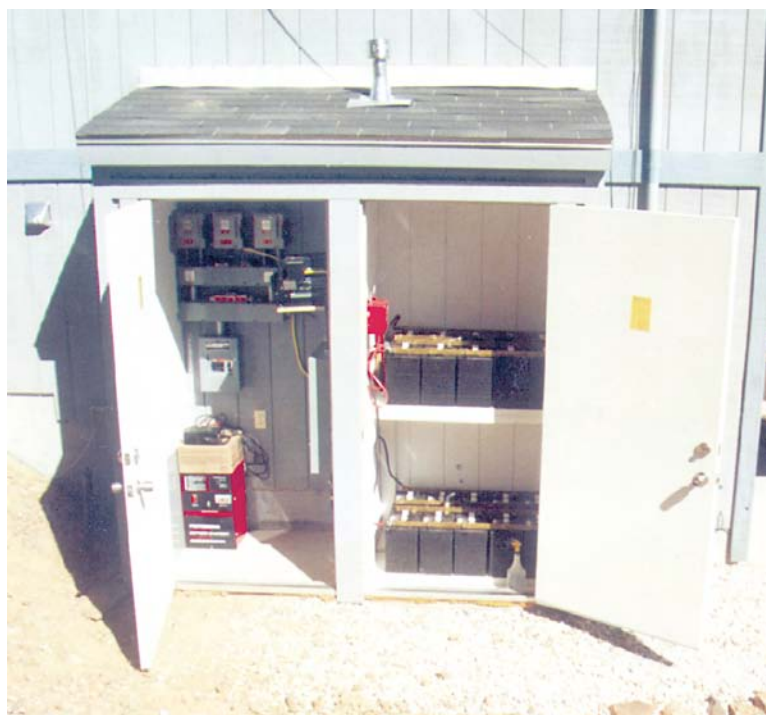
Above: The power/battery room. The inverters are safely sequestered from the battery in their own room.
