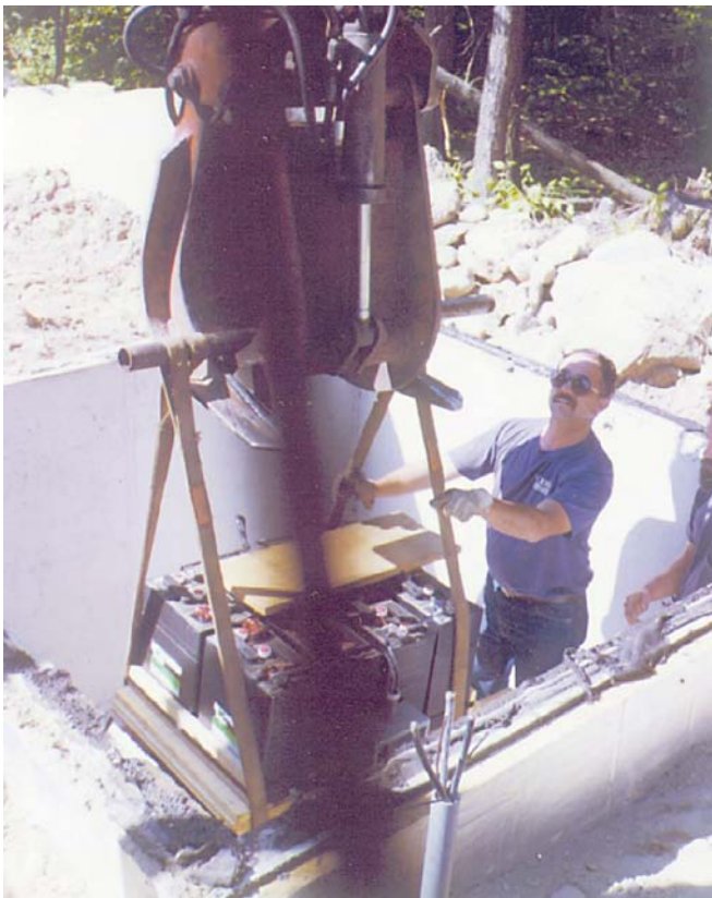
Above: Jean guides the batteries safely into their new underground home.
