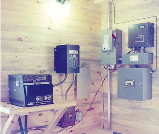
Above Left: The interior of the power shed with inverter, controls, instruments, and safety disconnects. Above Right: An exterior photo of the completed power shed with eight PV modules on its roof. The batteries are housed underground to keep them warm during the winter.
