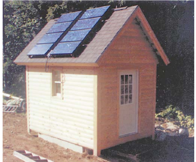
Above Left: The interior of the power shed with inverter, controls, instruments, and safety disconnects. Above Right: An exterior photo of the completed power shed with eight PV modules on its roof. The batteries are housed underground to keep them warm during the winter.
