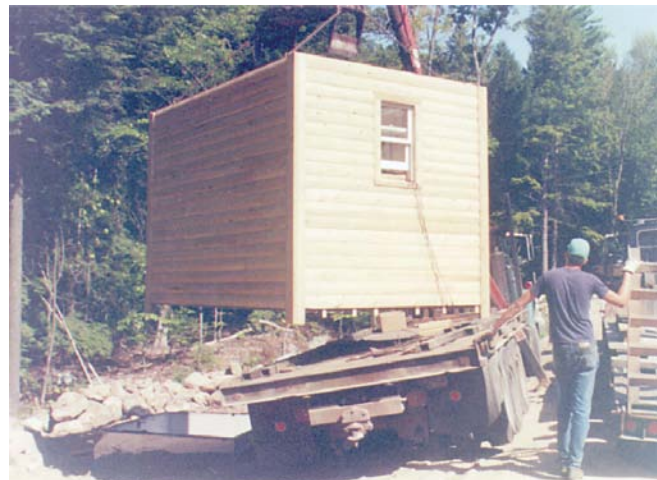
Above: A boom truck lowers the completed power shed onto its foundation.
