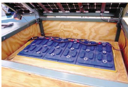
Above left, center and right: Steve Fox of Wyoming, Michigan demonstrates his portable PV power system. This system on a trailer uses eight modules, a 1000 Amp-hr. battery and an Exeltech sine wave inverter. Steve powered seven solid hours of live electric music with this system last Earth Day. The workmanship is first class!
