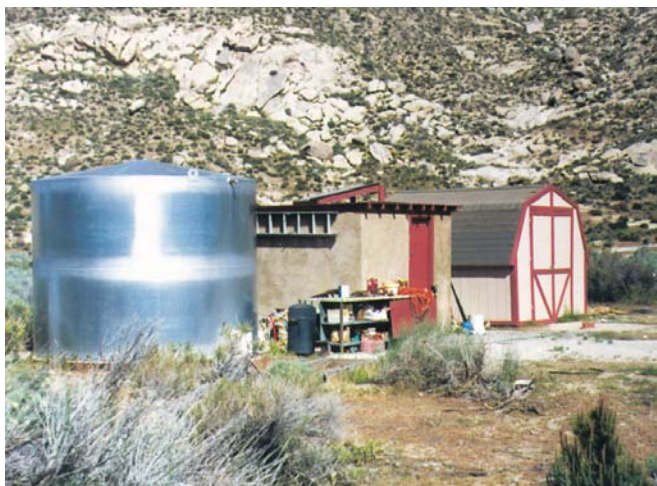
Above: The pump house with PV modules on its roof, and the water storage tank.
