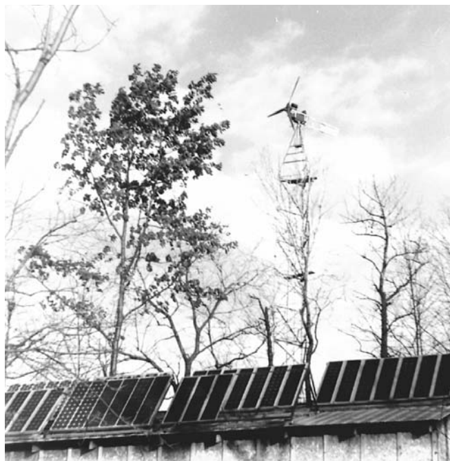
Above: The 1.5 kW. wind generator on a hill behind our barn's PV covered roof. Photo by Dick Linn
