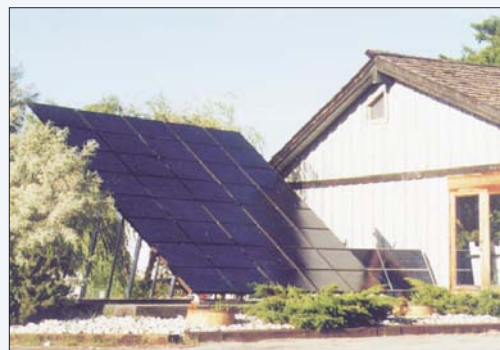
Our shop utilizes its own 2.5 kw array and 35 kw battery bank for daily power needs and testing of new products.
