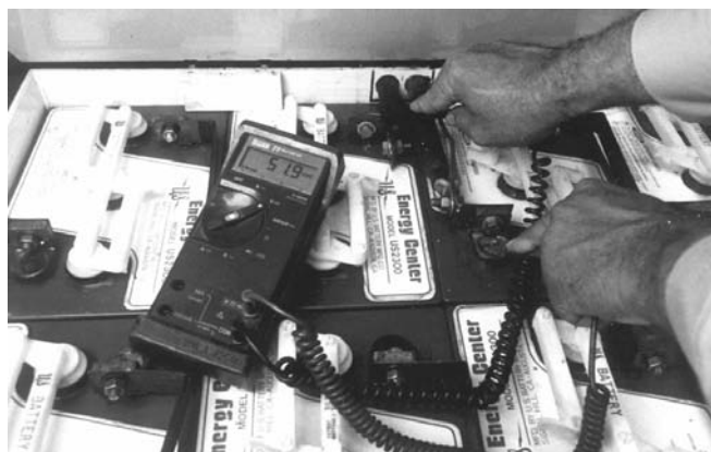
Above: Testing each battery pack for full voltage separately, before connecting them.
