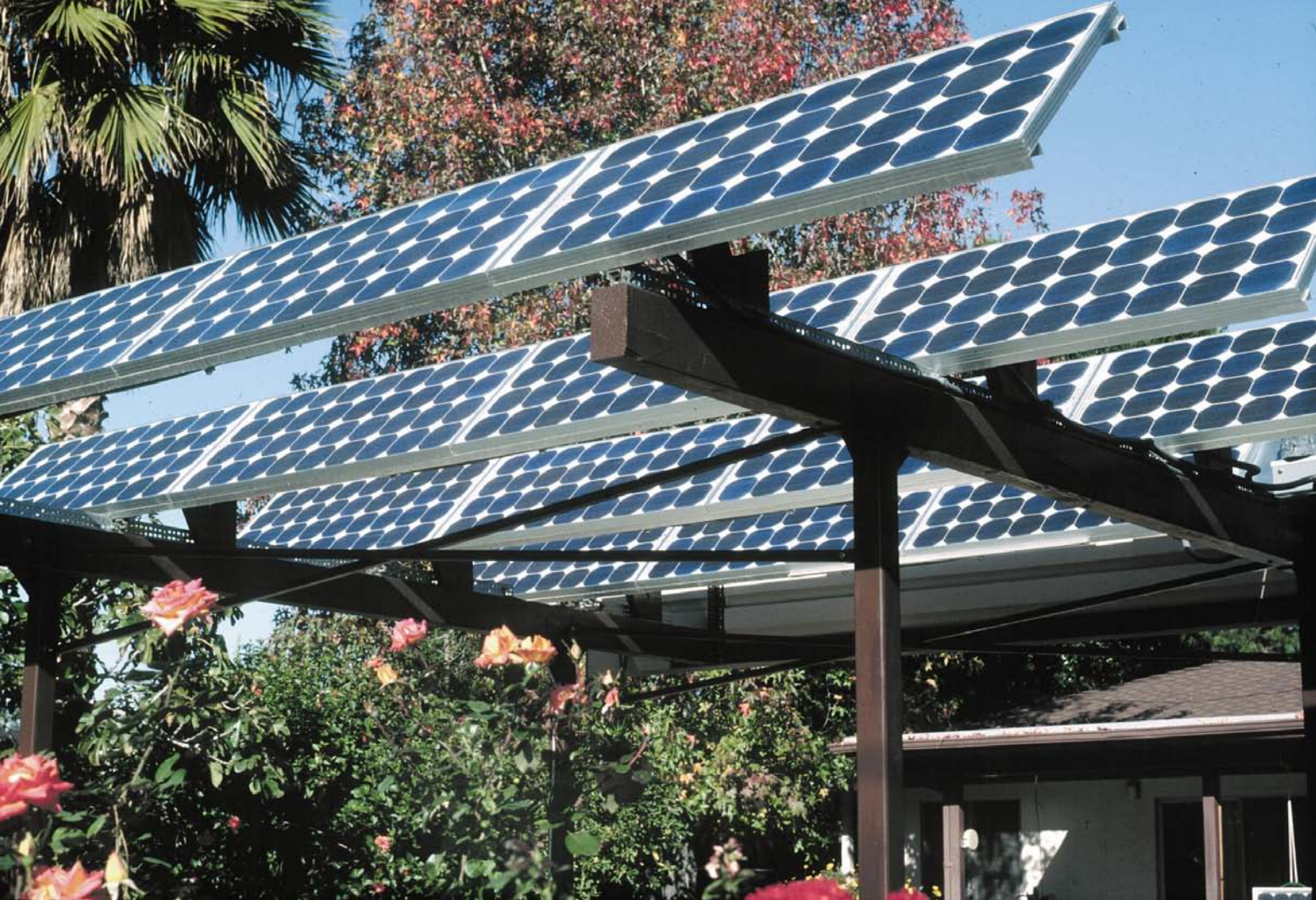
Above: Fifteen photovoltaic modules provide power to Robert Siebert's grid-connected California home.
