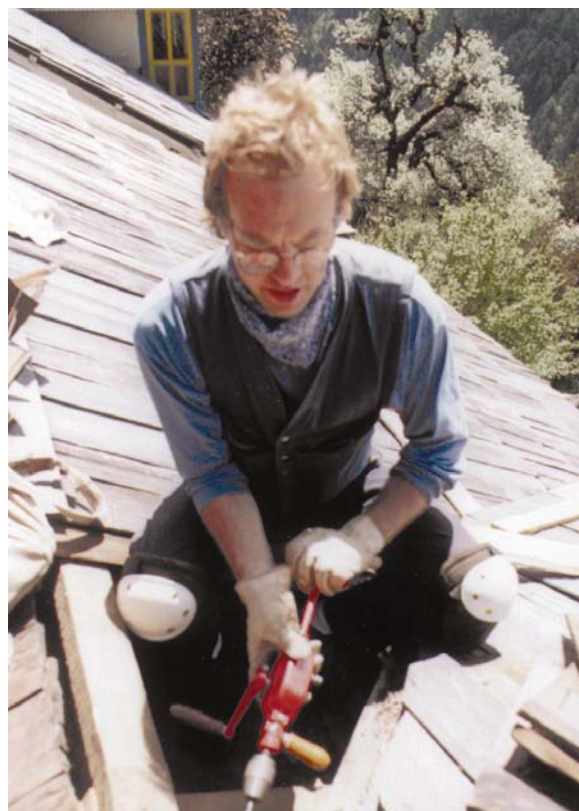
Below: Dennis drilled holes to run the wiring from the roof to the rooms below.
