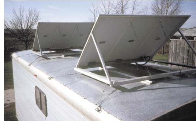
Above: A view of the PV laminates from behind, showing their mounting structures.
