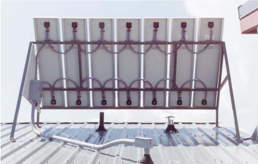
Above: the back of the PV array showing the wiring and mounting rack.
