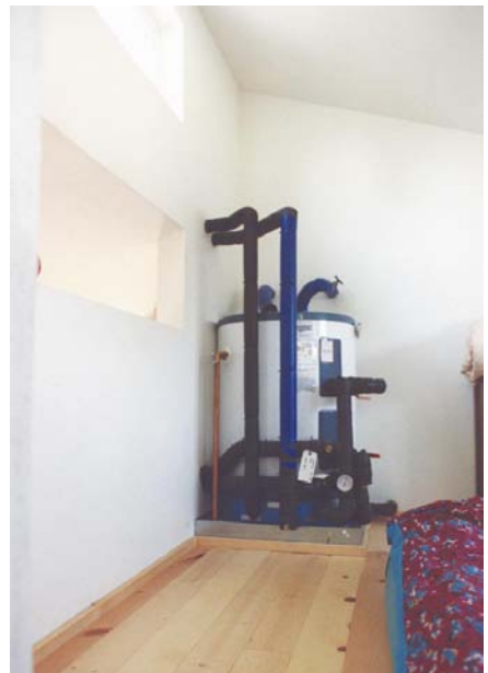
Above: the hot water tank with solar loop.
