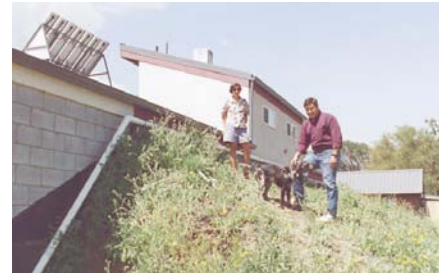
Above: the earthbermed north wall
