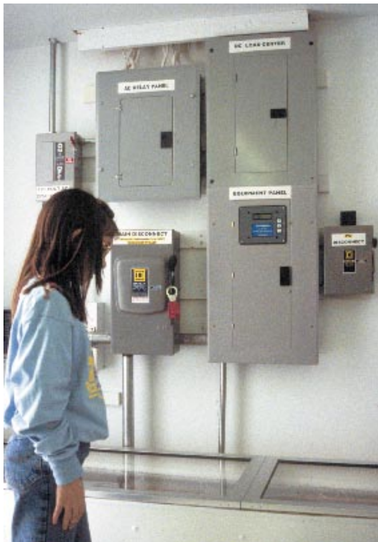
Above: The power center with the plexiglass-covered, battery box below
