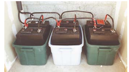
Above: the batteries in tubs
