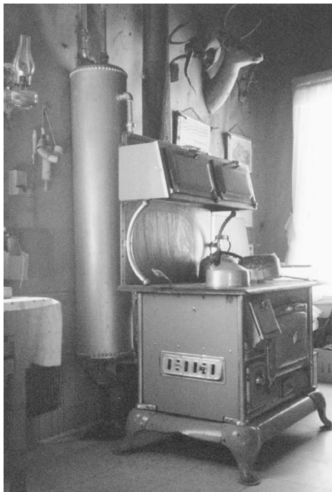
Above: This water-back/range boiler has been working since the early 1920s.
