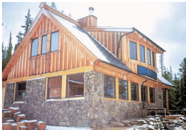
Above: The Traditional style of Uncle Bud's Hut integrates perfectly with the natural beauty of the Rocky Mountains. Notice the winter oriented (vertical) array before its replacement with an all-season pole mount system.
