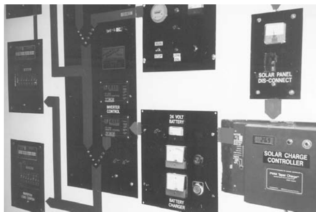
Above: Transfer Switch and Controls: The use of graphics and LED lights makes it easy to spot any electrical problems
