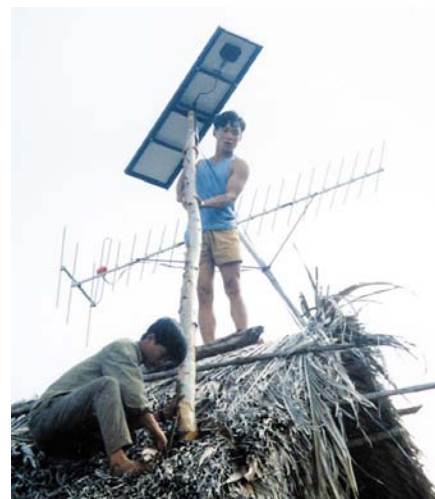
Above: Mounting the panel on a thatched roof, Hoa Minh Commune.
