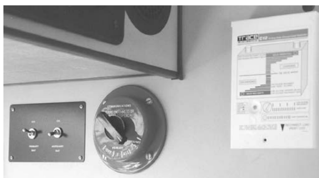
Above (left to right): coach load switches, transmitter switch, C-12 charge controller—all wiring is behind the closet wall shown here.
