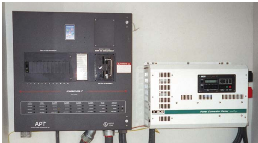
Above: The Ananda Powercenter 5 and the Trace SW4024 are mounted in a separate room from the batteries.
