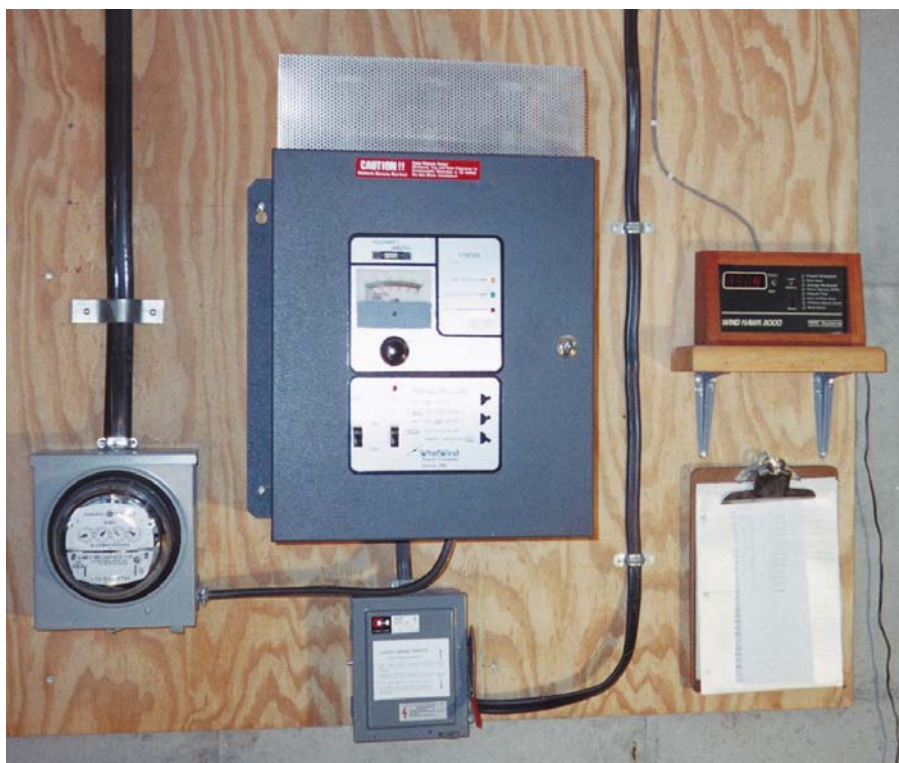
Above: Output Meter, synchronous inverter, safety brake switch, and Wind Hawk 8000 are located inside the house.
