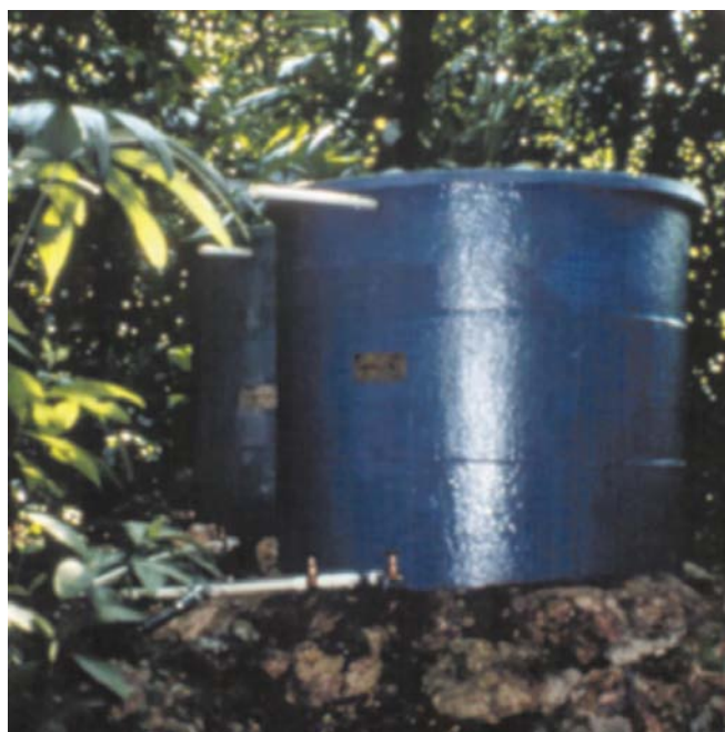
Above: Two 600 gallon water tanks sit 60 feet above the clinic and provide gravity pressure.
