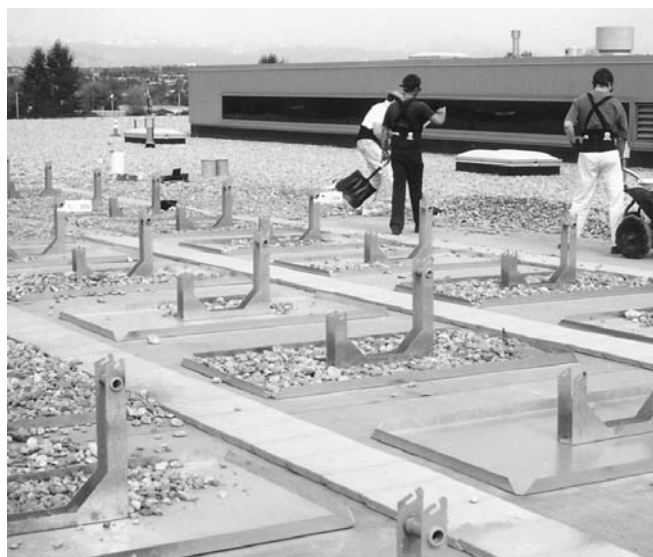
Above: Gravel holds roof jacks to roof.
