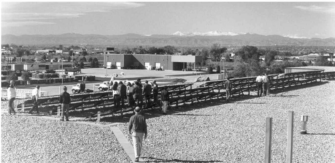
Above: The roof mounted ninety panel, 18 kW array.
