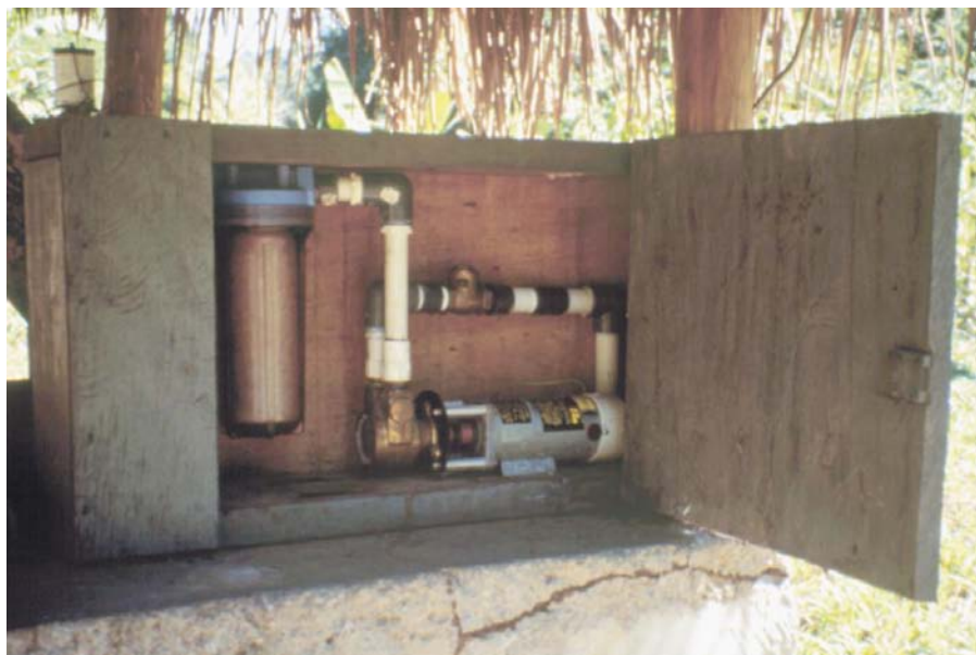
Above: Pump box containing Slowpump™, in-line filter, and Linear Current Booster™ supplies water from a spring. See the pump house on the cover.
