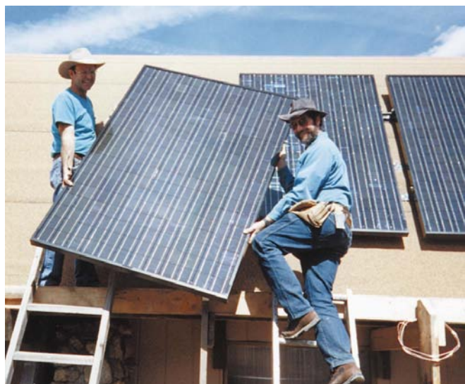
Above: Robert Warren and Don Waggoner heft a 4 by 6 foot, 245 Watt panel into place.
