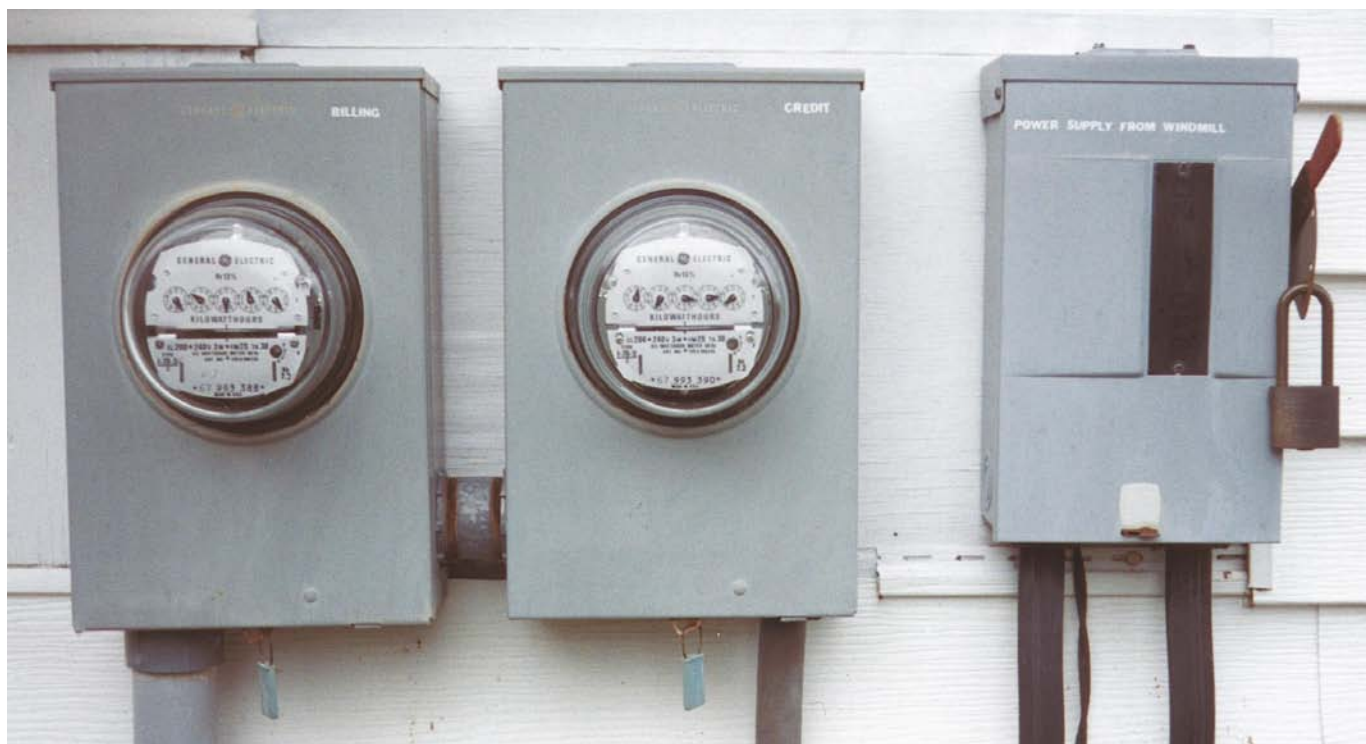
Above: The billing meter, credit meter, and lockable shutoff are located outside the house.
