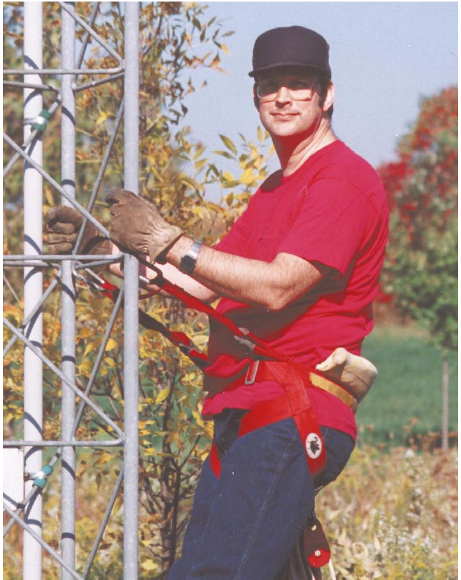
Above: Carl Berger clips in with a safety harness before beginning the 120 foot climb to the top of his tower.
