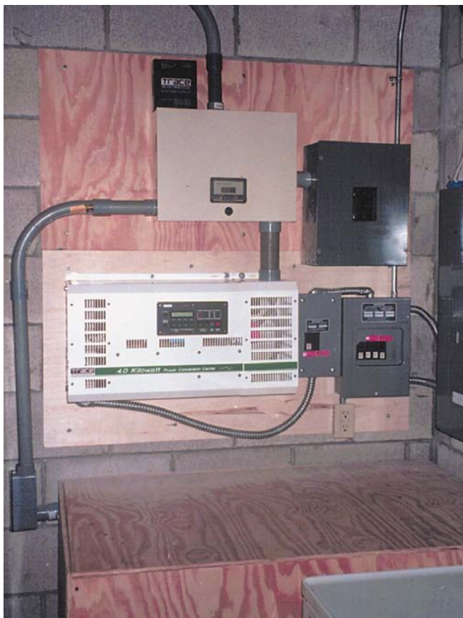
Above: The battery box and control center including a Trace SW-4024, C-30A, and Cruising AH+2 meter.
