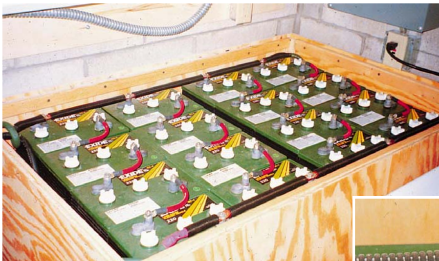
Left: Sixteen of the twenty-eight Exide GC-4 batteries. 1540 Ampere-hours at 24 Volts DC.
