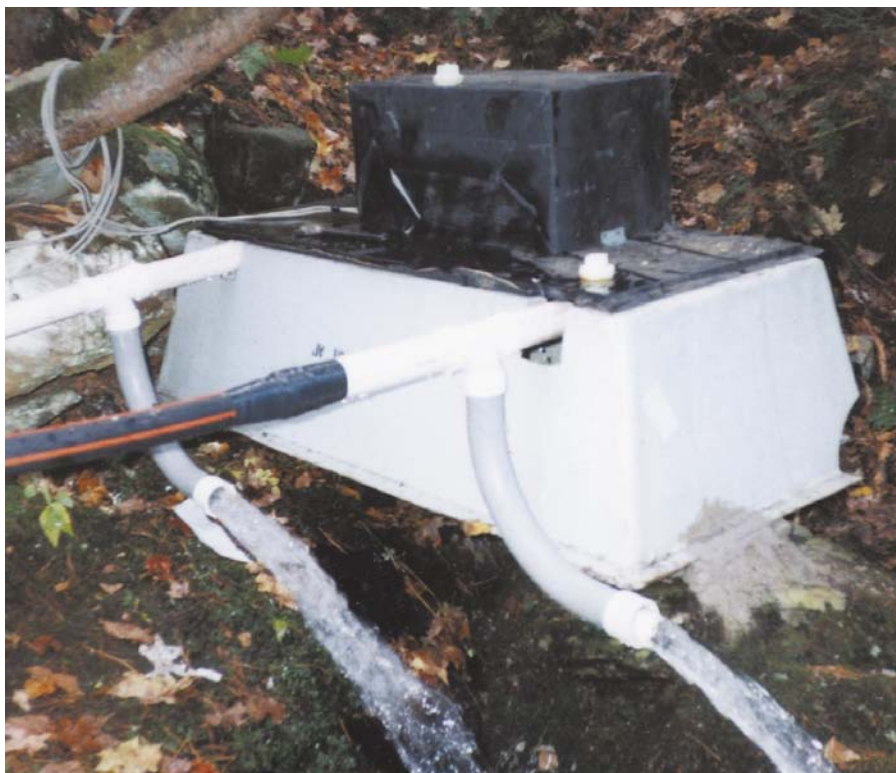
Below: The completed hydro plant showing the two diverters used when the cabin is unoccupied.
