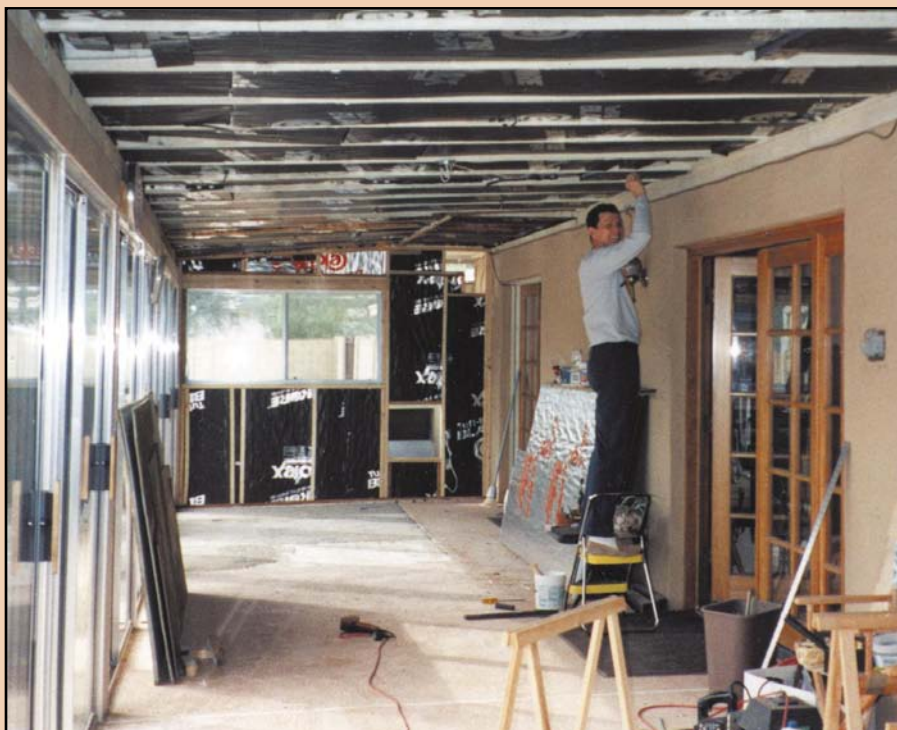
Above: Harold finishes the installation of foam board insulation on the ceiling
