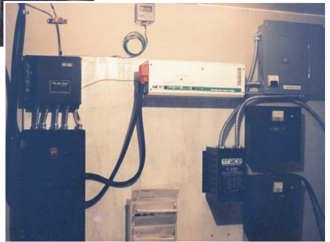
Below: The control board for the photovoltaic system. Notice the rack that keeps documentation for the components organized and handy.
