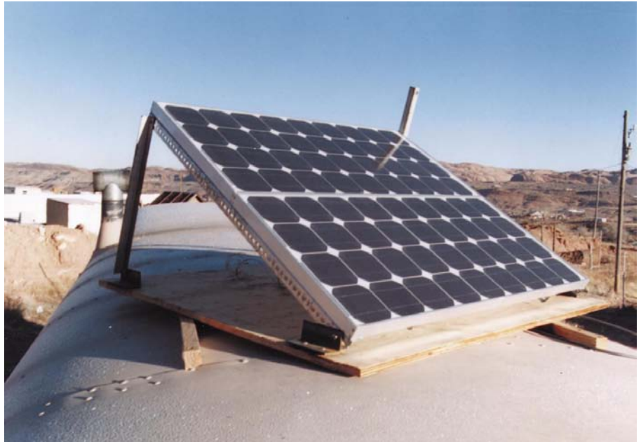
Above: Two Solavolt PV modules tilt and rotate on a homemade frame mounted on the roof of Rob's bus
