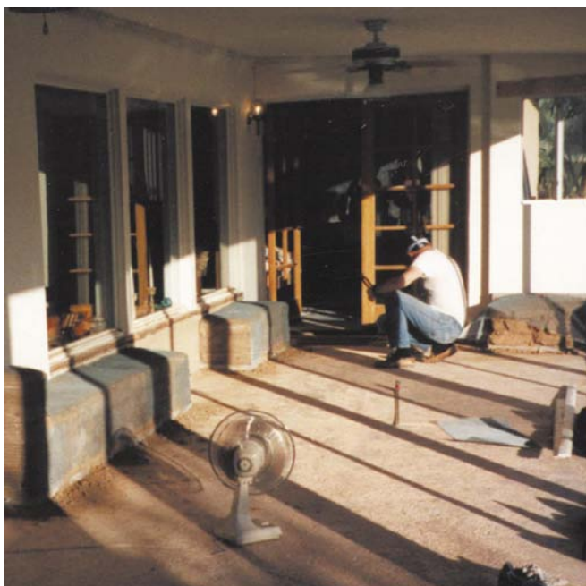
Below: Covering the adobe bancos with expanded metal prior to the application of the stucco.
