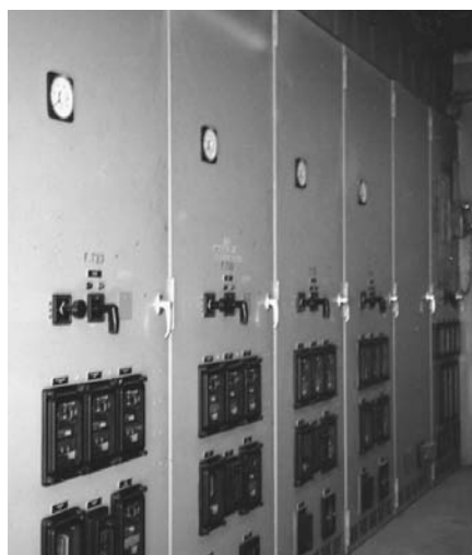
Picture 2, Left: An enclosed metal clad 13kv distribution switch gear. Each of the doors has a 3 phase circuit breaker behind it. On the door are protection relaying and an ammeter for reading each phase current.
