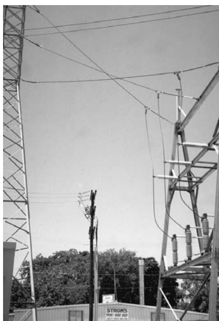
Picture 1, Above: On the left a 138 kv highline tower with conductors going to the right to a substation "A" frame dead-end. On the dead end are 138kv disconnect switches in the closed position. In the middle of the picture is a wood pole with an underground riser 3 phase pothead (that's what they call them) going through switches and attaching to a 3 phase 13kv distribution circuit. These circuits would come from a feeder breaker in the switch gear.
