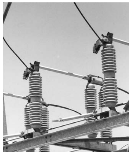
Picture 3, Right: 3 phase 138kv disconnect switches as mentioned in picture #1. These switches are in the closed position. If the switches were open (they all open together) then the horizontal long tubes between the vertical insulators would be pointed up from the back of the switch (where the wires go down).
