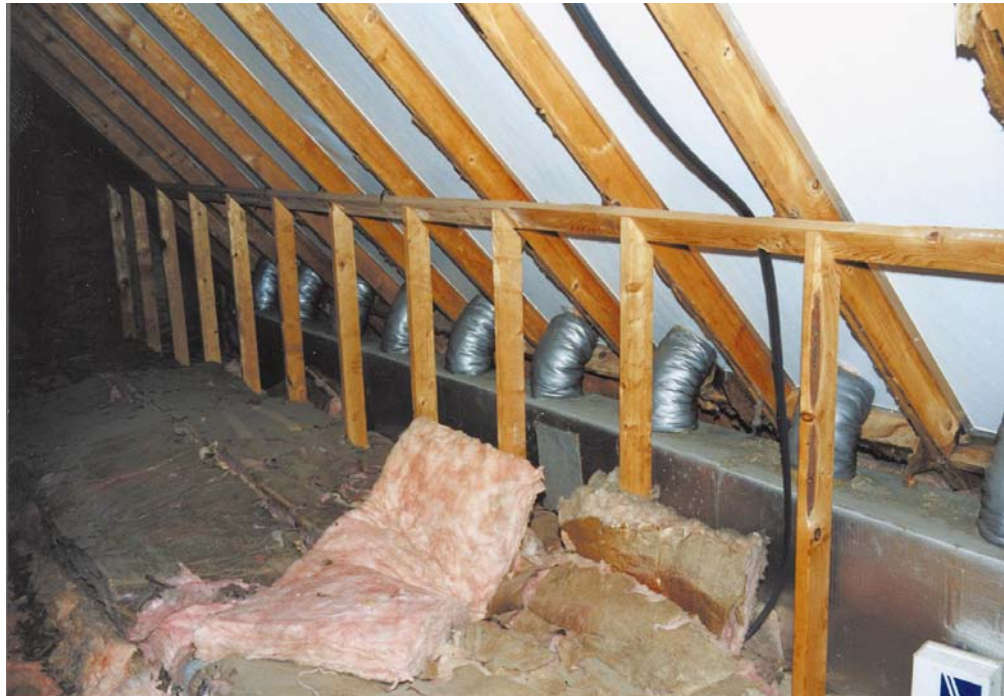
Above: The attic where cool air enters the hot air collectors.
