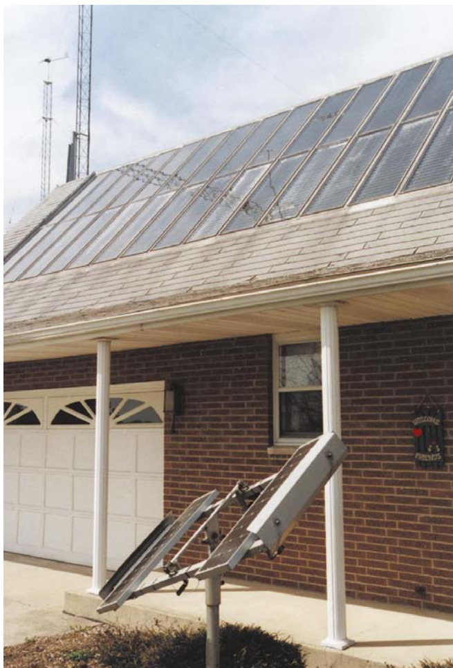
Above: Walt's front walk showing solar thermal panels on the roof and the photovoltaic array powering his HAM radio system.
