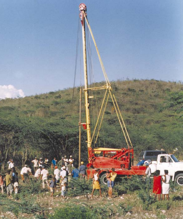
Above: Drilling for water at the initial (unsuccessful) well site. A second location provided more than enough water for the 546 residents.
