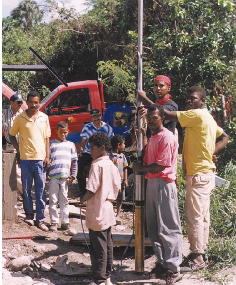
Above: The A.Y. McDonald pump assembled and ready for installation into the 35 foot deep well casing.
