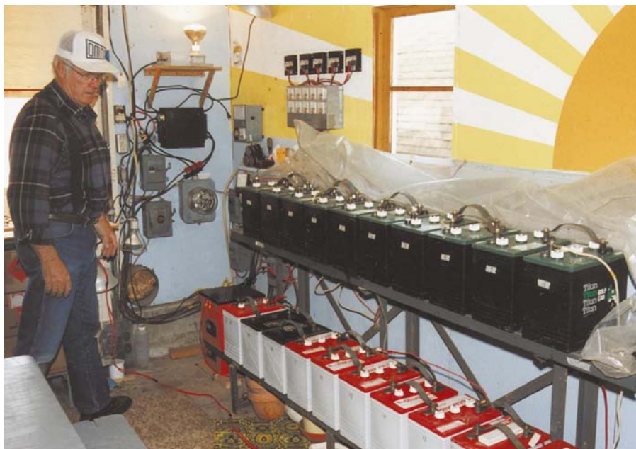
Above: Walt explains the single series string of twenty 6 Volt golf cart batteries which provide 220 Ampere-hours of storage.
