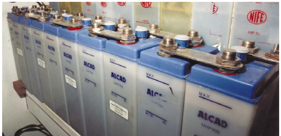
Below: The R/T's independant 12 Volt Nickel Cadmium battery bank
