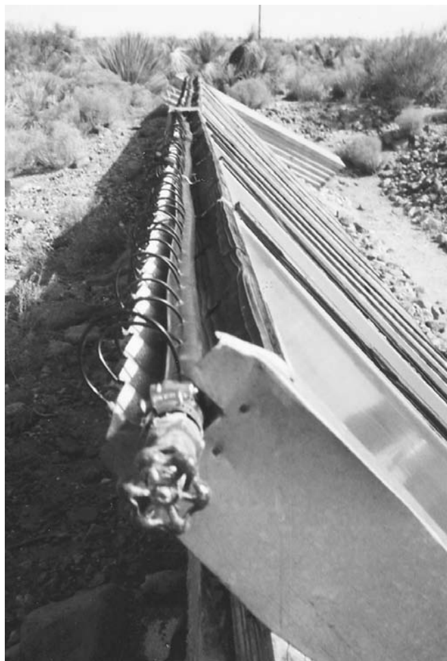
Above: Top view of solar collectors showing the water manifold.
