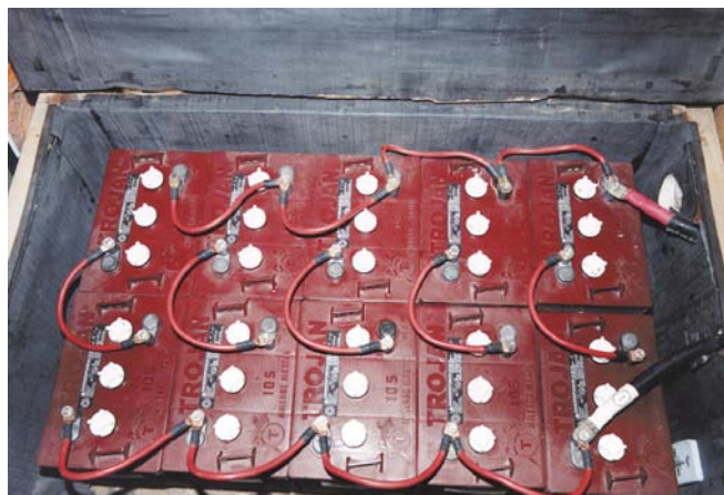
Above: Battery—1100 Ampere-hours at 12 VDC.
