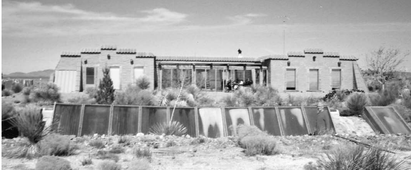
Above: Adobe house in desert setting, with ten house heating panels set into a ditch. Eleventh panel, at right, is for domestic hot water heating.
