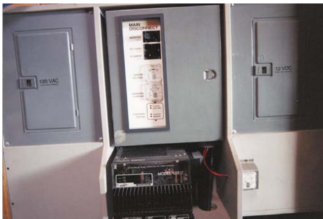
Above: Inverter, instrumentation, and breakers.
