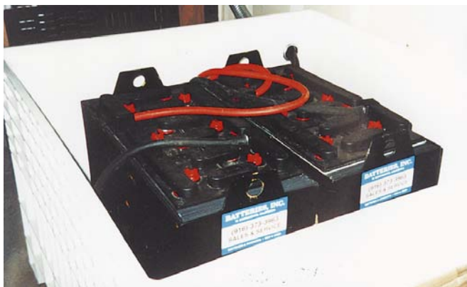
Above: Energy storage: Two Pacific Chloride 6-85-21 lead-acid batteries supplying 1055 Ampere-hours at 24 Volts DC.
