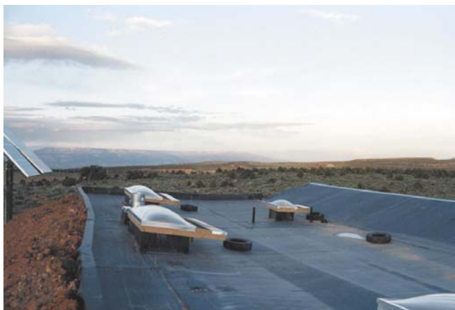
Above: The Earthship's roof is used to collect water.
