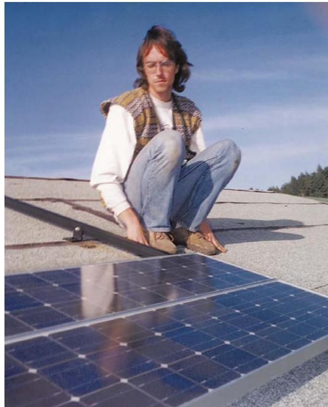
Above: John Gary of Earth Church looks over two PV panels on a rack that can hold six: room for expansion.
