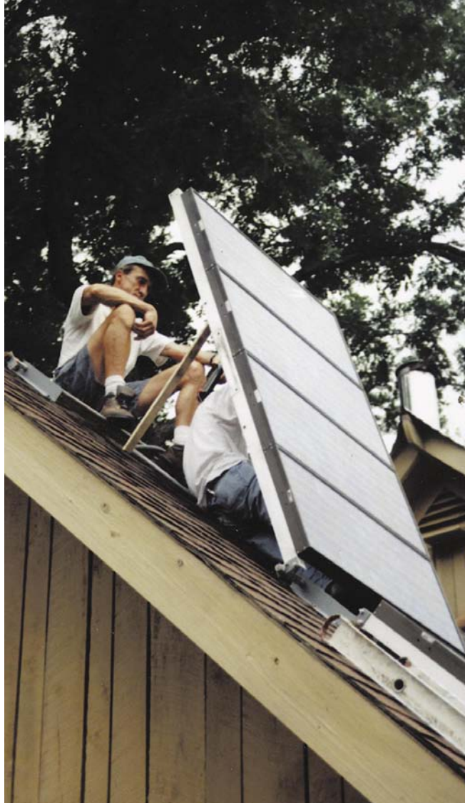
Above: With panels tilted up, series connections are easy to make.
