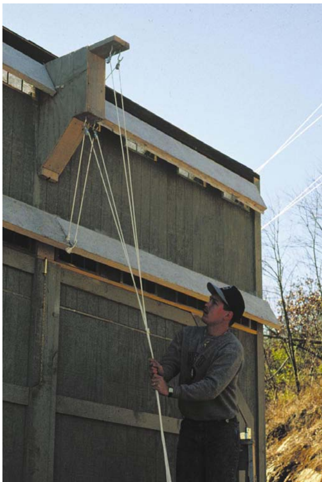
Above: Setting up vent control lines.
