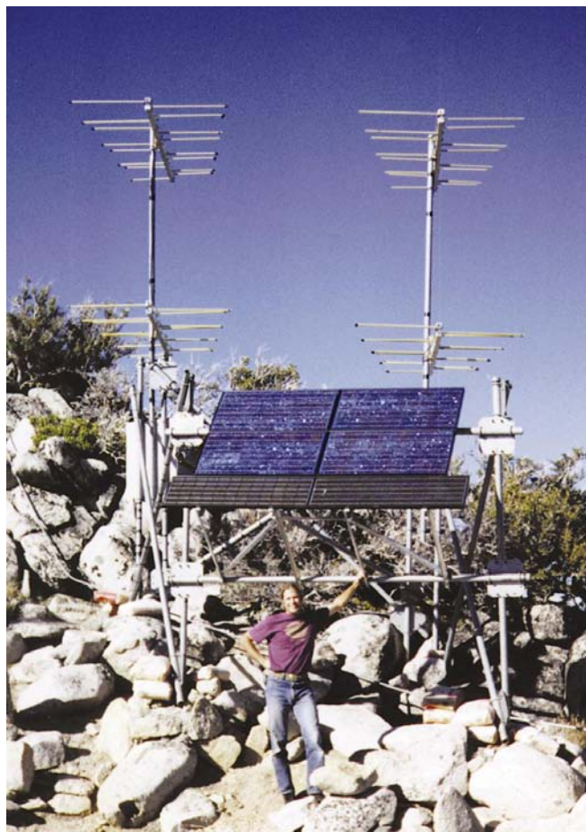
Above: The antenna and photovoltaic arrays at the Boulevard Mountain translator.
