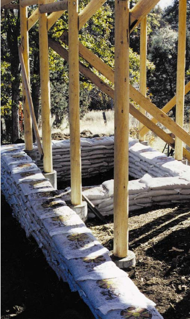
Above: Dirt bag retaining wall/footing along north wall and under future bathing deck.
