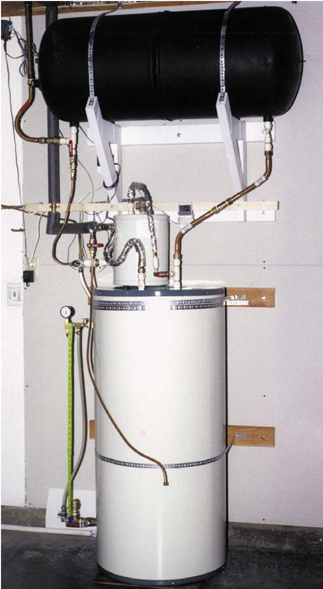
Figure 2: The gravity siphon system.
