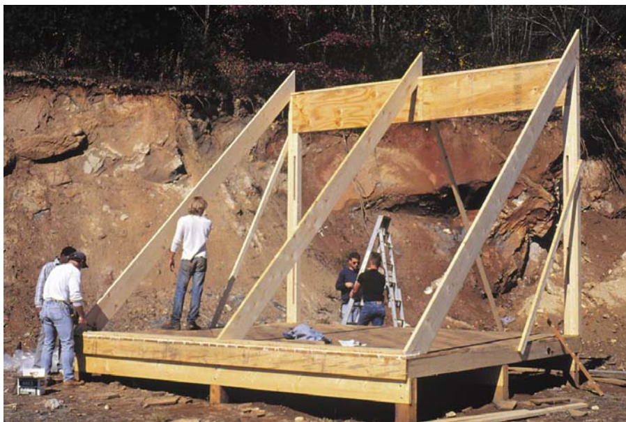
Above: Setting up 2 by 12 south wall rafters.
