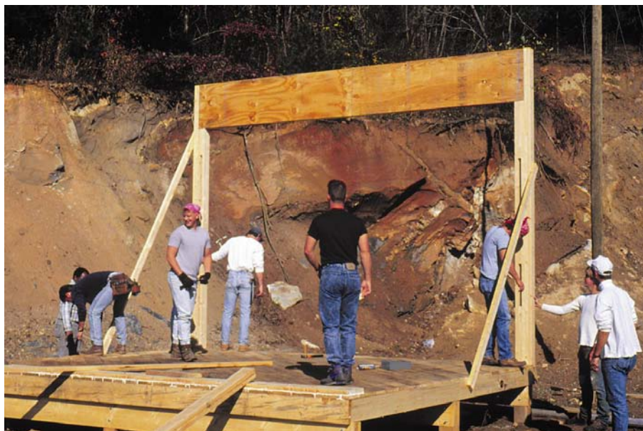
Above: Bracing the north wall.
