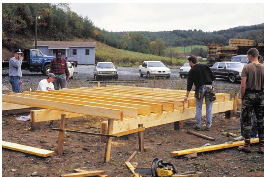
Above: Laying out foundation and floor.
