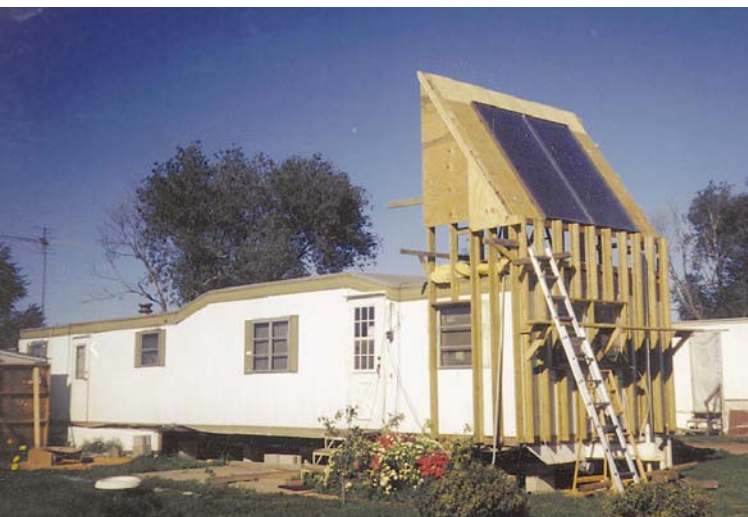
Above: Beginning framework with two hot air collectors.
