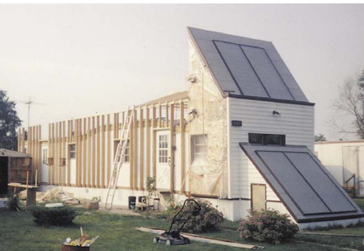
Above: Upper and lower hot air collectors finished. Starting to enclose the rest of the trailer.
