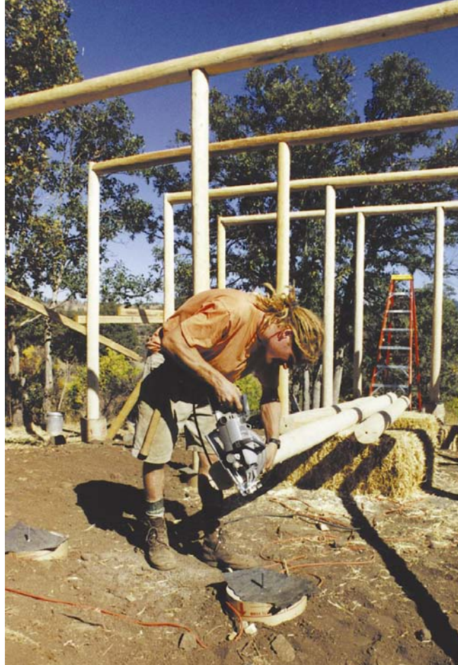
Above: Joe notches beams.
