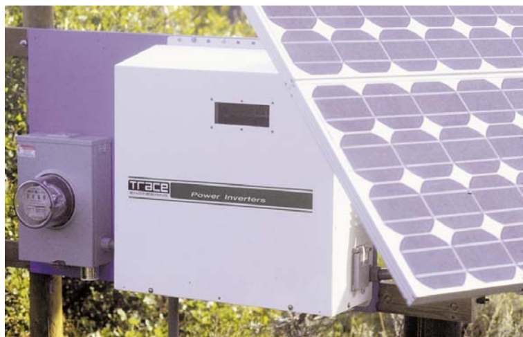
Above: The author's PVs, inverter, and independent kWh meter for measuring energy produced.
