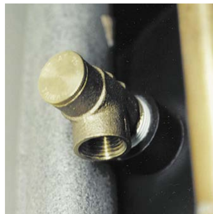
Above, Figure 7. Pressure safety ensured by 75 psi relief valve.
