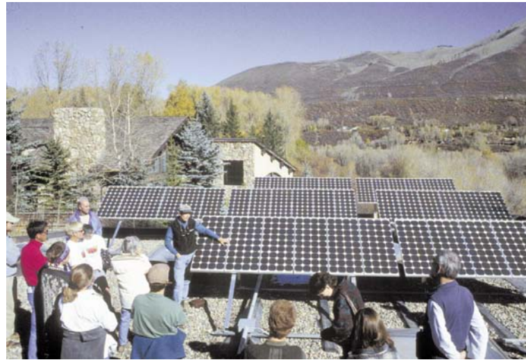
Above: This system contains sixty Siemens modules mounted on two adjacent flat roofs at an Aspen home. We believe it is the largest grid-connected system in Colorado. The 4.5 kW system was a big hit during the National Solar Home Tour.
