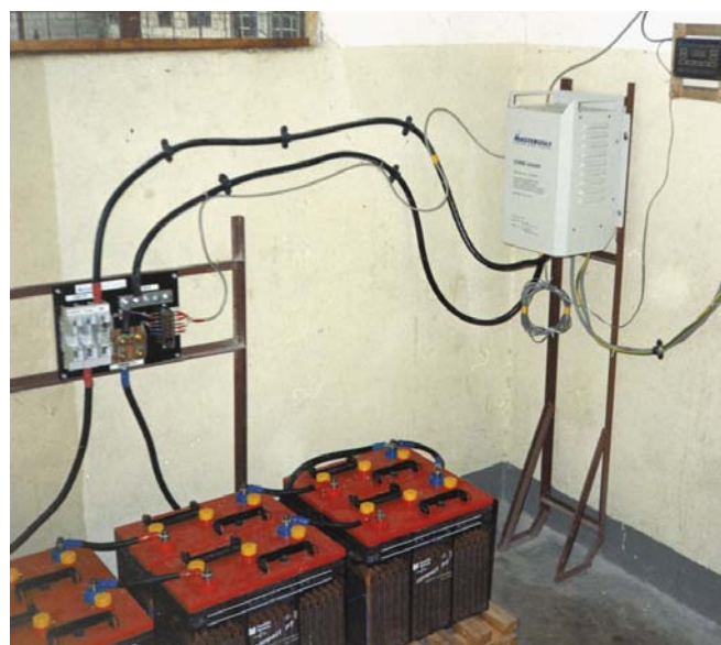
Above: The battery / inverter system.
