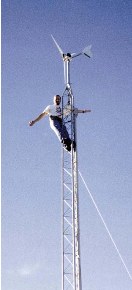
Above: Terry up the tower with his Windseeker 503. He will use this bird and data logging equipment to analyze his wind resource, then might buy a bigger genny.
