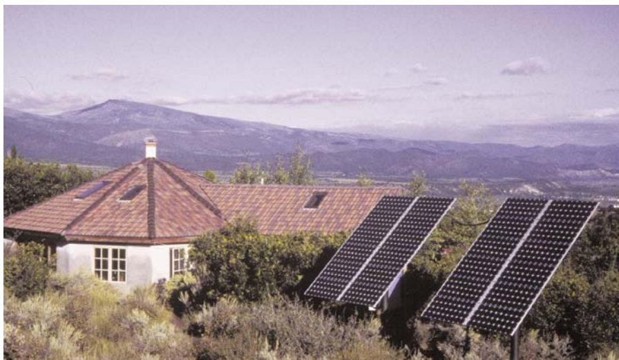
Above: The author's 1.8 kW pole-mounted system in Carbondale, Colorado. The system was installed by a class of Solar Energy International students supervised by Pat Kiernan of Eco Electric.
