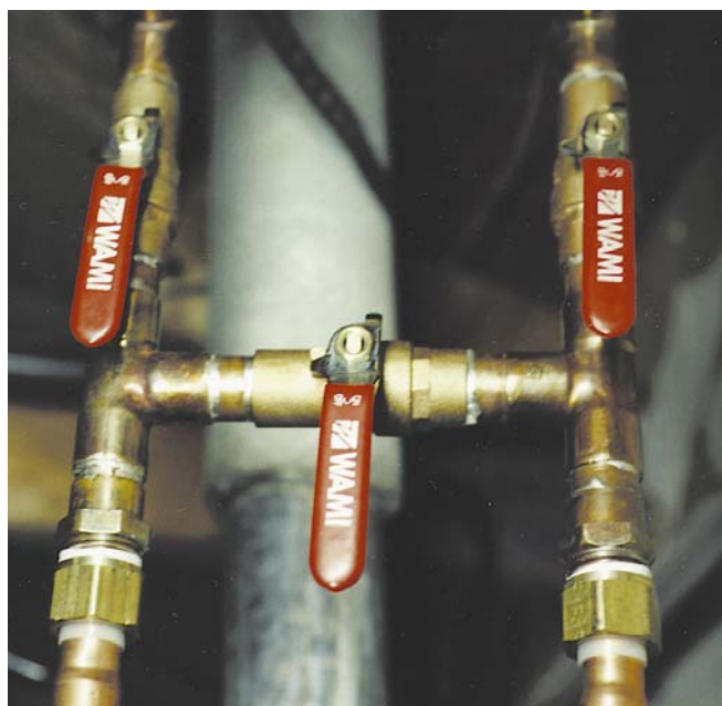
Figure 8. Three valve manifold above backup heater.
