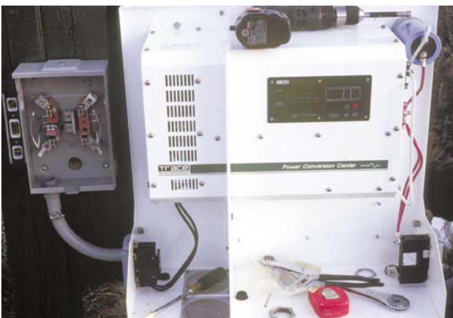
Above: Andrew’s Trace inverter being installed, sans its weather proof cover at this point. Socket box for PV meter is at left.
