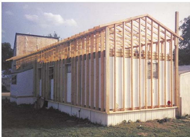
Above: Completed framework ready for roofing and insulation.
