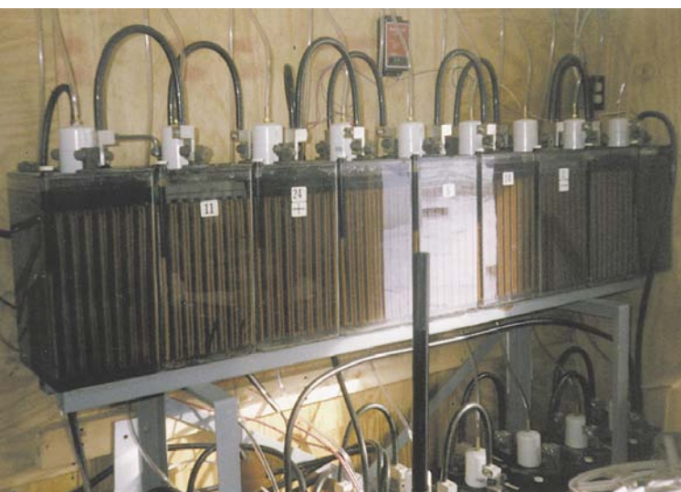
Above: Eighteen 2 Volt cells make up the 2160 Amp-hour, 12 Volt, battery. Notice the home made hydrogen venting system.
