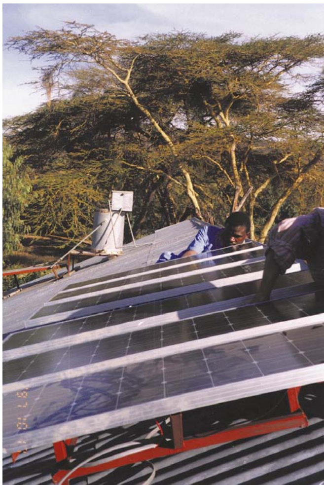
Above: Gaspar Makale wiring PV modules on the Doctor's house.
