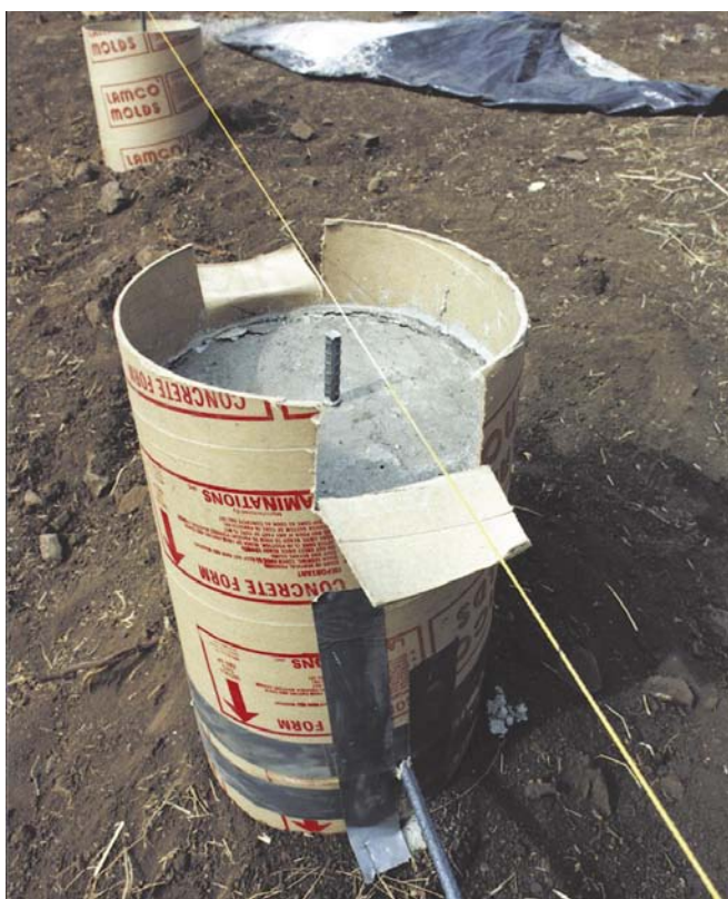
Above: Twelve inch concrete piers extend below frost line. Rebar prevents lateral movement of posts.
