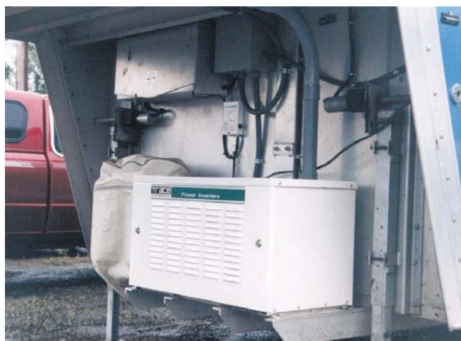
Above: The Trace battery box in place.
