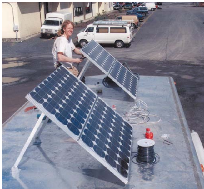
Above: Joe Schwartz, of Electron Connection, installs the four Siemens SP-75s on tilt-up mountings.
