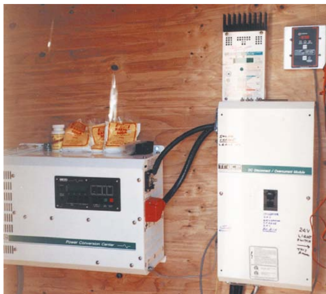
Below: The control center including the modified DC disconnect box.
