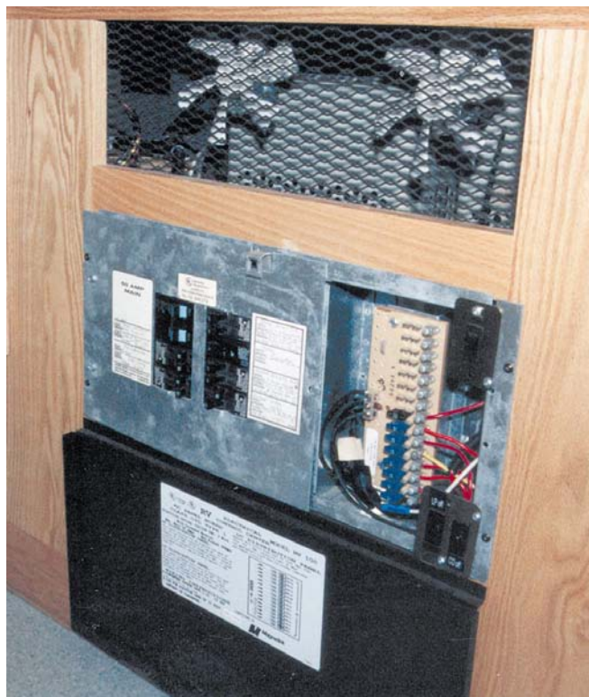
Above: The ac and DC fuse center. The Onan generator and Sola Micro isolation transformer are behind the grill.
