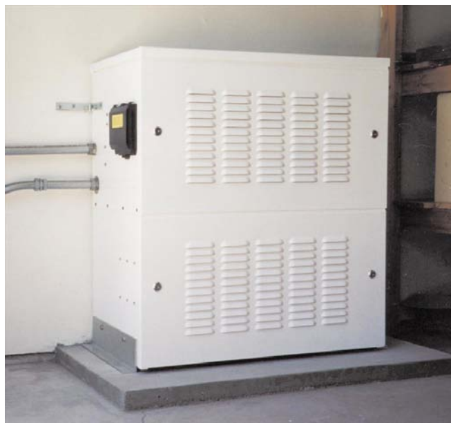
Below: The Power Module closed up tight. Note the earthquake-proof mounting.
