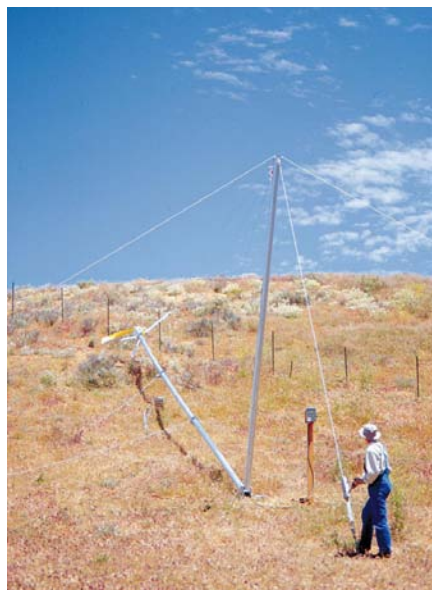
Above: Raising the tower again, this time with the Bergey 850, takes some effort. Going slow allows time for double checking.
