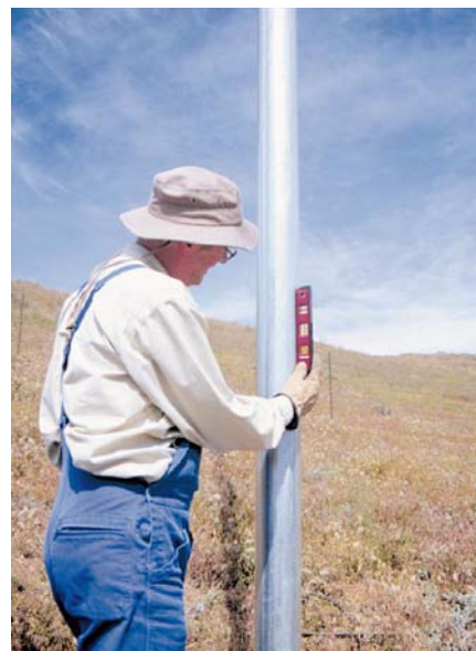
Above: Checking the tower for plumb. The turbine will only yaw properly on a plumb tower.
