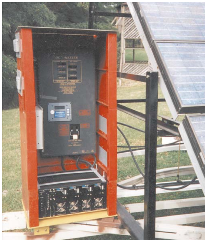
Above: Inside the control center lives the Sun Selector DC Master power center, Omnimeter, pull-out main disconnect, and Exeltech 4KW inverter.
