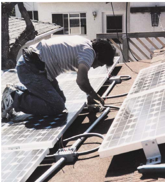
Above: Running the wires in rigid and flexible conduit.
