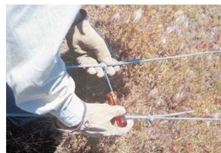
Above: Tightening wire rope clips. Remember, "Never saddle a dead horse."
