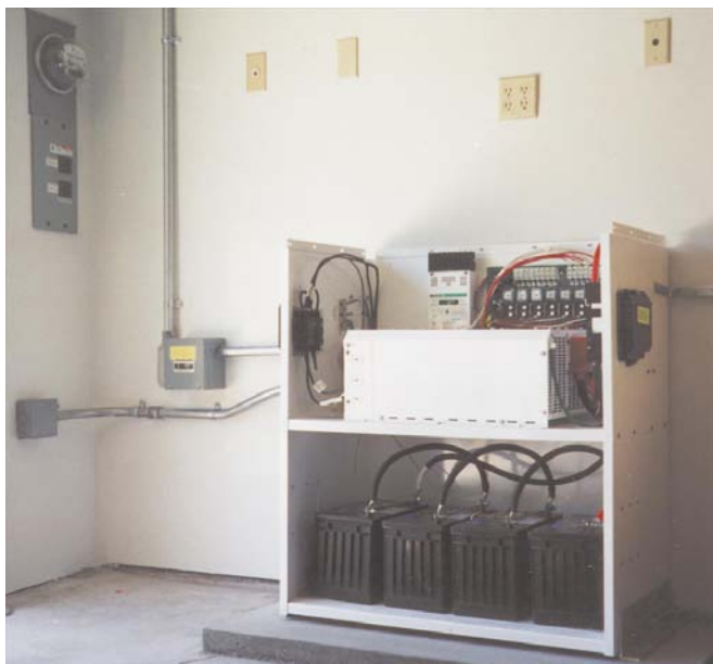
Below: The exposed Trace Power Module with SW4048 inverter, C40 charge controller, and batteries.
