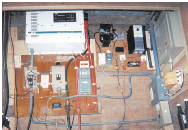
415 VAC becomes 24 VDC at Buena Vista's power center, 2,500 feet from the Harris hydro unit.
