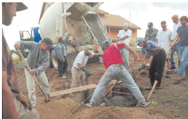
Pouring concrete for the tower anchors.
