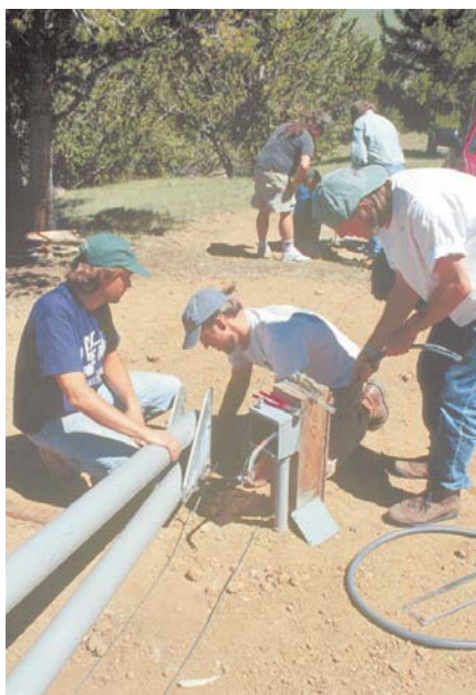
Assembling the tilt-up tower.
