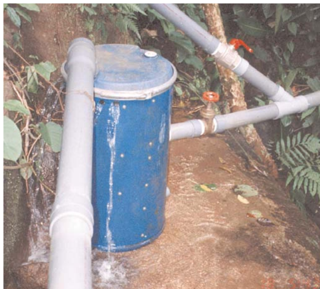
A typical filter tank at the top of the Lebos' penstock.
