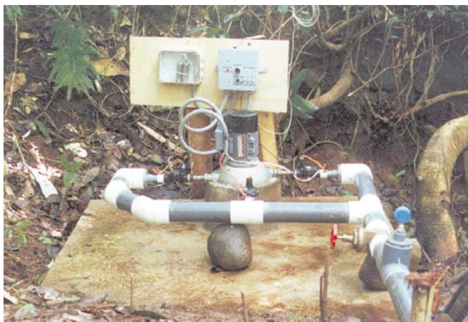
The Buena Vista Lodge uses a 1.5 HP motor to generate 370 watts from a three-nozzle pelton wheel.
