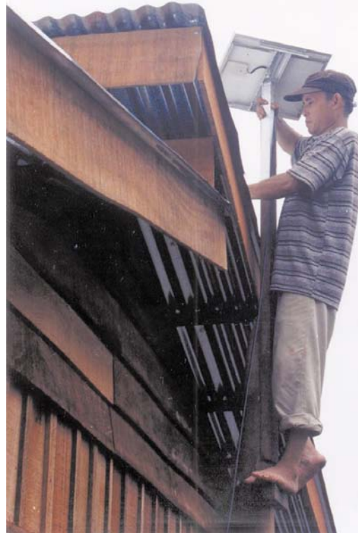
Installing a solar panel on a pole.
