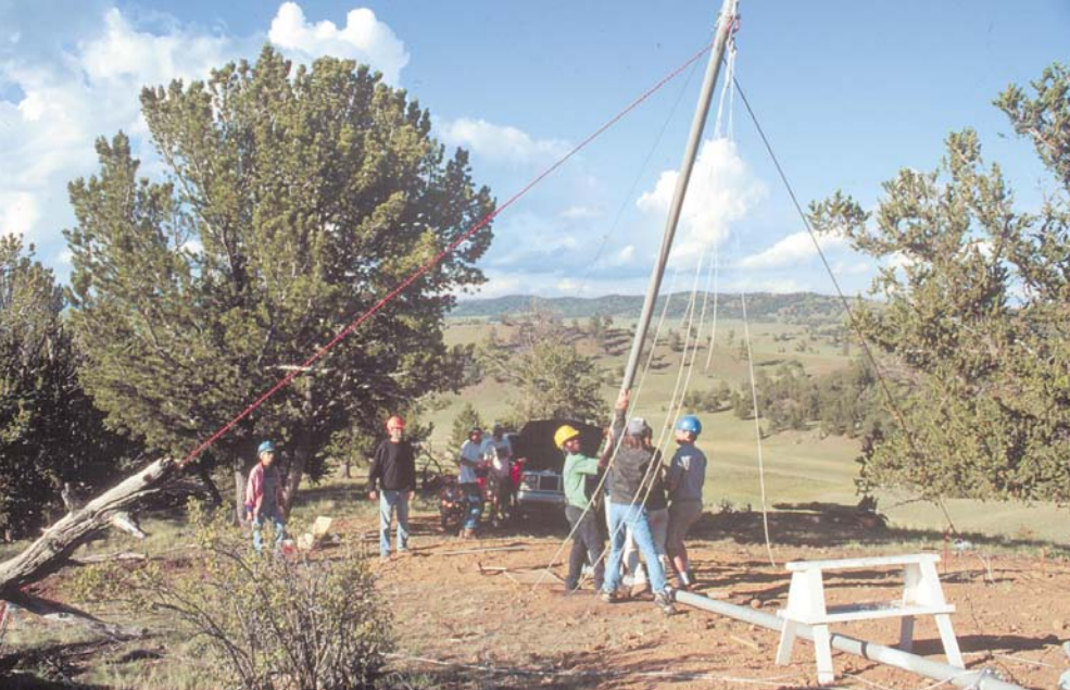
"Heave-ho"ing the tower gin pole into place.
