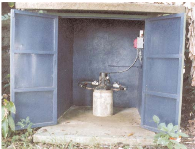
Casa Corcovado Lodge gets 410 watts from 60 gallons per minute at 148 feet of head.
