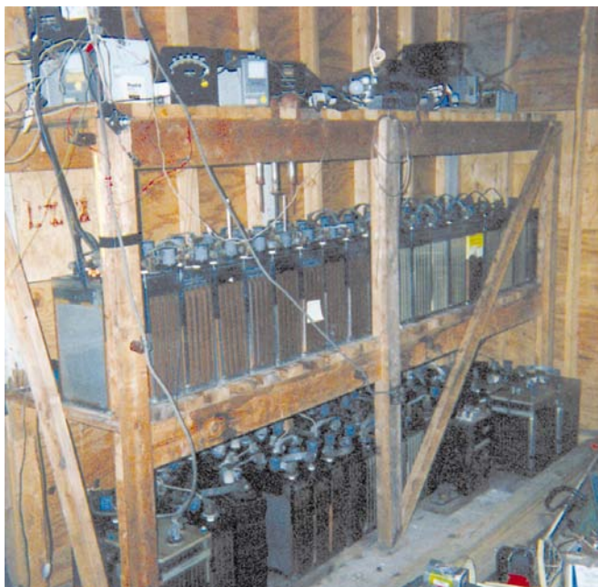
Half of the 120 lead-calcium cells.
