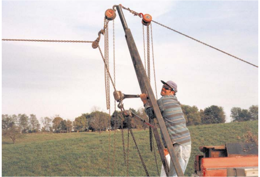
Lonnie cranking the tower up from the back of Nelson's boom truck.
