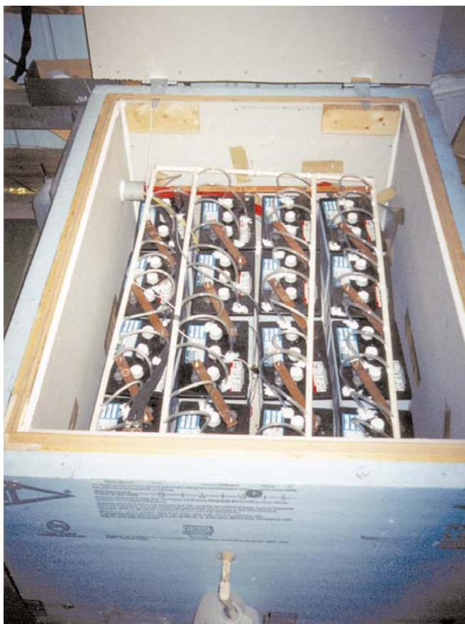
Sixteen HiTech batteries and their insulated box.
