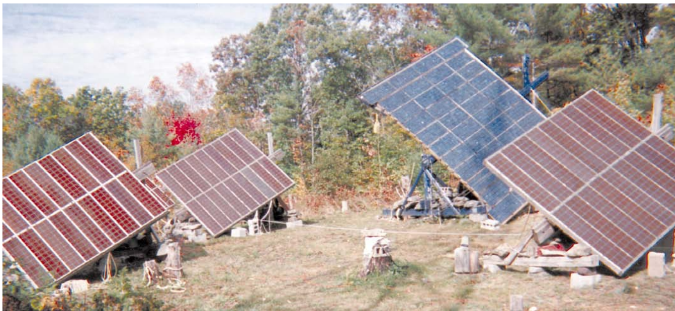
Four of the five PV arrays. Total PV output is about 3,000 watts.
