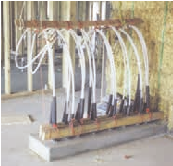
Tubes gathered and ready for a manifold.
