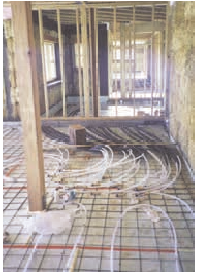
A tangle of tubes come together at the location of the future manifold in the main house.
