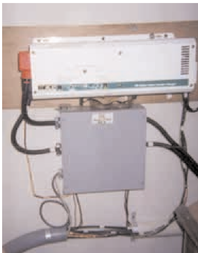
DC power comes in from the modules, through the safety disconnect (left) and charge controller (right), and then goes to the batteries. Power for DC loads comes directly off the batteries through the DC load center (below).
