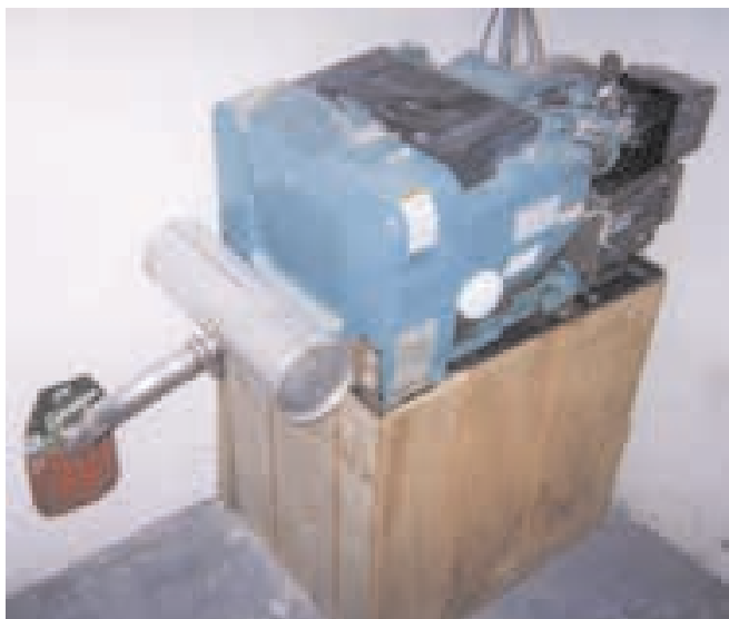
The 4 KW Onan generator in the north room of the power shed. The air intake is under the wooden stand.
