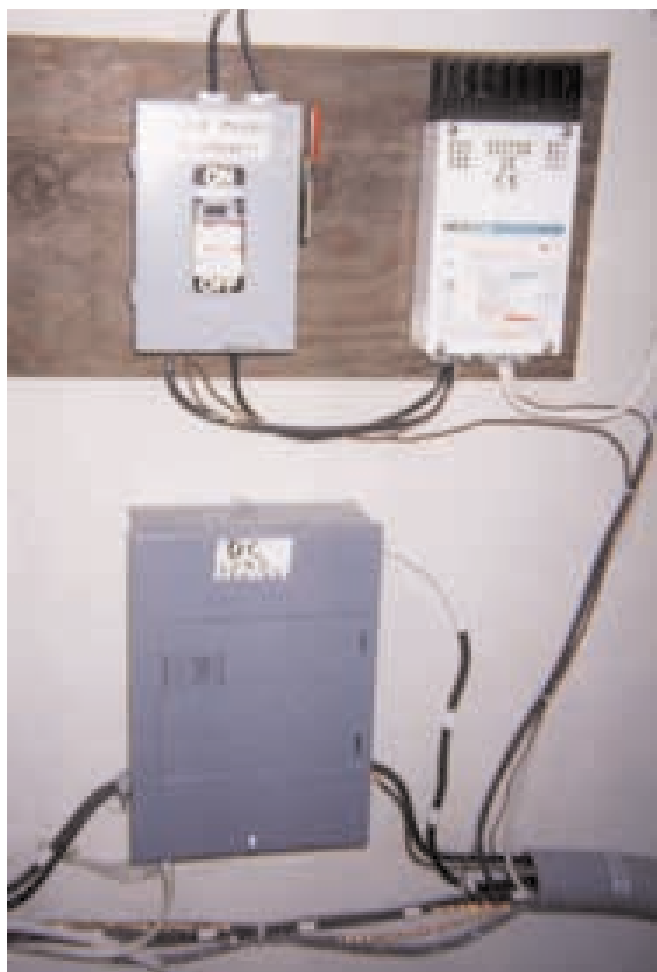
DC power comes in from the modules, through the safety disconnect (left) and charge controller (right), and then goes to the batteries. Power for DC loads comes directly off the batteries through the DC load center (below).
