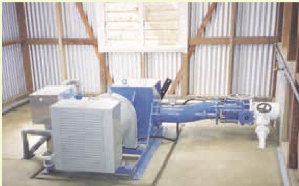
A typical Canyon Pelton (75 KW ) in a remote area of Papua New Guinea.
