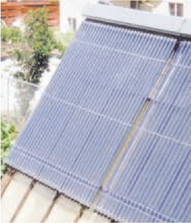
Eight Thermomax panels, with thirty evacuated tubes each, generate hot water for space heat and DHW.
