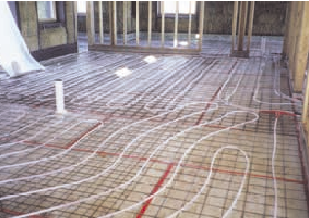
The Edisons' home, waiting for concrete to be poured. PEX tubing is tied to the weld wire to hold it in place during the pour.
