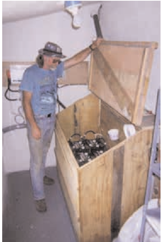
The vented battery box is built onto two small pallets to keep the batteries off the floor. Twelve Interstate 6 volt, 350 AH batteries provide 1,050 amp-hours at 24 volts.
