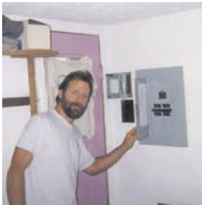
Chip Boggs flips the AC load center's main breaker in the house.
