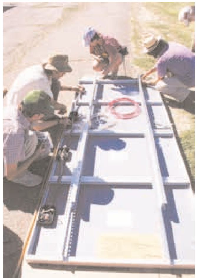
Top: Hey, the rack is too small for these PVs.... Bottom: A successful rack klüge using steel angle iron.
