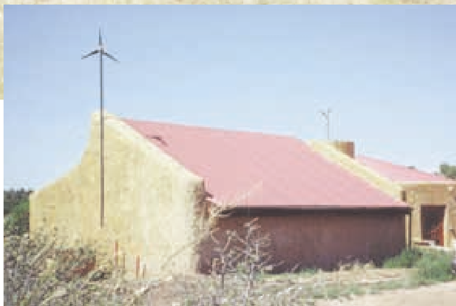
The shop contains the renewable energy system.
