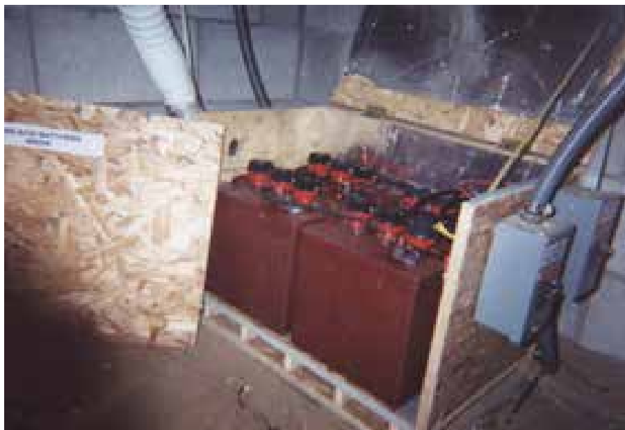
Four Trojan T-105 batteries, 440 AH at 12 VDC. Note the Hydrocaps, DC disconnects, and removable front wall on the box.
