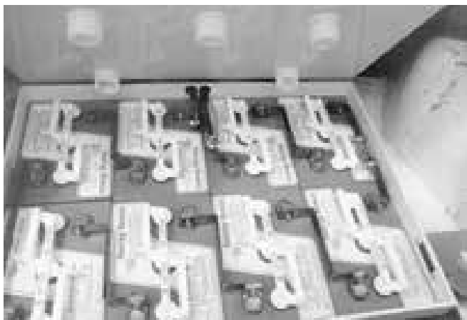
The tubes on the lid of this box press down to hold the batteries firmly in place.
