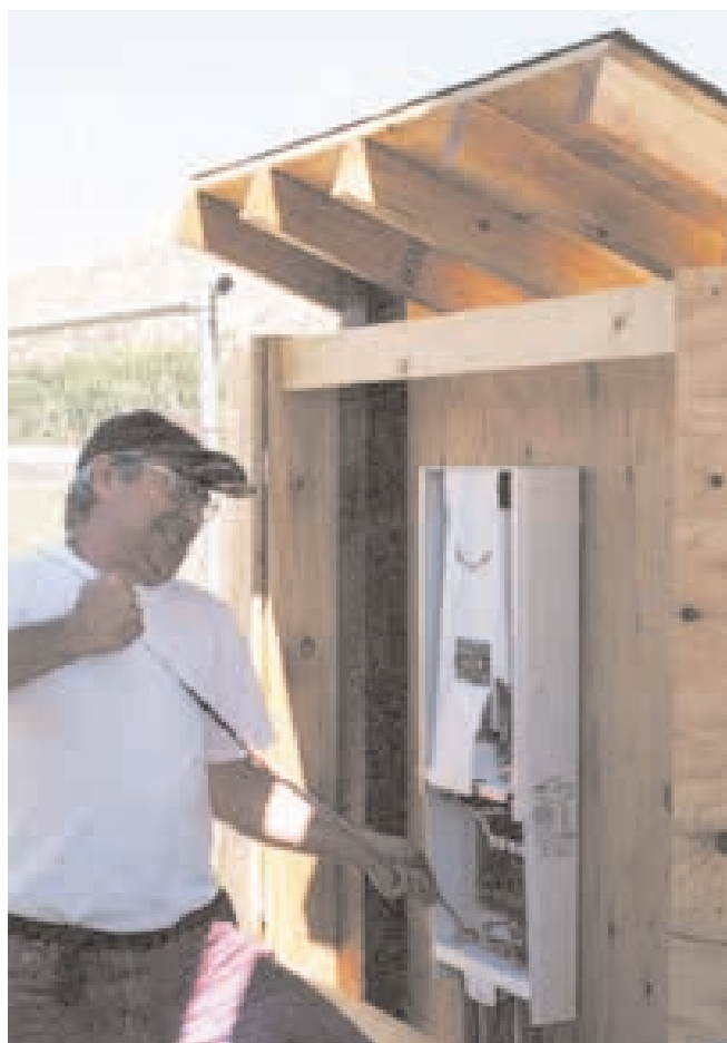
Top: Attaching the home runs to the array. Bottom: Pulling the home runs through the conduit and into the inverter.
