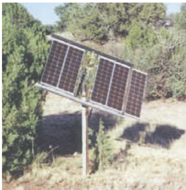
Five M-75 Arco panels on the south of the house.
