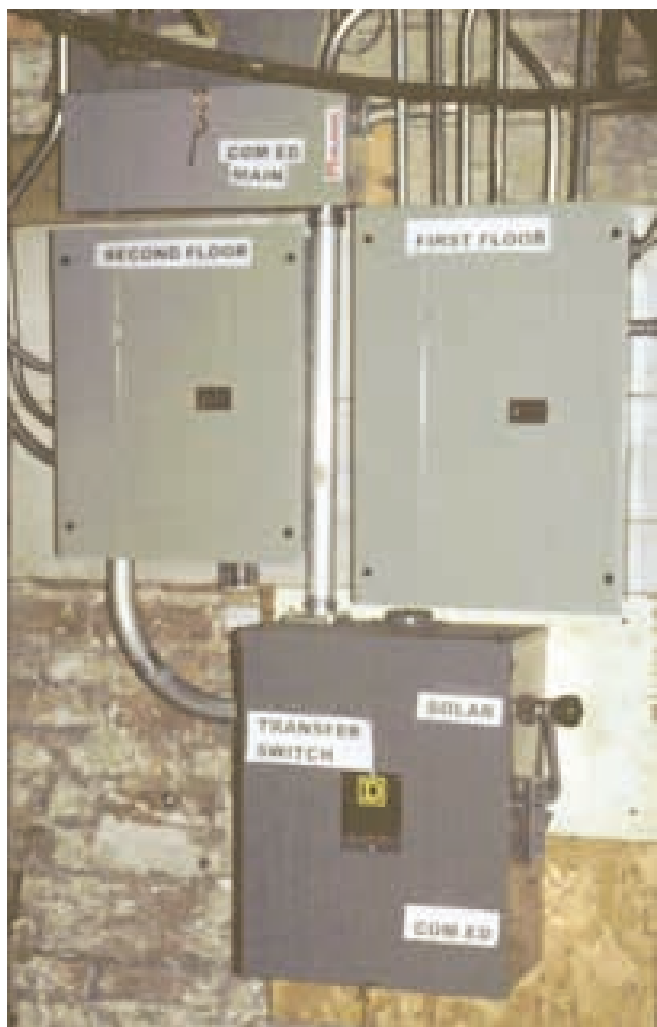
Renewable energy or the grid—notice the position.
