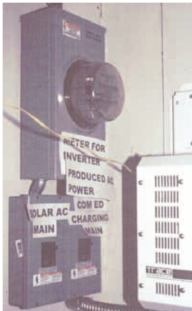
All solar energy is counted with a KWH meter.
