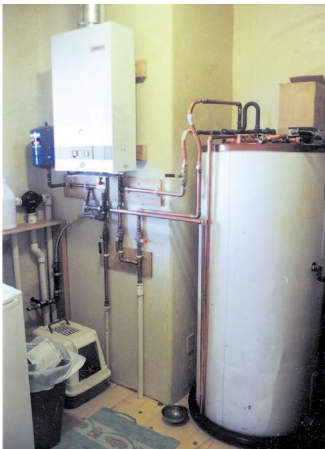
An Aquastar BS on-demand water heater (upper left) backs up the solar hot water system.
