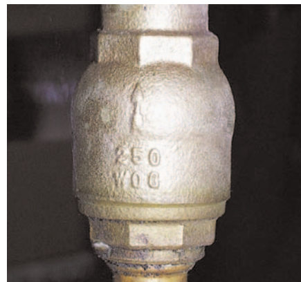
A check valve allows flow in only one direction, (see arrow).
