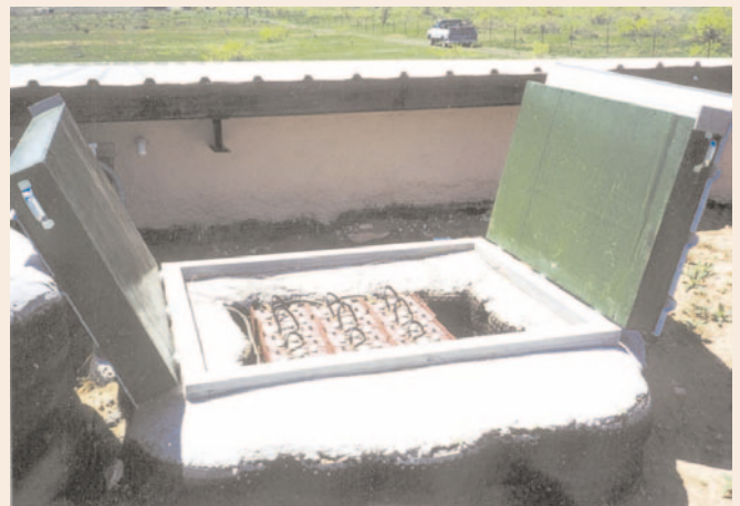
A rammed earth and tire battery box.
