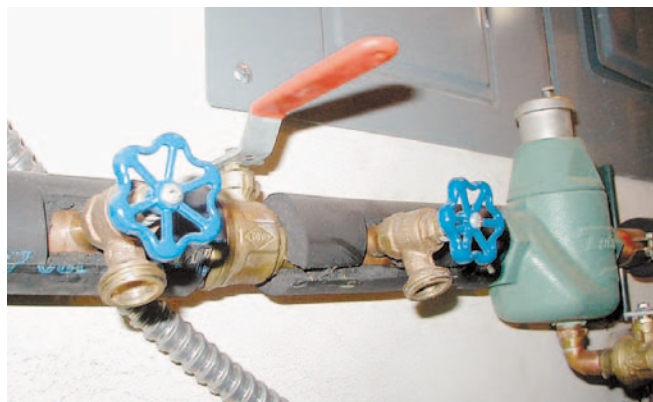
Three valves make up the drain/fill assembly.
