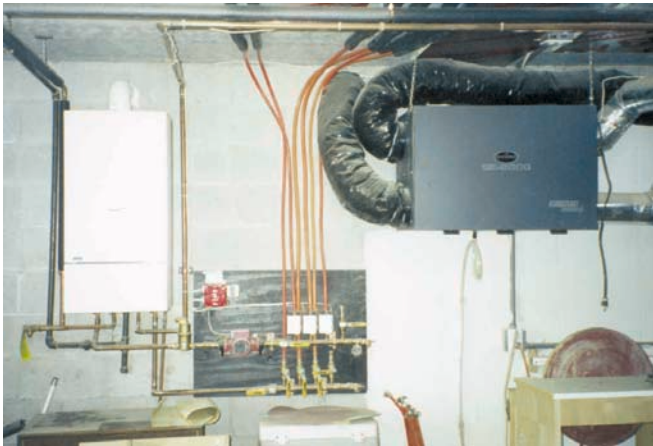
The natural-gas-fired boiler (left) and heat recovery unit (right). Note the basement ceiling is Spancrete.
