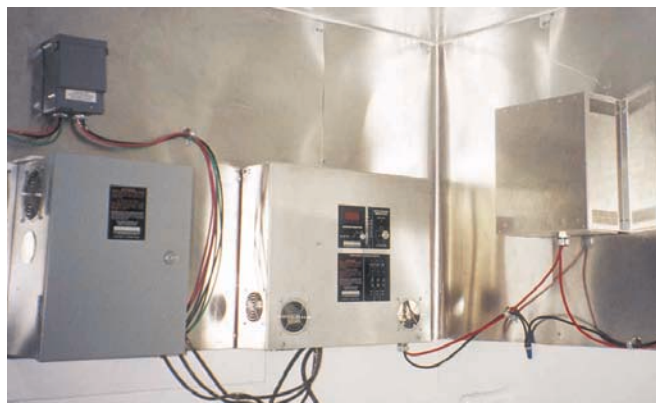
The Whisper EZ-Wire Center, step-down transformer, and diversion load heater box in the power room.
