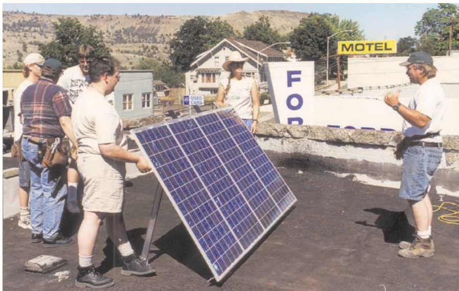
Four Photowatt PW1000, 90 watt modules, in the relentless Eastern Oregon sun, should easily meet the office loads .
