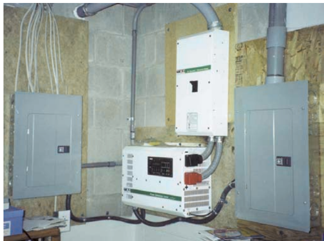
The DC disconnect box, inverter, and two subpanels are located in the basement, and the batteries are in the garage above.
