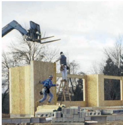
Structural insulated panels (SIPs) form the entire house structure. A small crane sets the SIPs into place.
