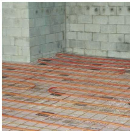
Basement during construction, showing 2 inches (5 cm) of insulation on the floor and radiant floor tubing. The repaired holes in the cement block are where expanding foam insulation was injected inside the 12 inch (30 cm) blocks.
