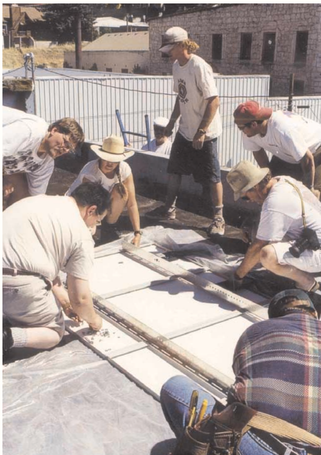
Rack 'em and stack 'em—Sixteen students learned about photovoltaics while helping to install the system.
