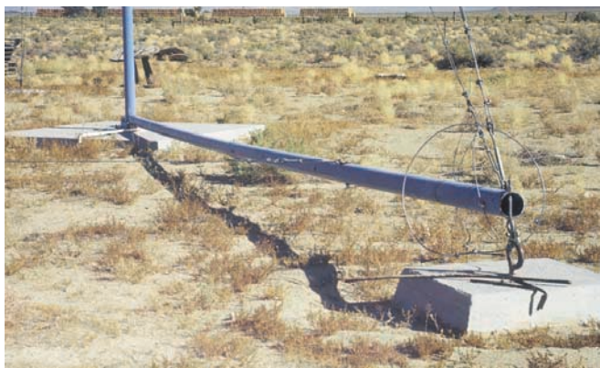
Sandy soil necessitated large concrete footings for the 70 foot tall tilt-up tower.
