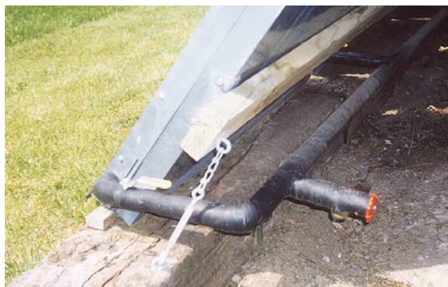
The three Yazaki panels are anchored to railroad ties.
