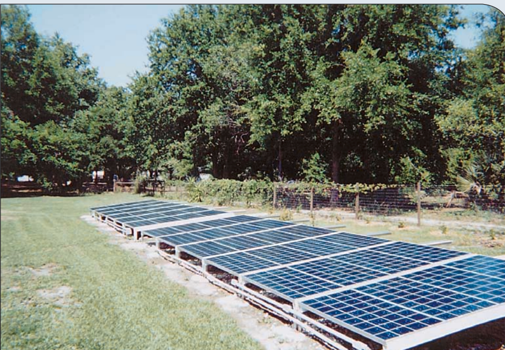
The two identical arrays—each has 24 Kyocera 120-1, 120 watt panels.
