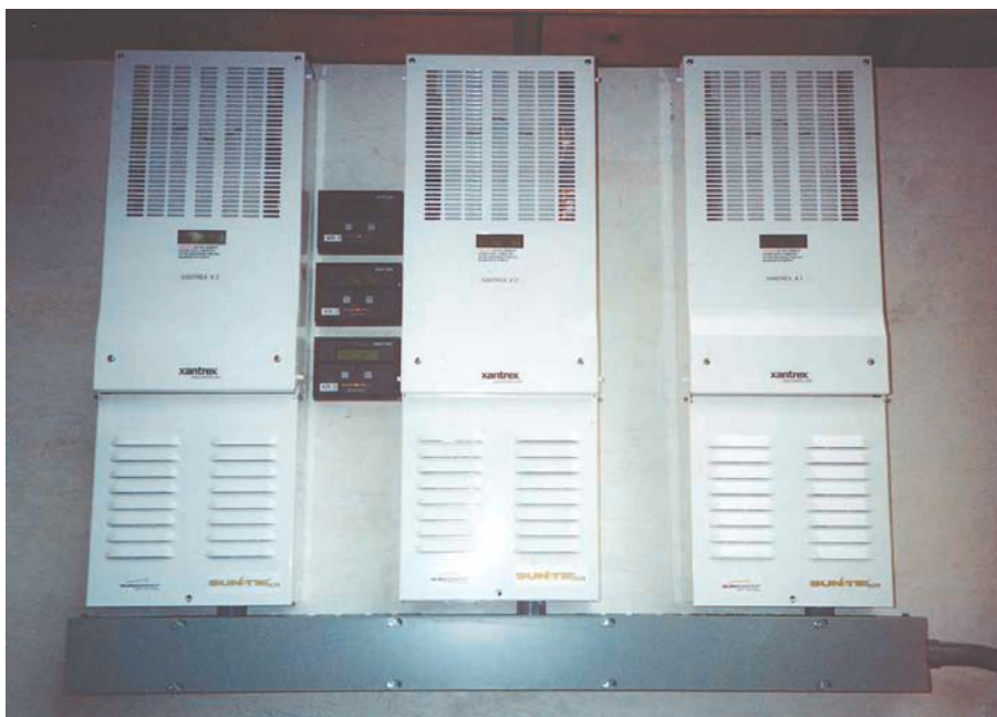
Three Xantrex Sun Tie XR inverters pump green electricity into the utility grid.
