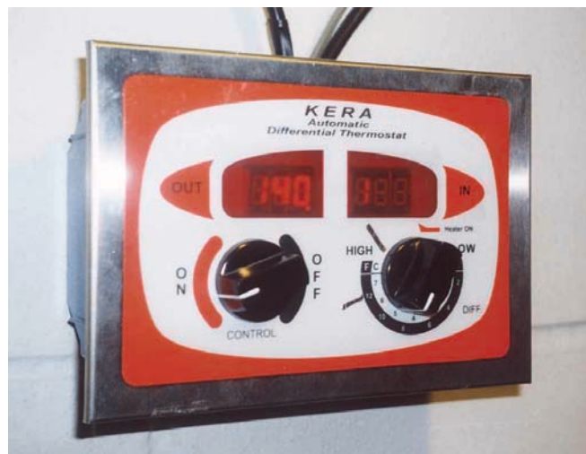
A Kera differential thermostat controls operation.
