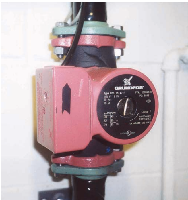
The single, AC powered, Grundfos circulating pump.
