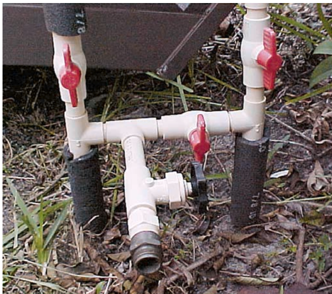
Bypass valves on the solar batch heater allow for draining the tank.
