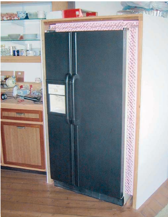
Refrigerator in enclosure, lined with foam insulation.
