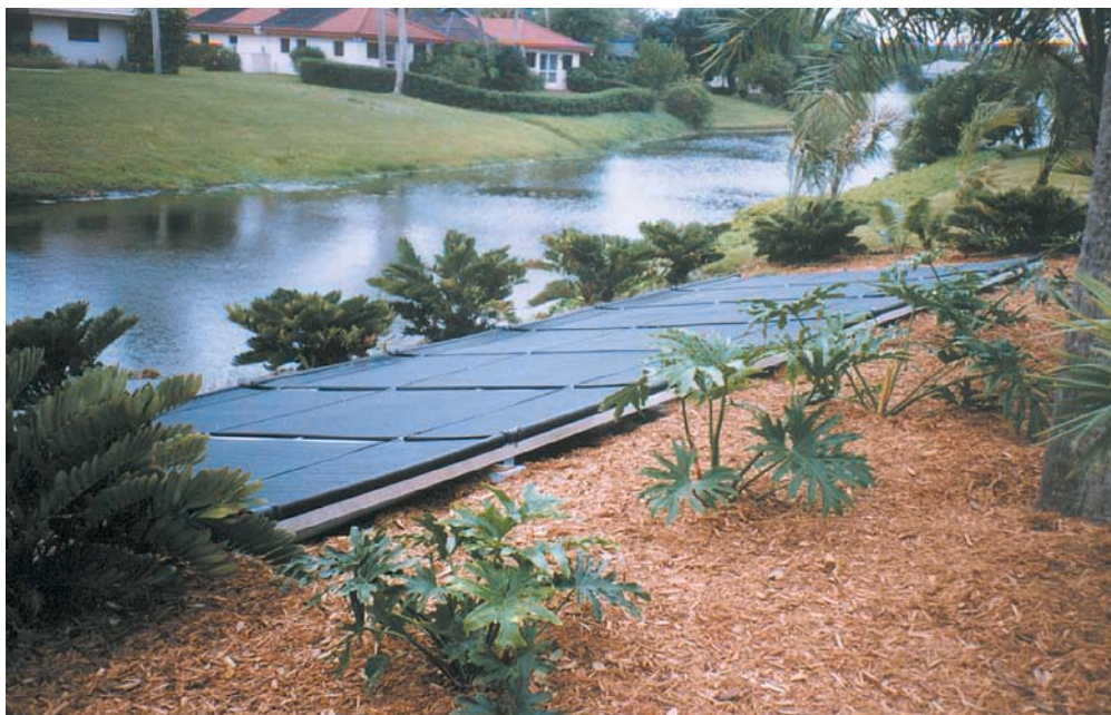
A ground-mounted collector is subject to plant shading and more wear.
