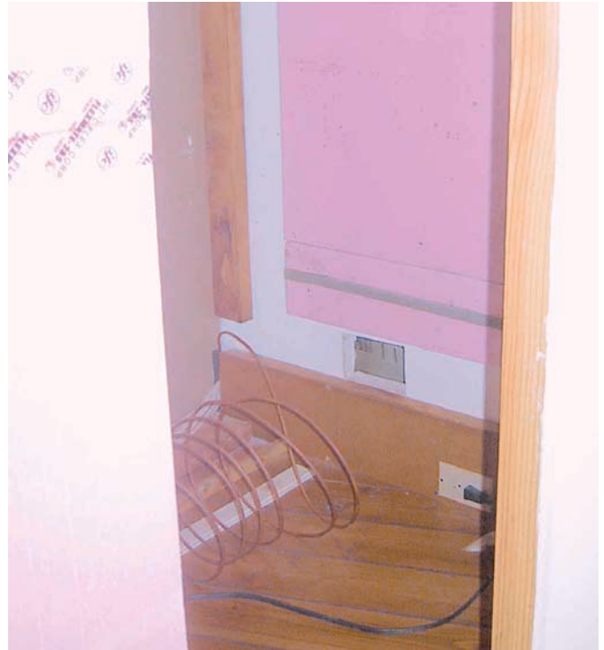
A vent is cut in the wall in the back of the enclosure. The copper coil is the feed for the ice maker.
