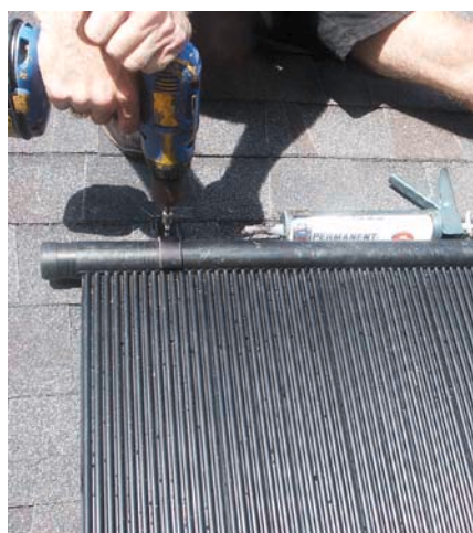
Metal pipe clamps 1/2 inch larger than the pipe hold PVC pipe and collector headers securely to the roof. A generous amount of quality sealant is used to prevent roof leaks.
