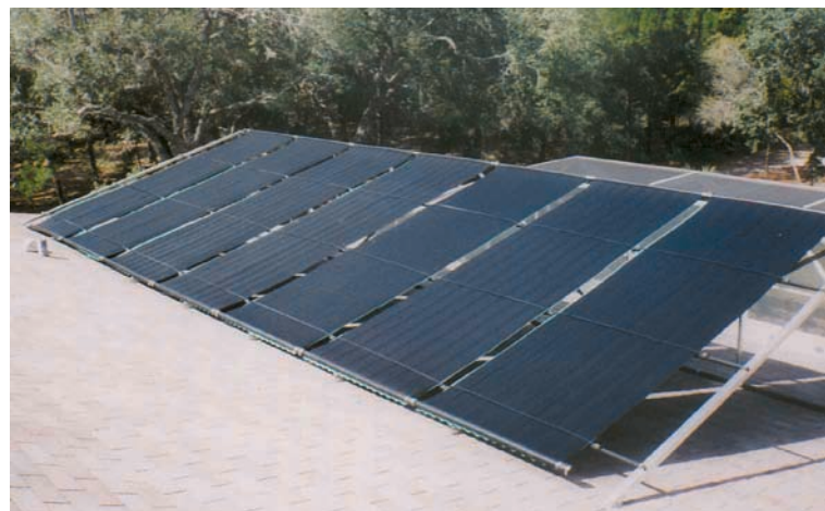
South-facing solar collectors on a north-facing roof.
