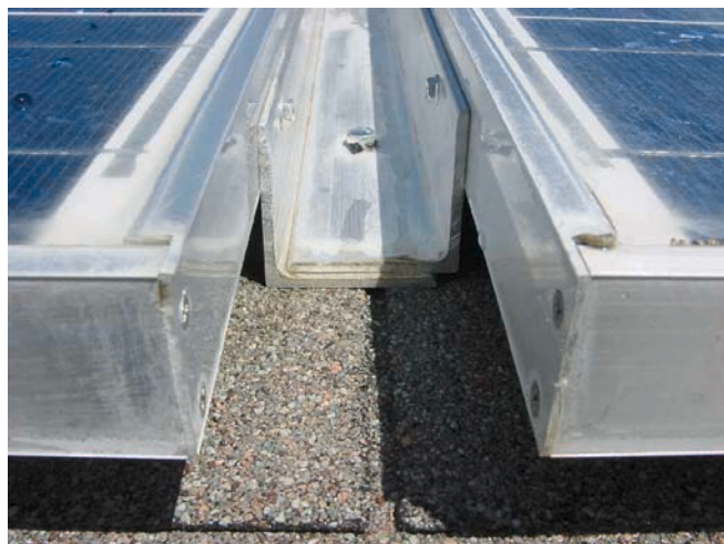
Doubling up the mounts minimized holes in the roof.
