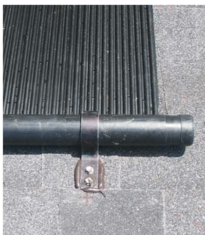
Metal pipe clamps 1/2 inch larger than the pipe hold PVC pipe and collector headers securely to the roof. A generous amount of quality sealant is used to prevent roof leaks.
