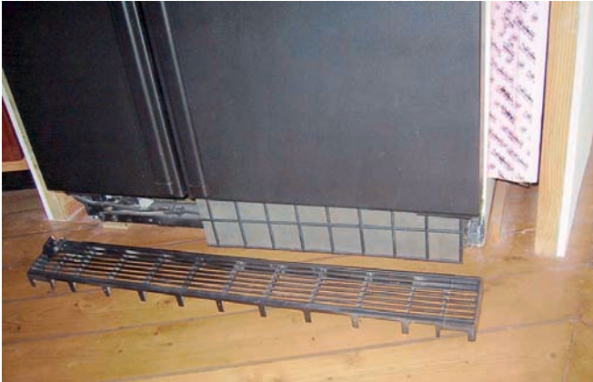
A piece of air conditioning filter is used to slow dust buildup on the coils. Front venting is pretty close to "normal."
