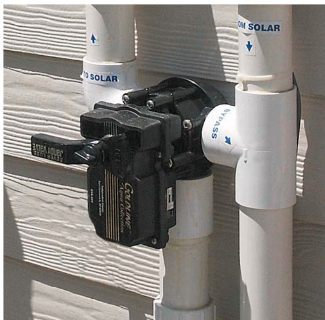
The automatic diverter valve bypasses the solar collector loop when the pool reaches the desired temperature.
