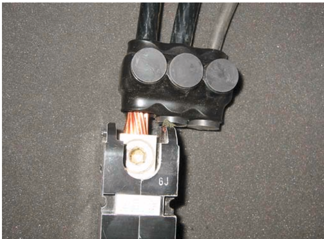
Multiple conductor connectors by NSi Industries provide pre-insulated connection for various sizes of wire.
