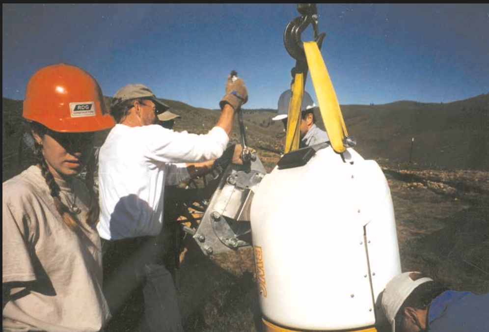
The crane holds the weight while the Bergey Excel is bolted to the tower top.
