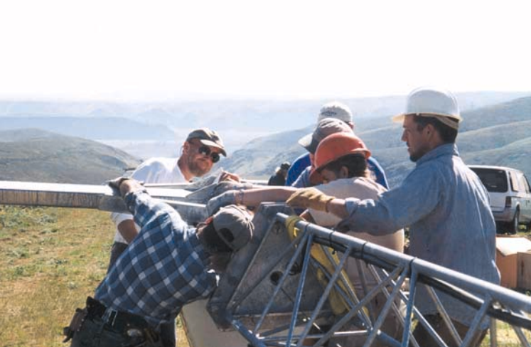
Muscling the Bergey's tail into position.
