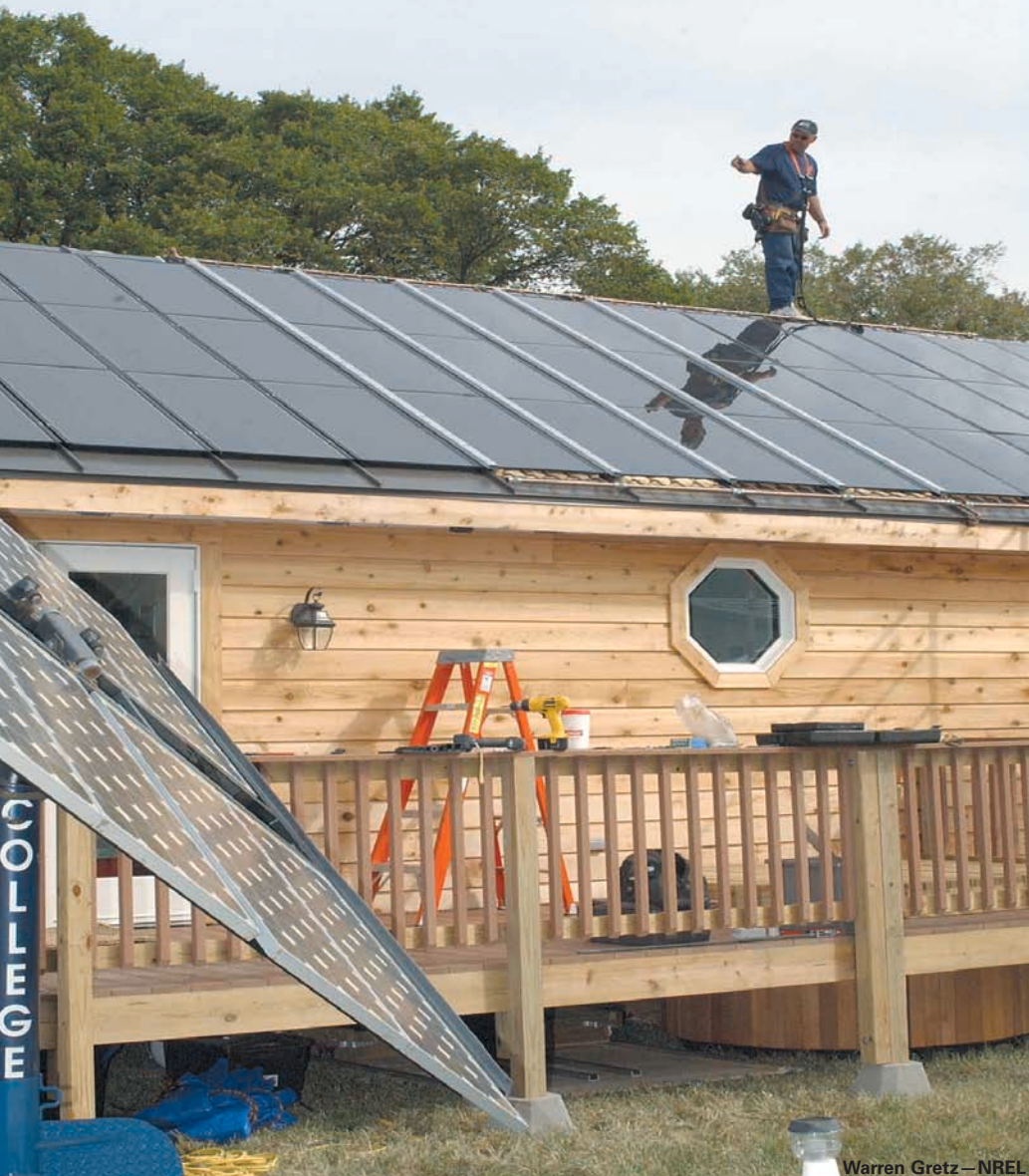
Crowder College's experimental building integrated PV and solar thermal system. Note the exposed plumbing below the PVs on the roof—insulated hot water transfer tubes run below the PVs and heat-absorbing plate.
