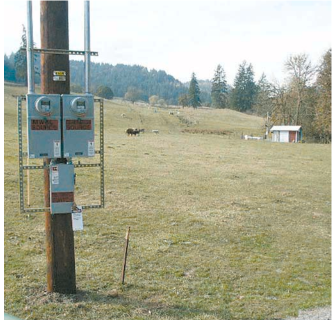
Two KWH meters measure grid energy to the farm and hydro energy to the utility grid. Below is the disconnect required by McMinnville Water & Light. The shed that houses the turbines and controls is in the background.
