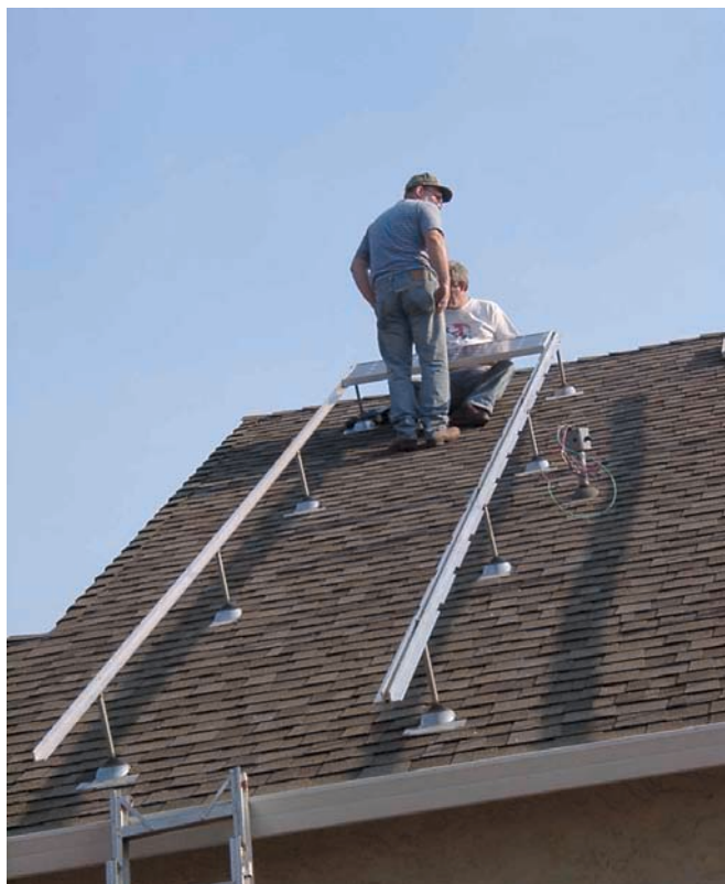
Installing the first PV module.
