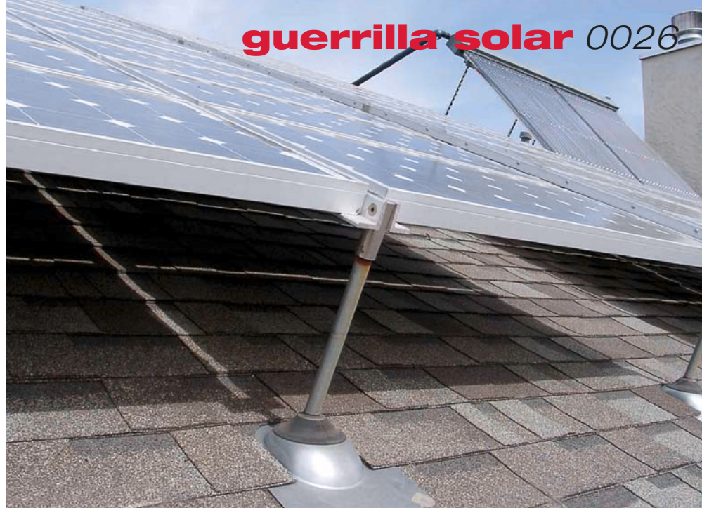
Close-up of PV rack support, with hot water collectors in background.
