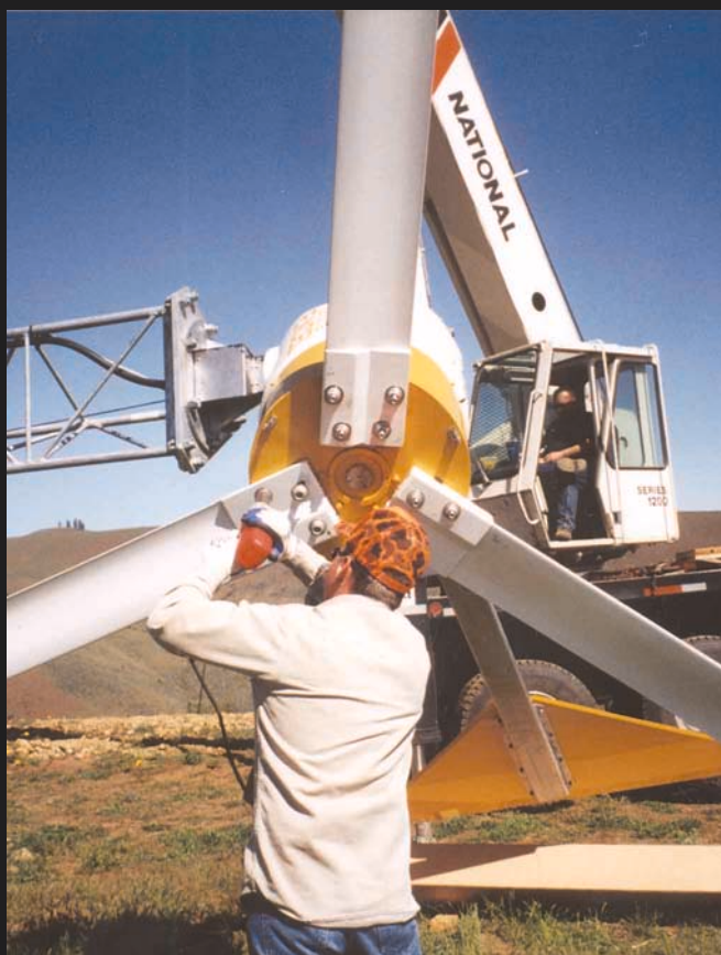
Mounting the blades using an impact wrench.
