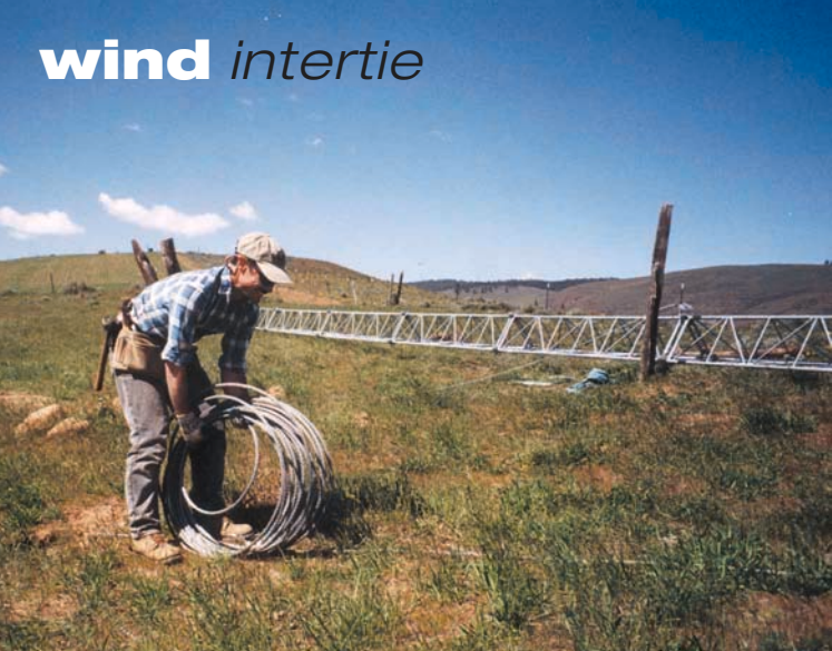
Rolling out the guy wires.
