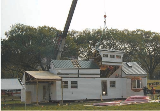
In Maryland's modular construction, the tech pod was located on the left side of the building, next to the carport.
