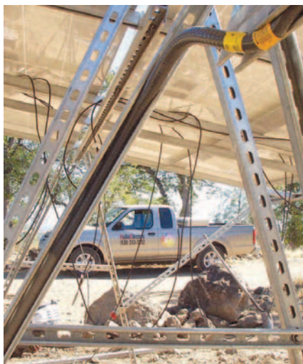
The Carflex conduit is pressed into the rack's channel.
