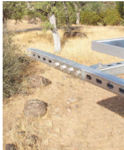
To extend the front arm, splice on an additional piece of Power Strut with a four-hole plate or sleeve.
