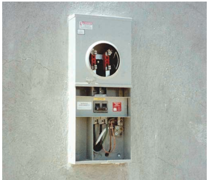
An AC service disconnect, with the meter yet to be installed.
