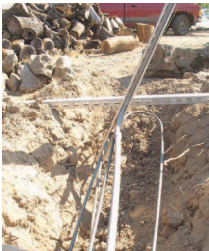
The arrays are leveled with pieces of Power Strut laid on the ground.
