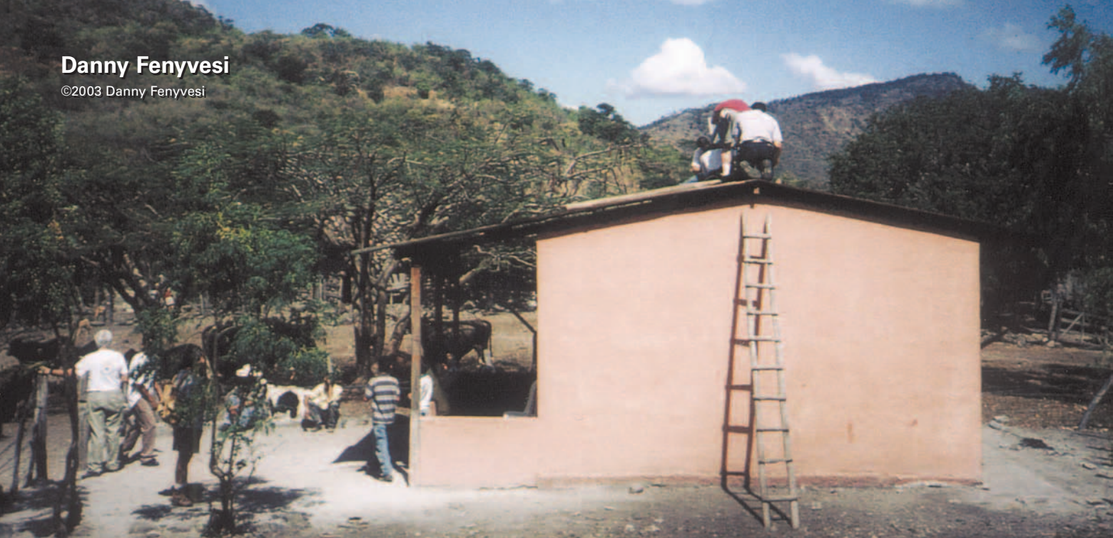
Grupo Fenix workshop participants install a 50 watt photovoltaic panel for lighting on the health clinic in the little village of Las Pintadas, Nicaragua.
