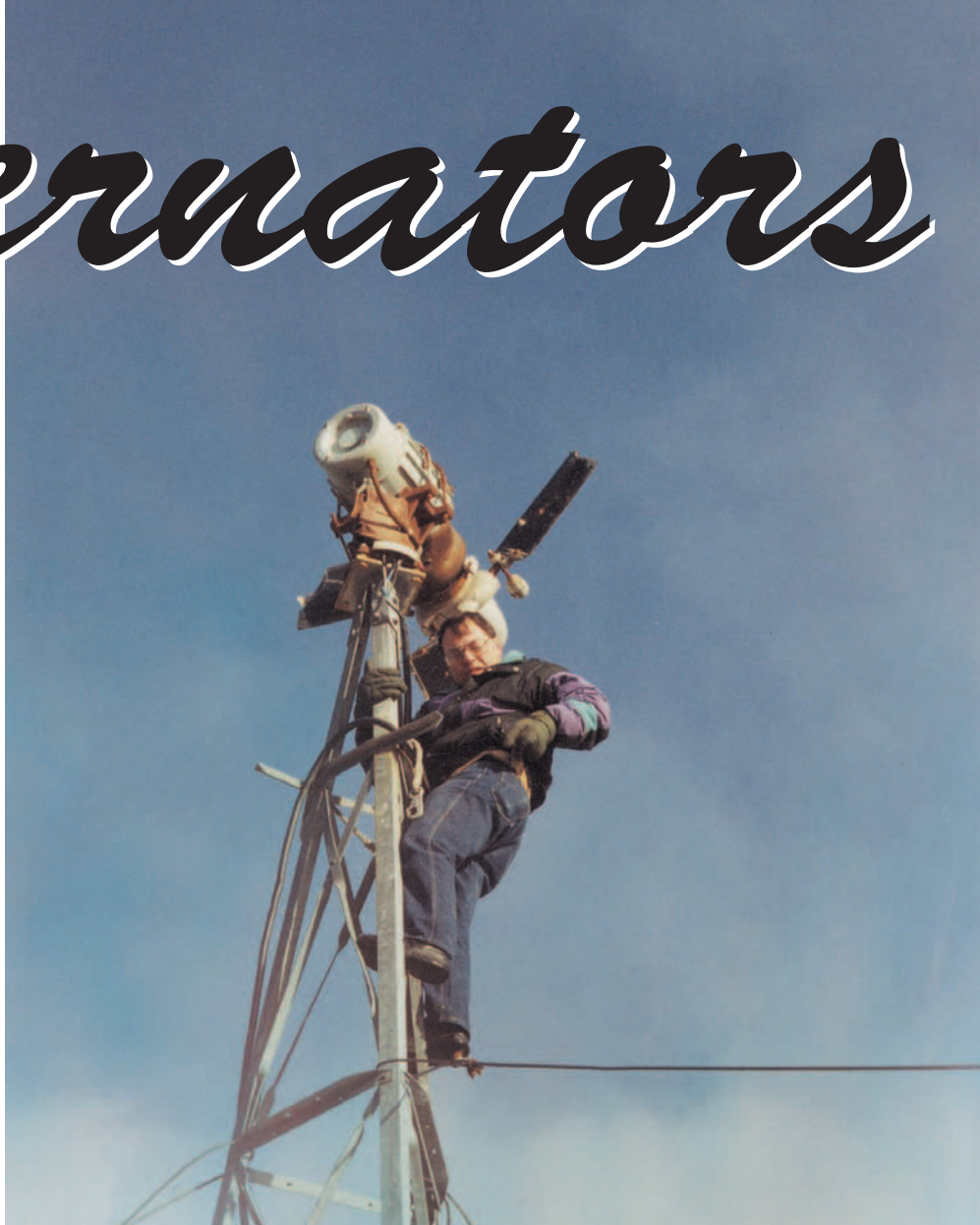
The author prepares to repair a Dunlite BL, 2 KW wind generator that uses a brushless, 3-phase alternator.
