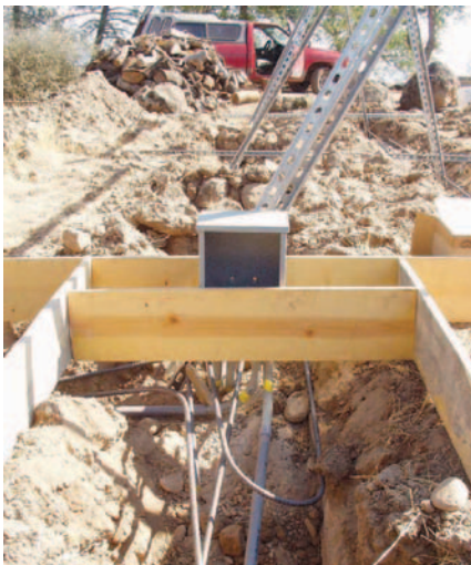
The junction box prior to the concrete pour—it can also be easily attached to a rear array leg.
