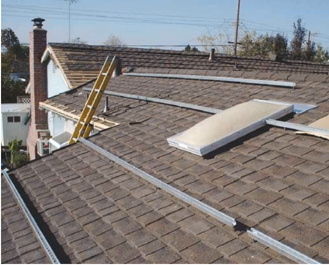
Unistrut rack material on top of the new metal shake roof.
