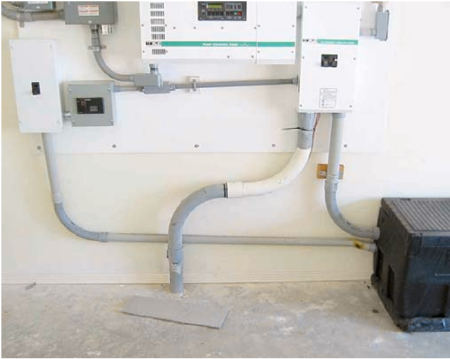
Good working clearances, with the equipment not mounted over the batteries.
