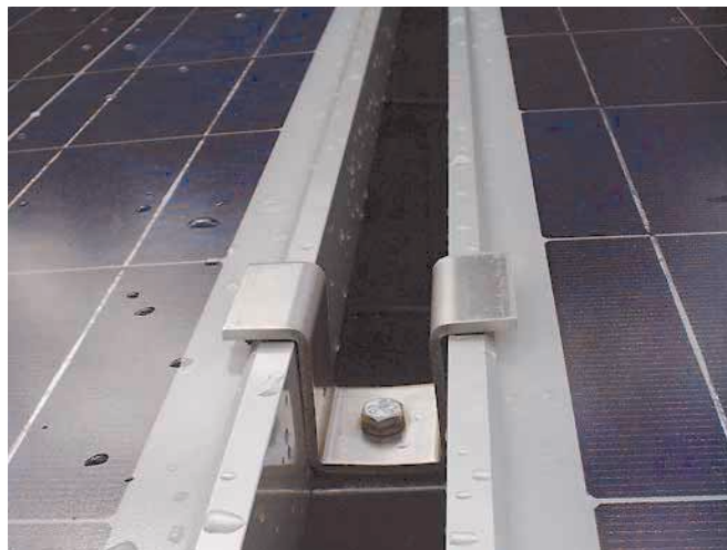
Custom U-brackets hold down adjacent panels.
