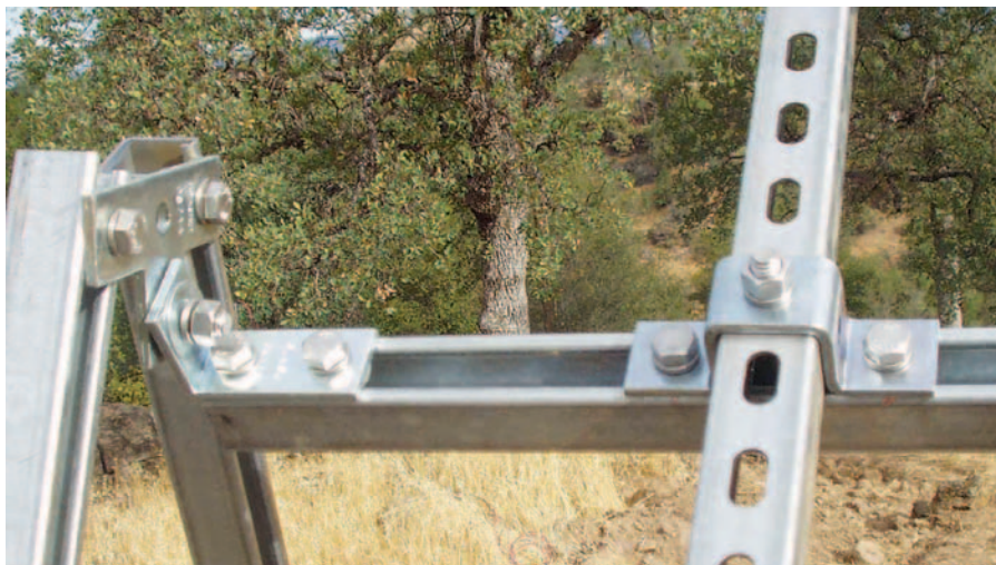
Pivot detail assembly: T-plate, pivot beam, corner angle, U-support, and fasteners.
