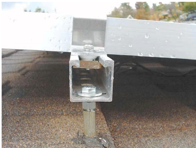
Hanger bolts, Unistrut rails, and custom-made brackets (Z-bracket shown) for securing the panels make up this mounting system.
