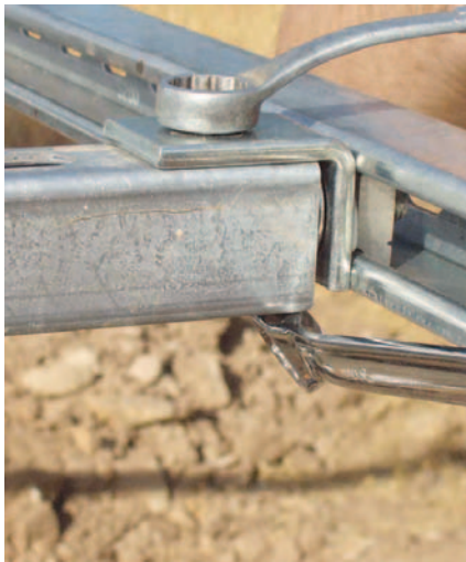
A top or bottom end is attached to a cross-arm with a two-hole corner angle and a channel nut.
