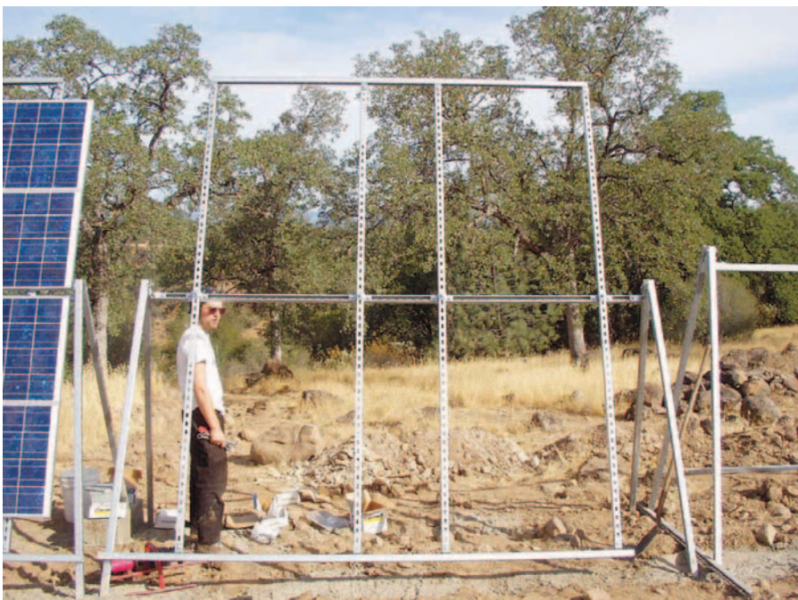
The rack framing and pivot arm assembly. The array will become plumb when the right arm extension is installed.
