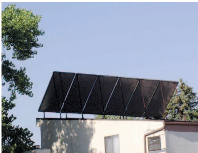
From the back of this drainback array of six, 4 by 8 foot collectors, the slight slope of the collectors can be seen.
