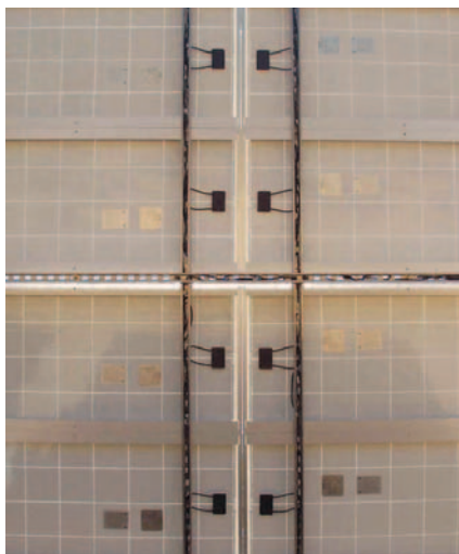
Finished—all the wiring is neatly tucked away in the PowerStrut and conduit.
