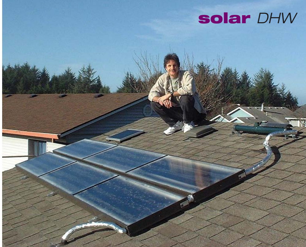
Solar installer Andrew Gerl of Blazing Solar of Mesa, Arizona, on the roof with solar thermal collectors, the PV module for the pump, and the TPFRS radiator/reservoir unit.
