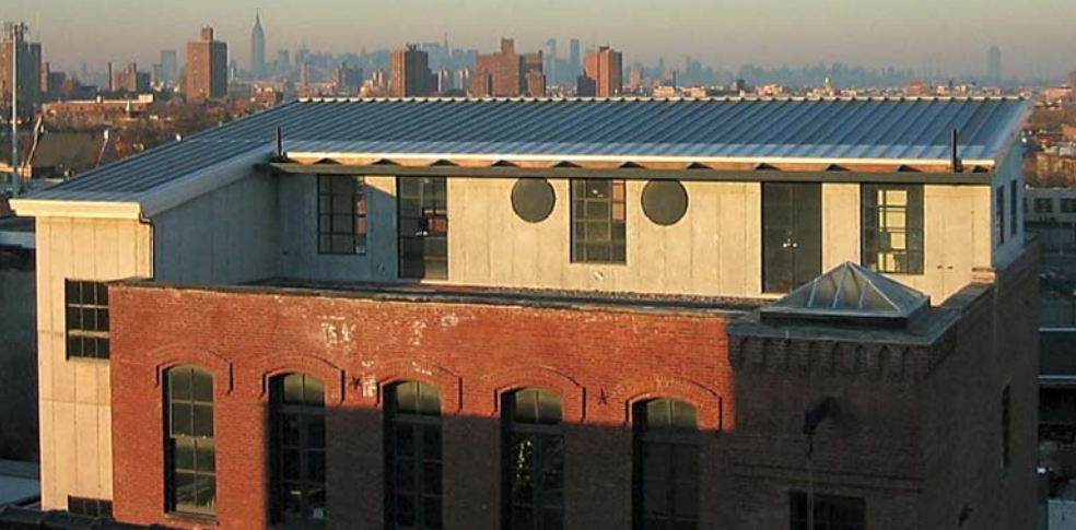
Seven kilowatts of Uni-Solar photovoltaic laminates cover almost the entire 1,200-square-foot area of the icehouse's rooftop addition.
