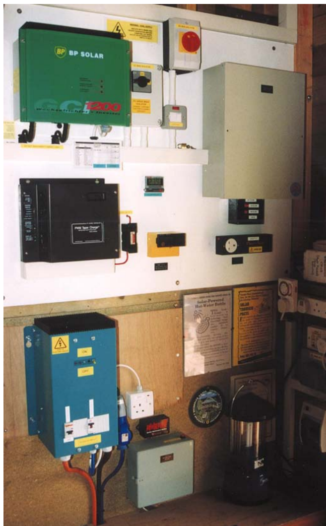
The grid-intertied BP inverter and related components, as well as the independent battery-based system, are housed inside the garden shed.
