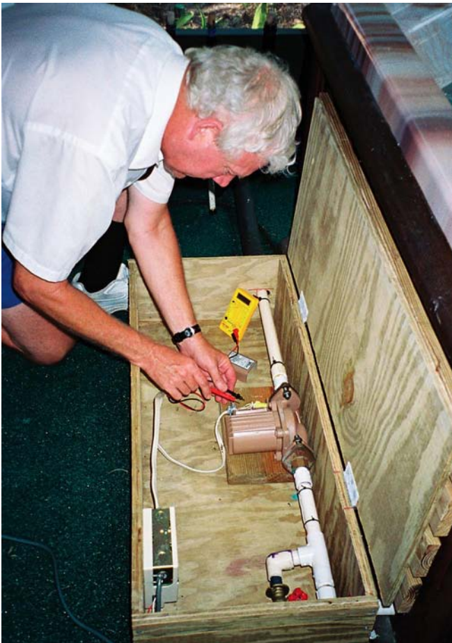
Bob uses a multimeter to test the voltage to the pump relay.
