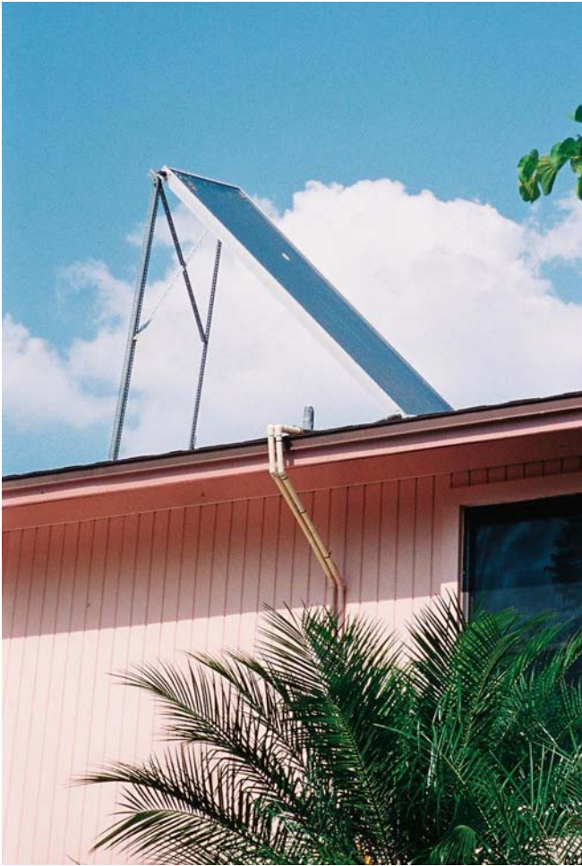
The Owens' roof-mounted, flat-plate solar collector. Note the piping detail that allows the water to flow easily.
