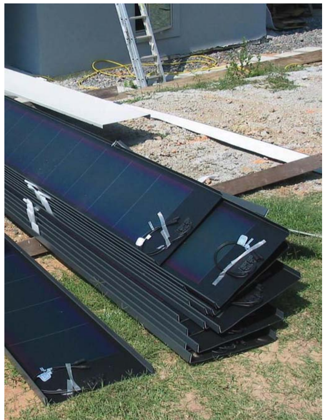
Assembled PV-laminated roof panels ready to go on the roof.
