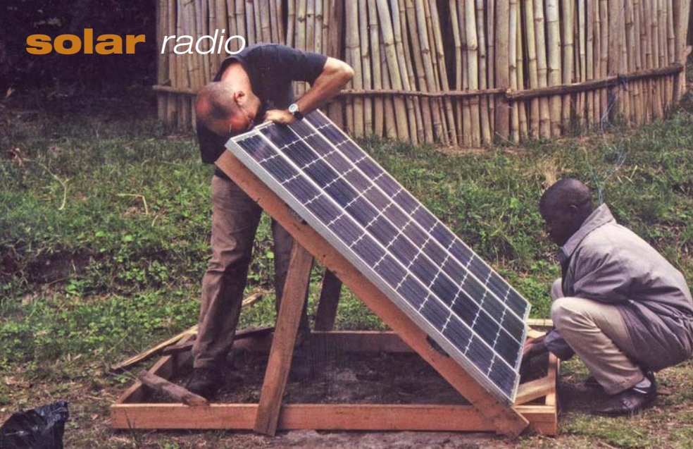
Martin Nsengumuremyi helps the author check that the array fits on the frame before everything is hauled up the mountain.
