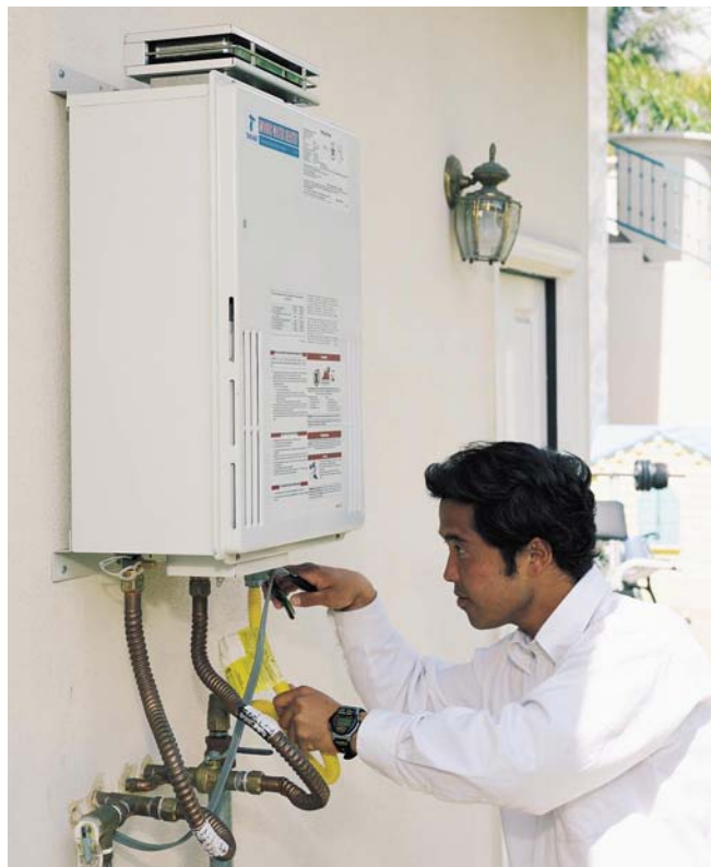
On-demand water heaters can be installed indoors, or outdoors where the average winter temperature stays above 5°F.
