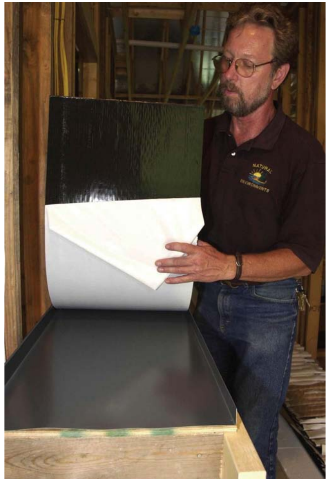
Peeling the backing from the end of a Uni-Solar laminate before adhering it to the metal roofing.
