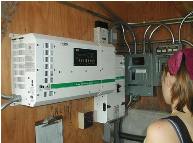
The balance of system components for a DC hydro system are very much like a photovoltaic system, except the charge controller shunts to a diversion load.
