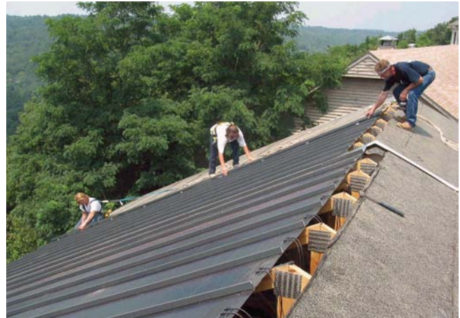
Installing the roof panels.
