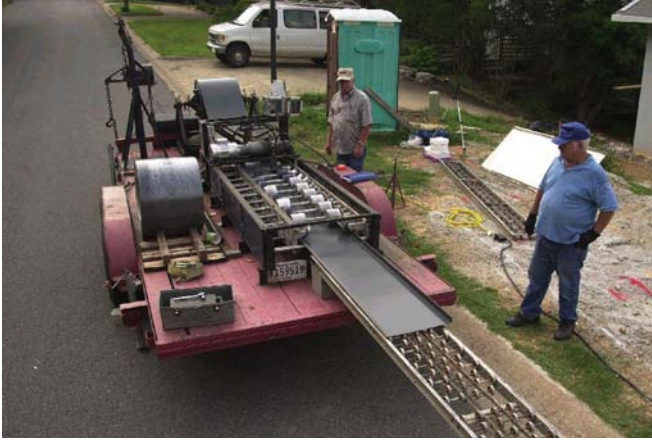
Making the roof panels on site.
