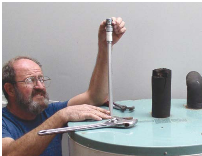
Installing a new rod in the tank.
