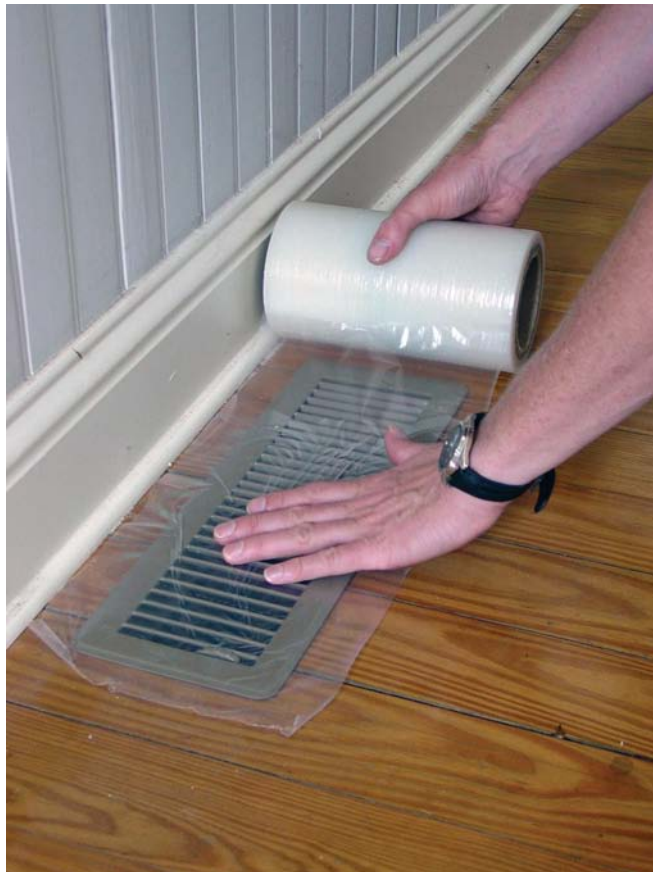
Sealing the registers in preparation for the duct pressure test.
