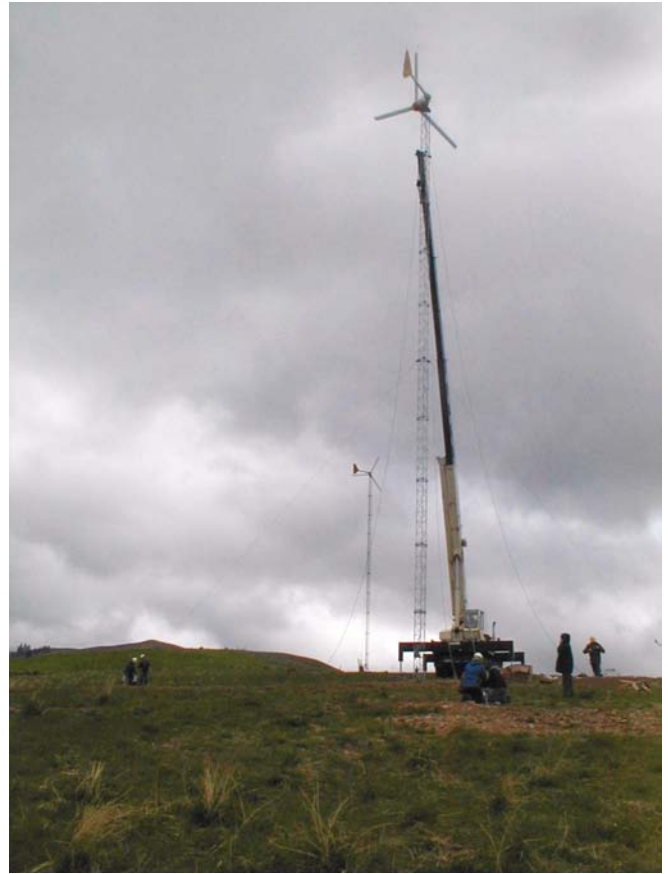
A crane lifts the second Bergey Excel wind turbine on a 100-foot (30 m), guyed, lattice tower.
