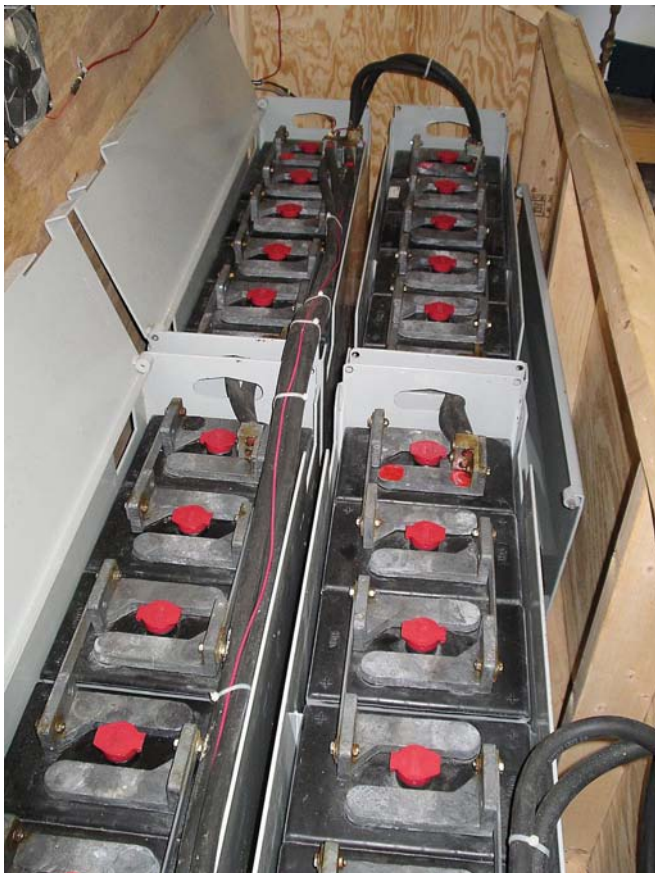
Left: Four large, industrial quality, deep-cycle batteries provide energy storage for the island home.
