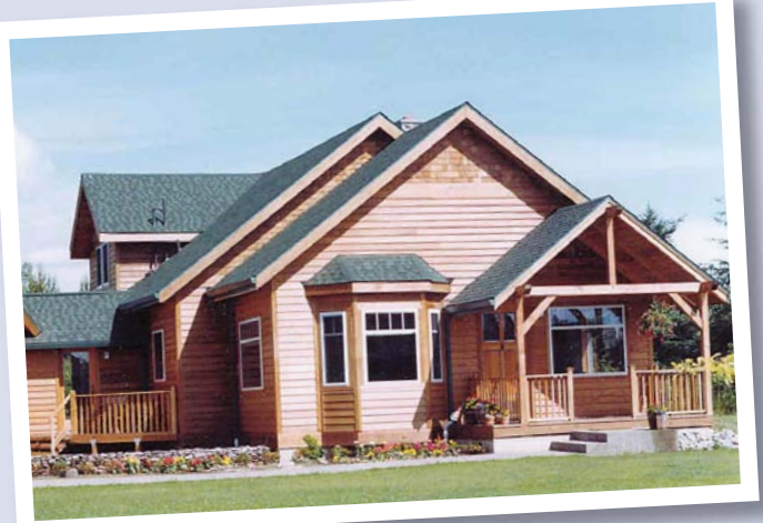
The Sughrue home in Vancouver, Washington, integrates SIPs and recycled timbers for energy and resource efficiency. Built in 1999, heating bills have averaged only US$350 per year.
