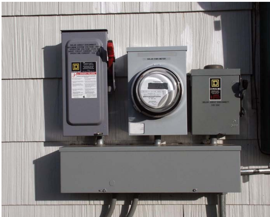
Solar array disconnect, system AC kilowatt-hour meter, and inverter disconnect mounted over a weatherproof wiring enclosure.
