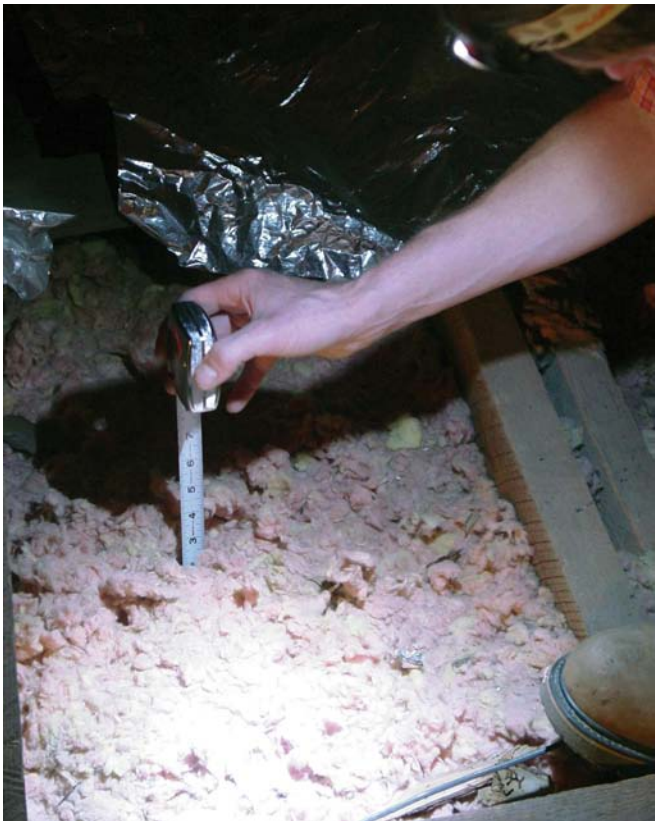
Checking the attic insulation levels.
