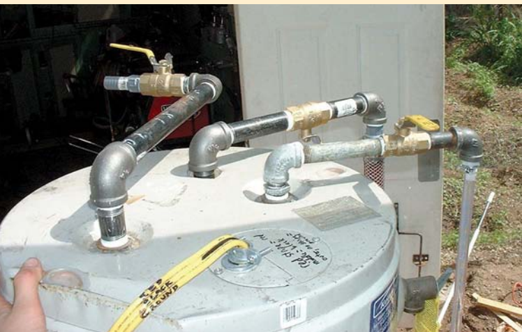
The vent assembly at the top of this tank is set up for methanol recovery using a condenser.
