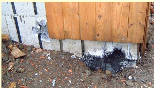
Attracted to the rebar in the building's foundation, the lightning induced surge traveled to and blew out the corner of this garage.
