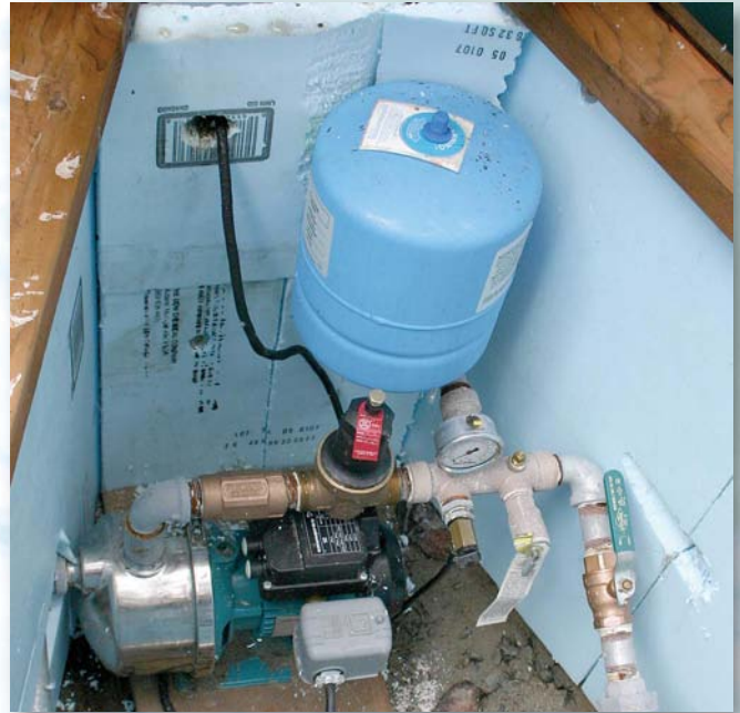
The basic components of a rainwater irrigation system, including pump and pressure tank, in an insulated box.
