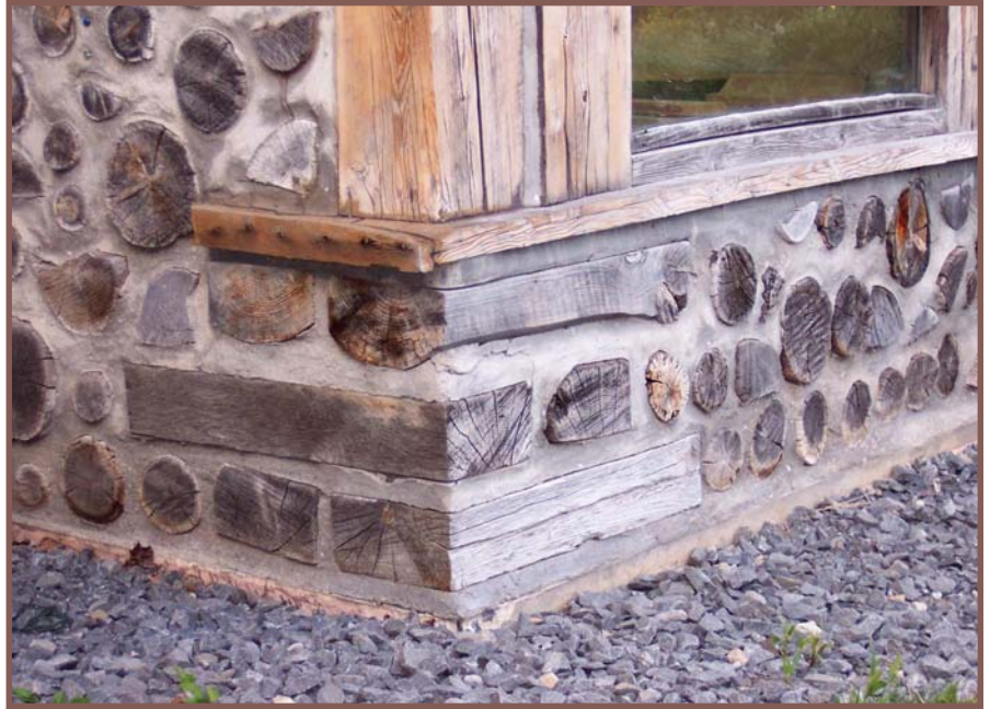
Stackwall corners consist of alternating corner pieces called quoins or Lomax corners.
