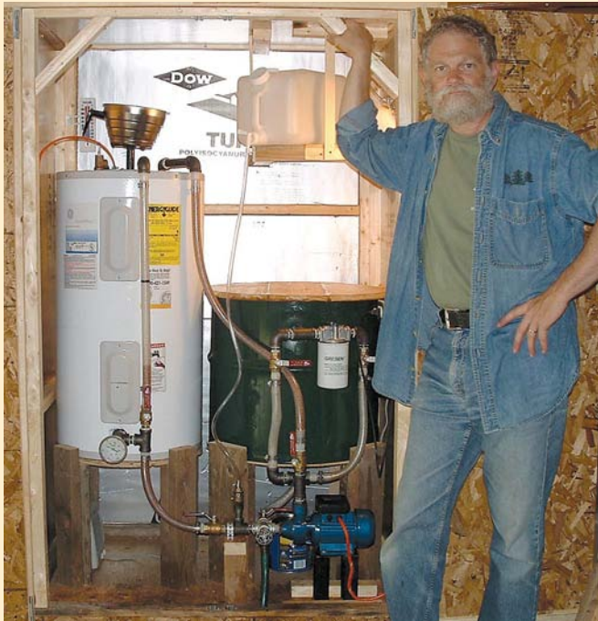
David Probert tucked his beautiful system into a cabinet, insulated for Maine winters. In this small system, based on a 19-gallon, mobile-home water heater, several parts perform more than one job.
