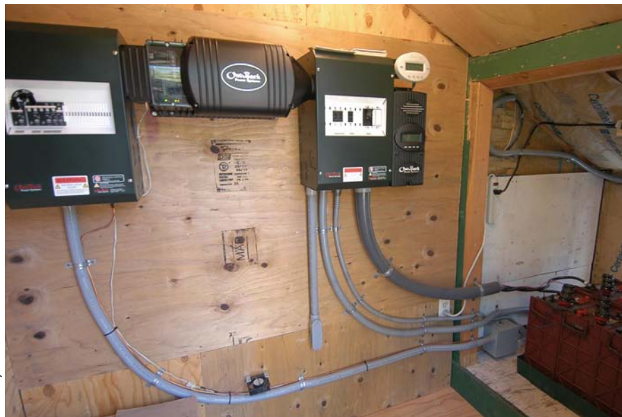
The PV power shed houses an OutBack inverter, charge controller, AC and DC disconnect panels, and the battery bank.
