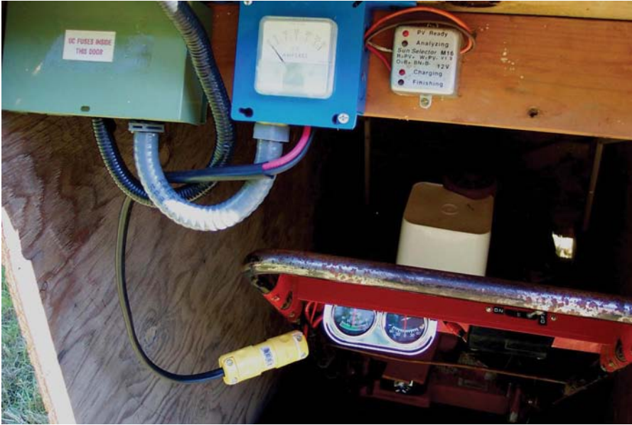
PV charging system the in shed: fuse box, ammeter, charge controller, charging cord, and mower.
