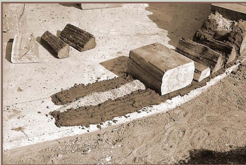
The first course of wood laid on top of the first layer of mortar.
