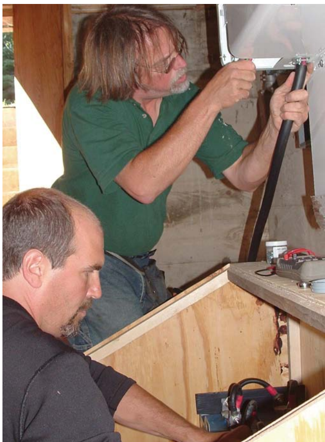
Daryl DeJoy (left) wires the battery bank while Stu Hall runs cable to the system's inverter.
