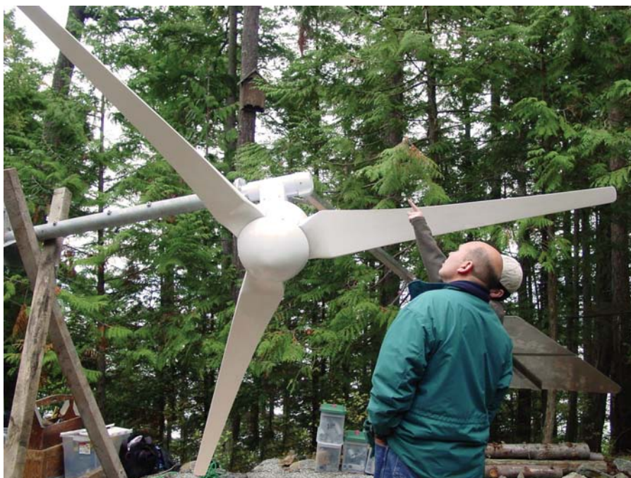
The complete AWP wind turbine was bolted to the tower’s top section prior to lift.
