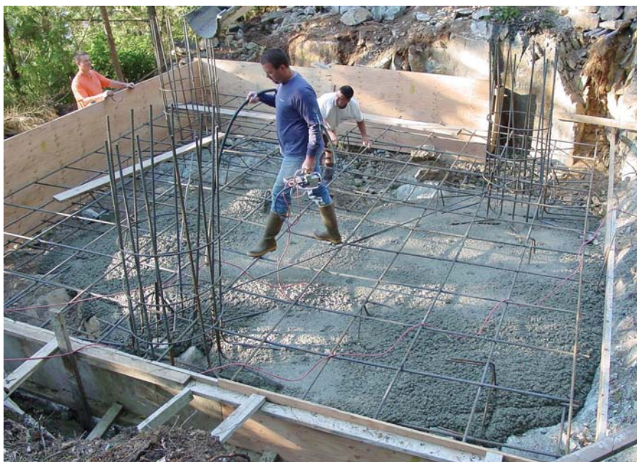
Reinforcing steel and bolts were set into the foundation before pouring concrete.
