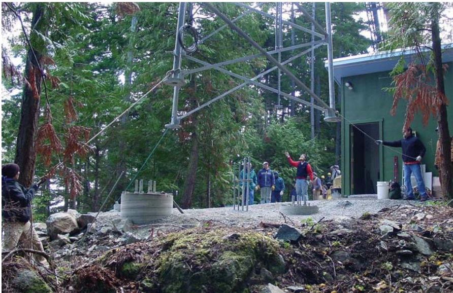
A 50-ton crane lifted each assembled tower section into place. Amazingly enough, the first section lined up perfectly with the column bolts set into the concrete.
