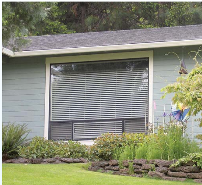
During the day, interior blinds block the sun. At night, operable windows can be opened to admit cool air.
