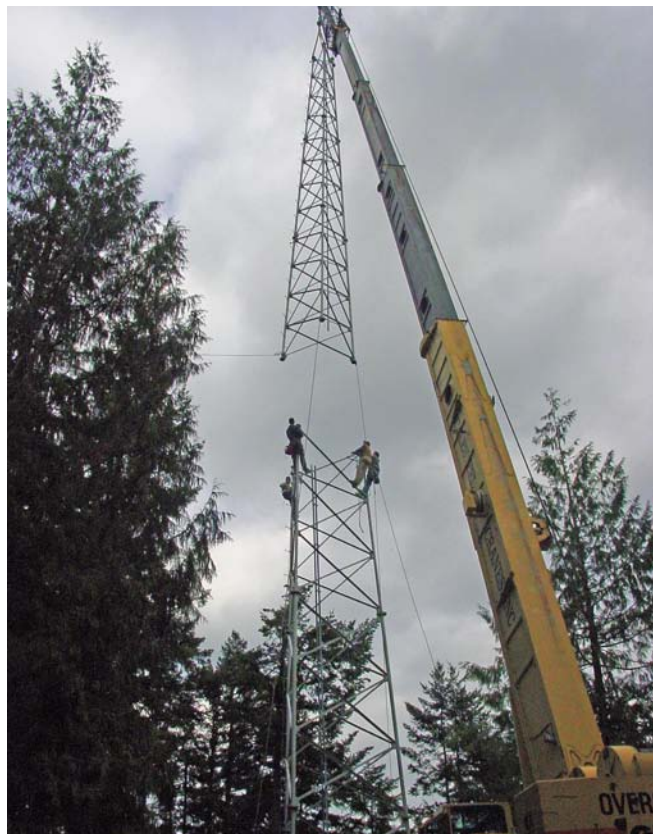
The crew at the top of the tower's first section gets ready to receive and bolt the second section into place.
