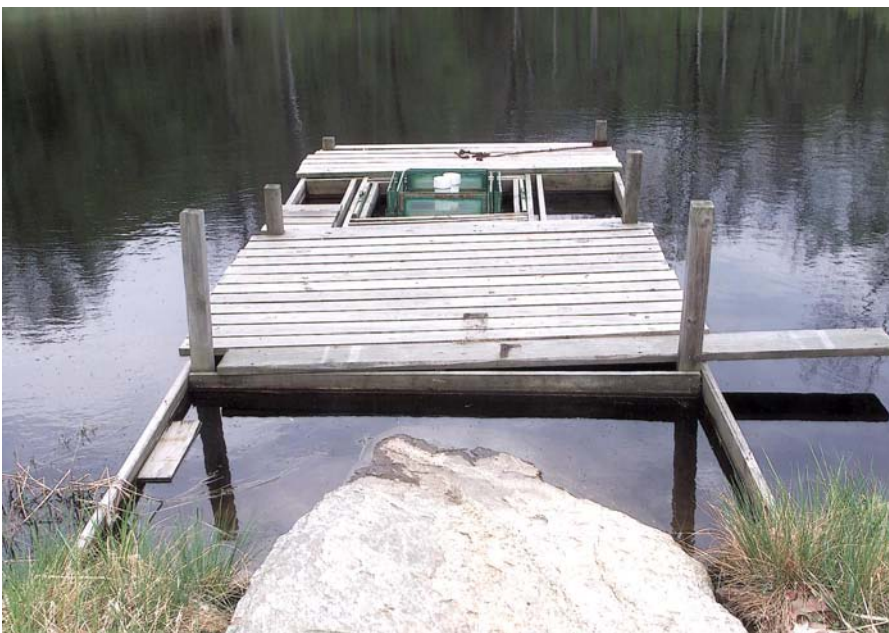
The intake pipe is secured to the bottom half of a new septic tank hidden beneath the dock.
