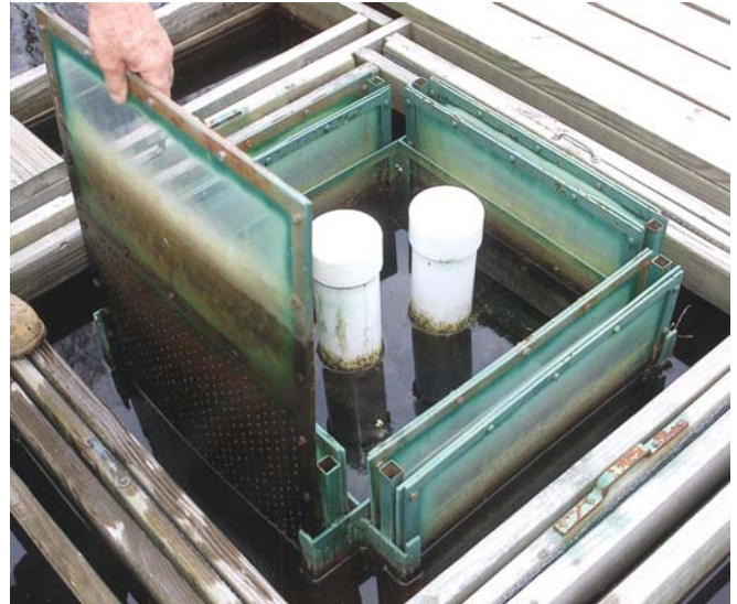
The removable intake screens are easy to clean.
