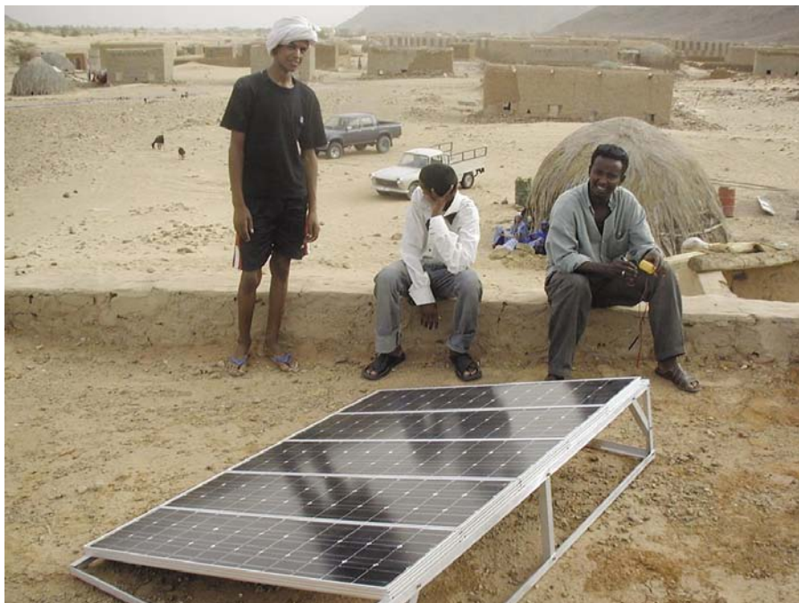
The villagers look at the completed PV array on the roof of the chief's house. The rack was later weighted down with rocks and sandbags to keep it secured.
