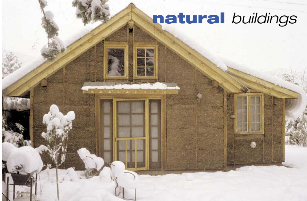
Straw light-clay provides about the same insulation value per inch of thickness as straw bale, and is compatible with conventional stud framing. This straw-clay house was built by Robert Laporte of EcoNest, and is awaiting exterior plaster.
