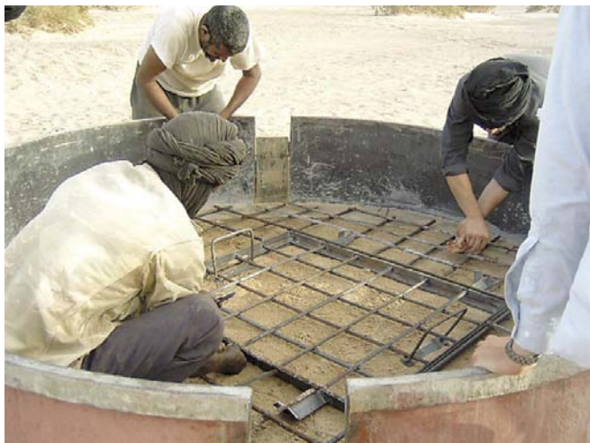
Setting the rebar for the poured concrete well cap.
