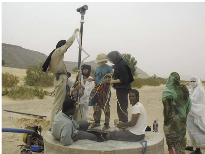
Lowering the submersible pump and sand trap assembly into the well.
