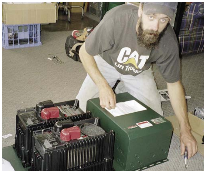
Installer Ben Scurfield assembles the OutBack PS2 power panel. The second inverter case is for display only.
