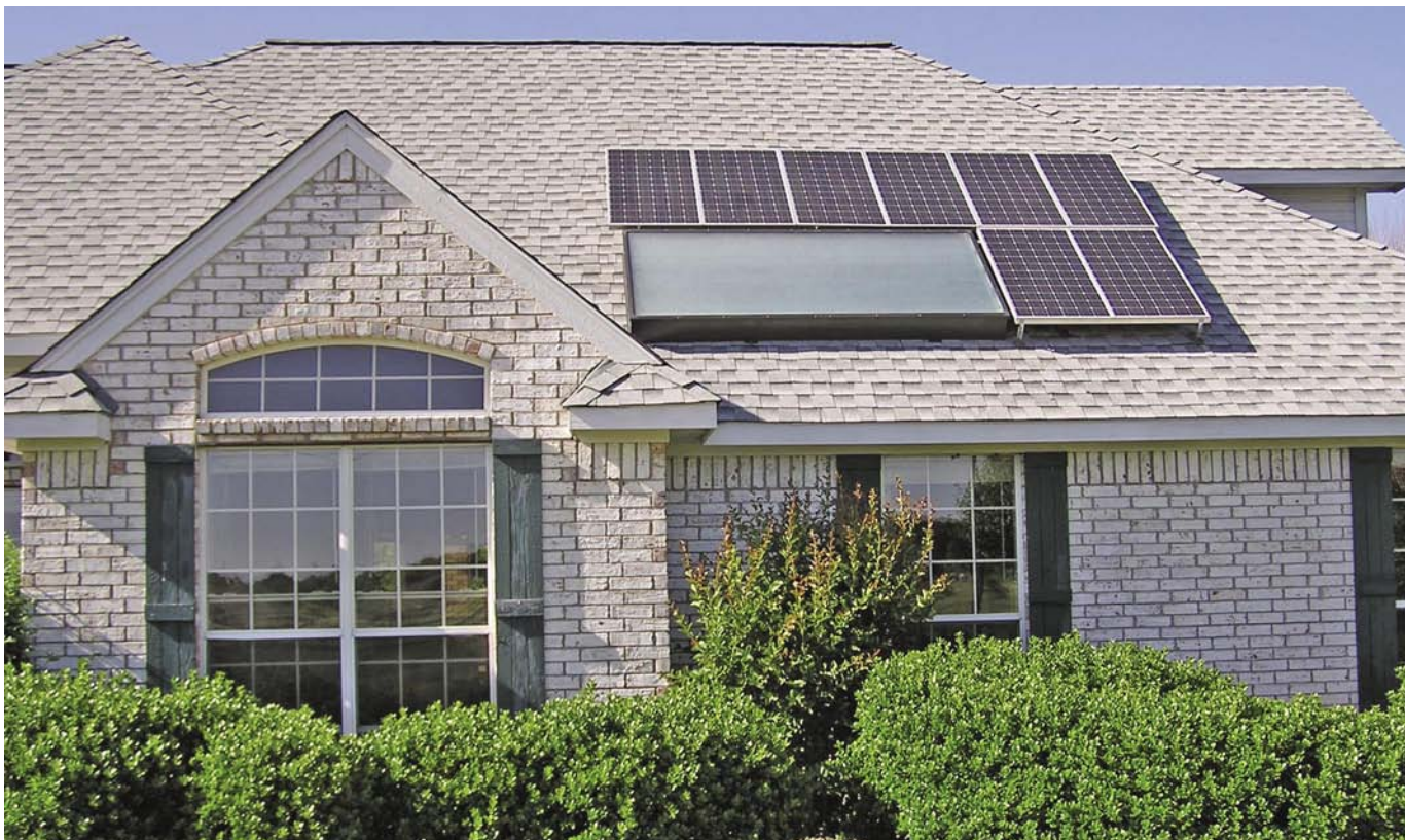
A batch water heater mounted on the garage roof (alongside the solar-electric array) meets a large portion of the Geisler family's hot water needs. The 880-watt, utility-intertied array offsets electrical use by about 15 percent.
