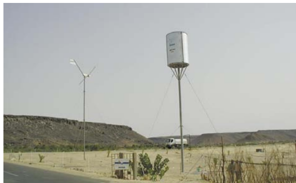
A French wind-electric water pumping system in a neighboring village. The wind resource was strong enough that we never saw this turbine stopped while we were there. The water is pumped to the storage cistern on the pole, and then used to fill up tanker trucks that deliver it.
