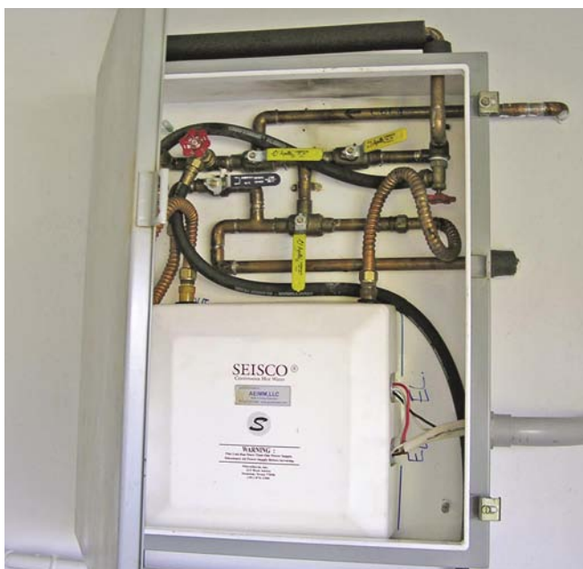
An energy saving, on-demand, tankless water heater serves as a good backup to a solar domestic hot water system.
