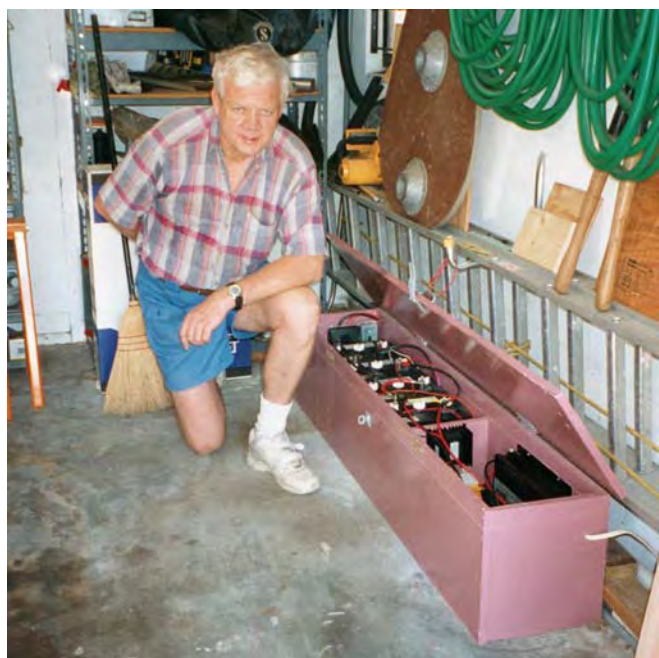
The author with his batteries and inverter.
