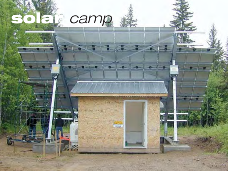
Rear view of the array and electrical building. This building contains the batteries, inverters, back-up generator, and charge controllers.
