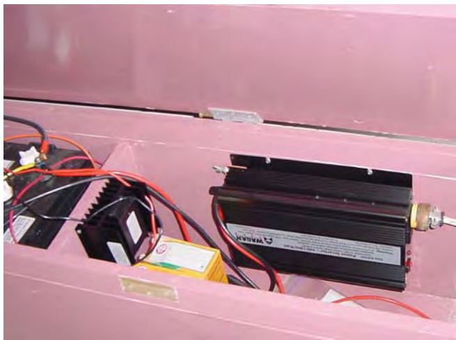
The battery box stores the batteries, PWM charge controller, and inverter. A divider separates the batteries from the electronics.
