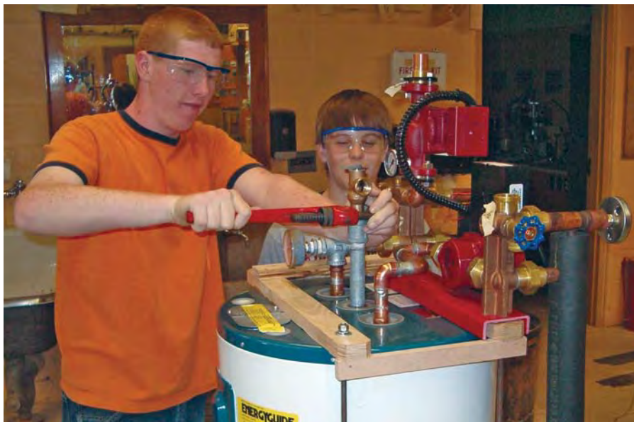
Chad is learning to judge how tight pipe fittings must be while keeping in mind the alignment to other fittings, like elbows and tees.
