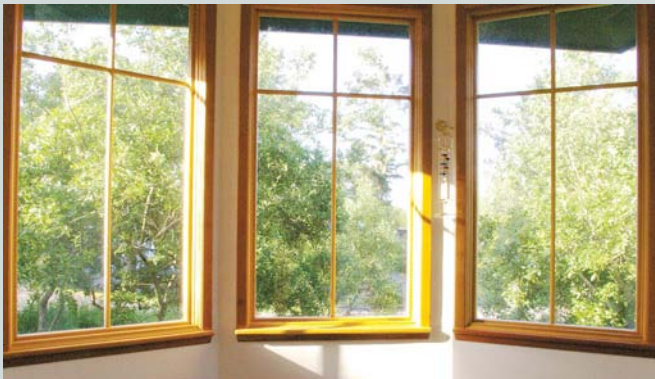
South-facing, single-pane windows in the sunspace let in lots of sunshine for natural lighting and passive solar heating.
