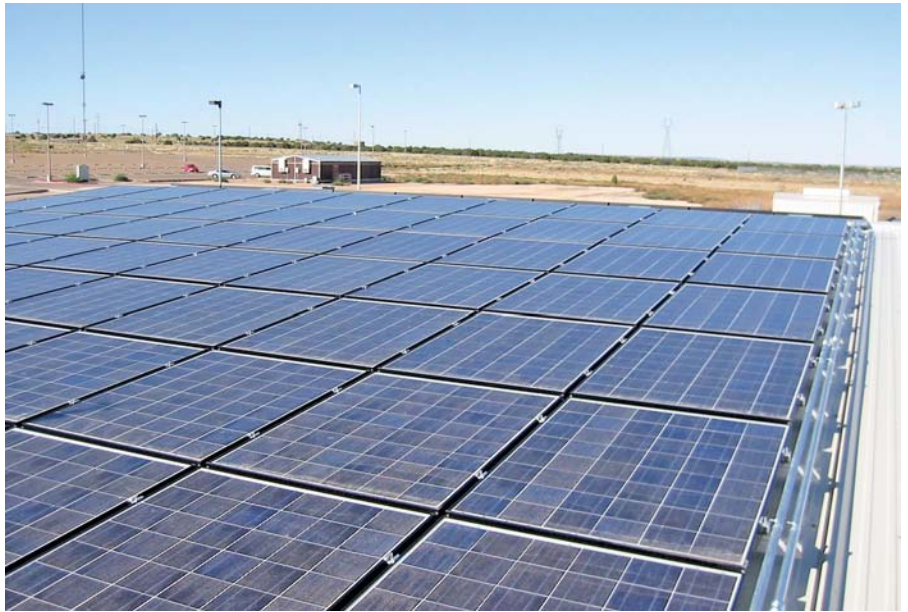
This 30 KW PV system requires a supply-side utility connection.
