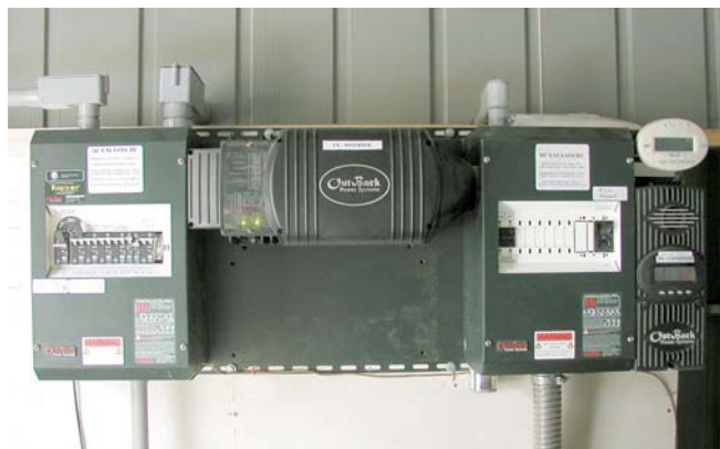
The OutBack Power Systems inverter, charge controller, system monitor, and AC and DC breaker panels.
