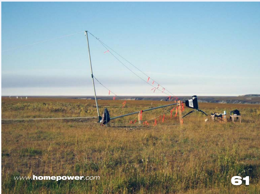
The 155-pound Proven wind turbine and its 20-foot tower were raised into place with a rope-and-pulley system.
