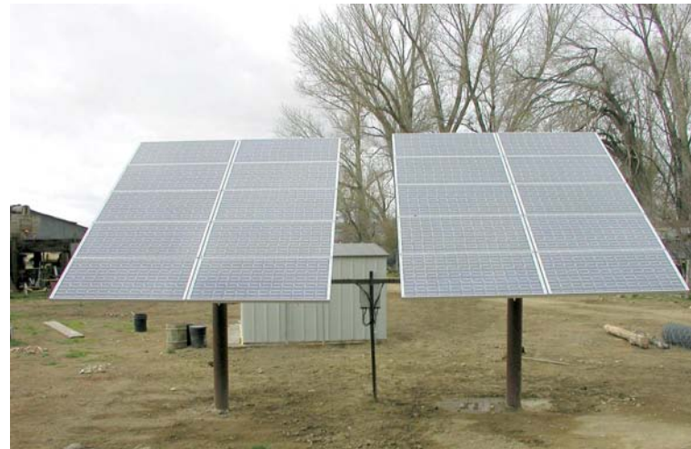
Two kilowatts of photovoltaic panels and some load efficiency measures significantly reduce the need for the diesel generator.
