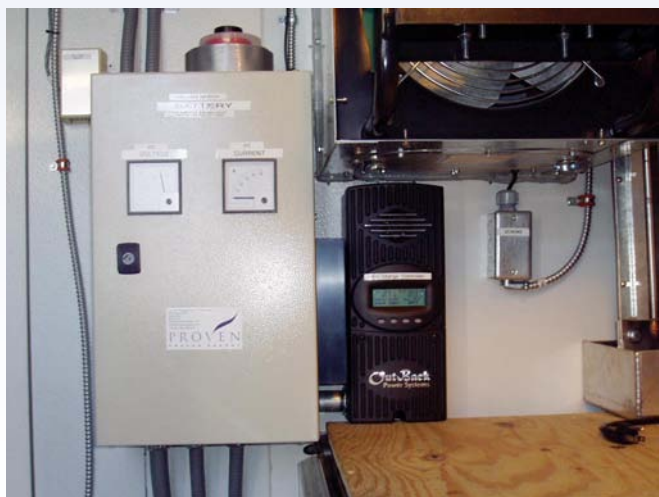
The Proven and the OutBack controllers regulate wind and PV charging.
