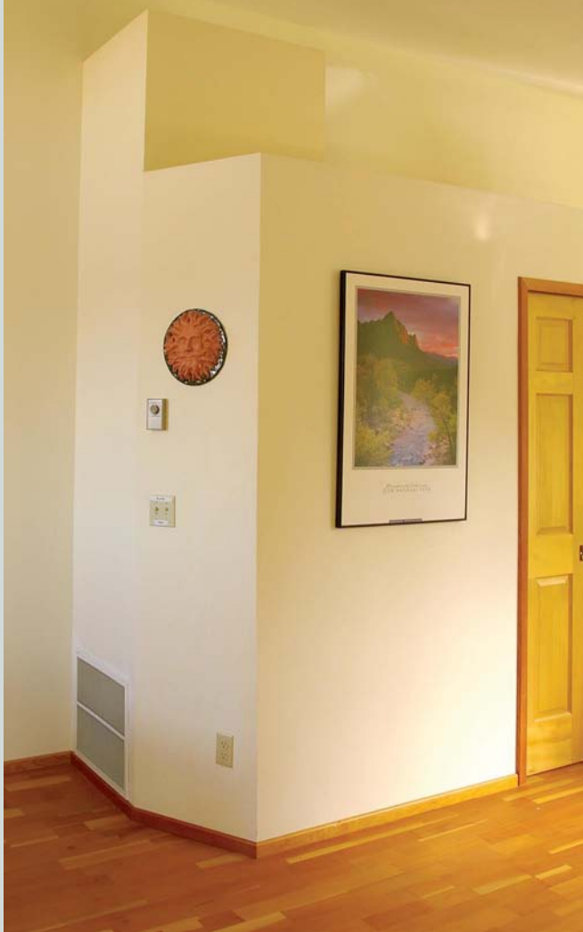
Solar-heated water cycles through fan coils inside this built-in enclosure. Air enters from the top right and exits lower left.
