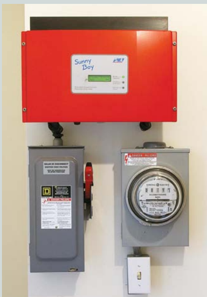
Left: The SMA Sunny Boy utility-interactive inverter, PV disconnect, and dedicated PV KWH meter are located inside the house.
