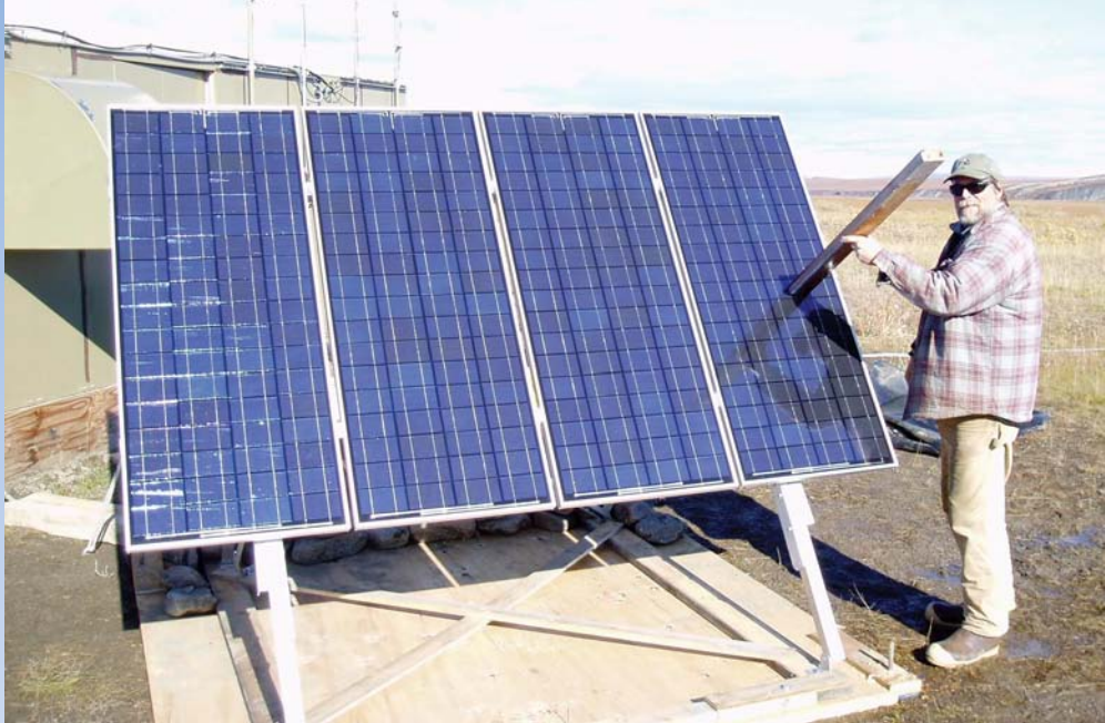
The author demonstrates that the PV tilt angle is to spec.
