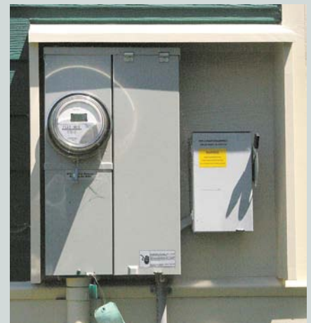
Right: The service entrance, utility lockable disconnect, and utility KWH meter are mounted outside.
