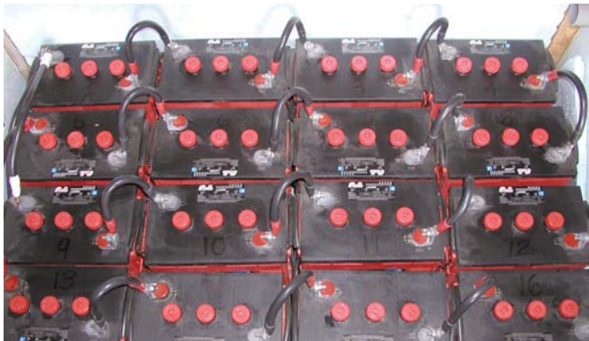
Sixteen Surrette S-460 batteries store solar energy for silent nighttime power.
