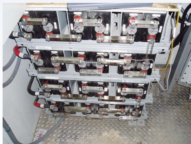
The battery bank is made up of 24 industrial-quality, 2-volt cells.
